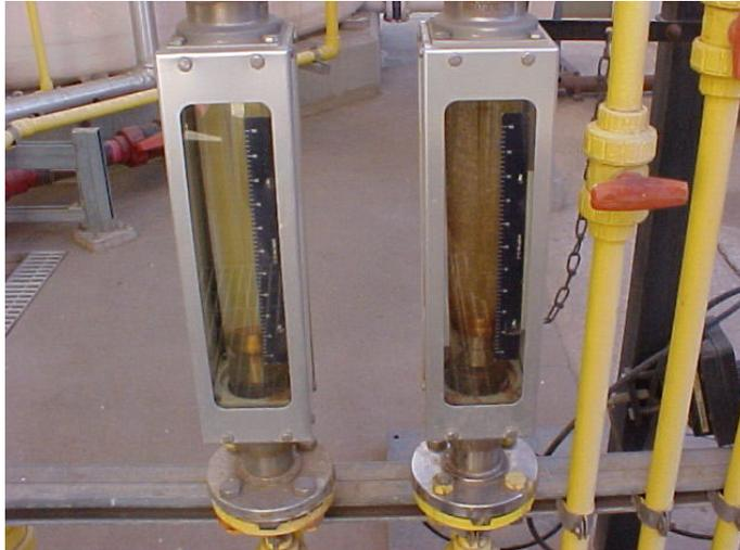
Various Chlorine measurement devices or Rotometers.
