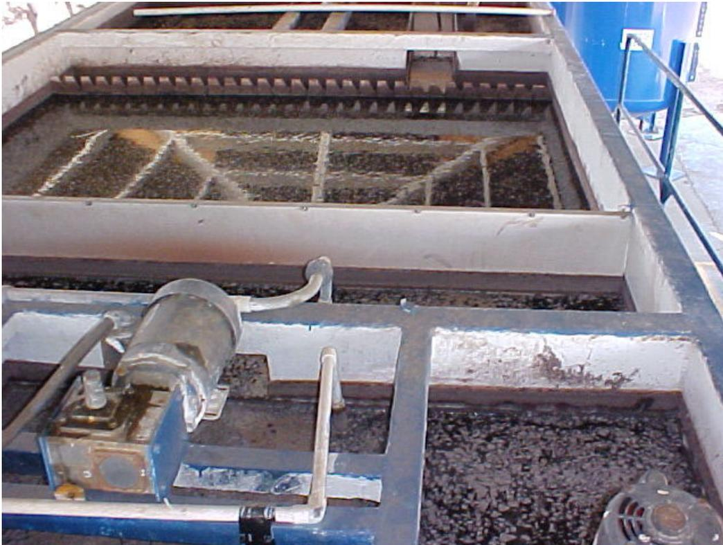
Example of a small water treatment package plant with coagulation, flocculation and filtration all within a 20-foot area.
