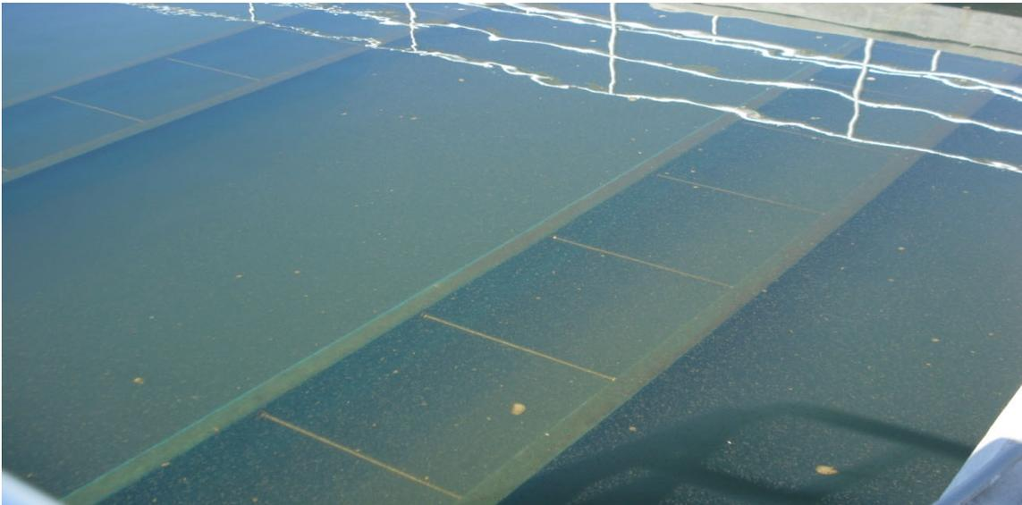
The above photograph is a filter from a direct filtration plant; notice the size of the floc – a good size for filtration.
