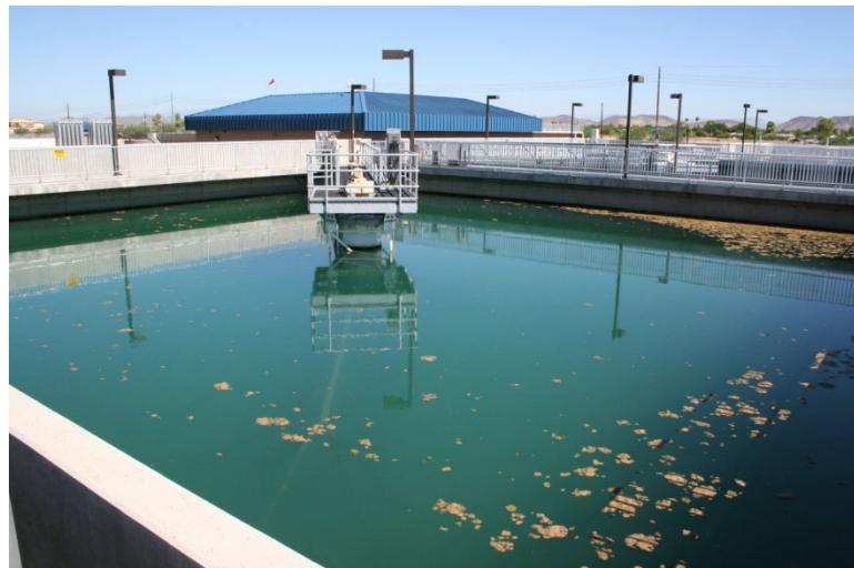
Let's first look at the components of a rectangular clarifier. Most are designed with scrapers on the bottom to move the settled sludge to one or more hoppers at the end of the tank. It could have a screw conveyor or traveling bridge used to collect the sludge. The most common is a chain and flight collector. Most designs will have baffles to prevent short circuiting and scum from entering the effluent.
