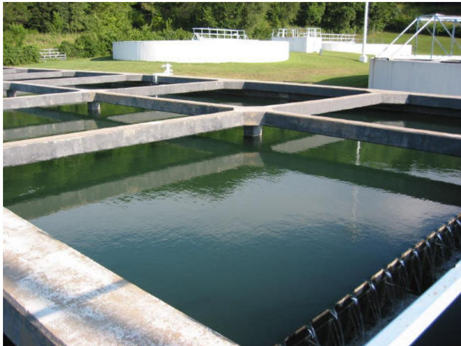
Top Photograph - Final Rectangular Sedimentation Basin Discharge Weirs
