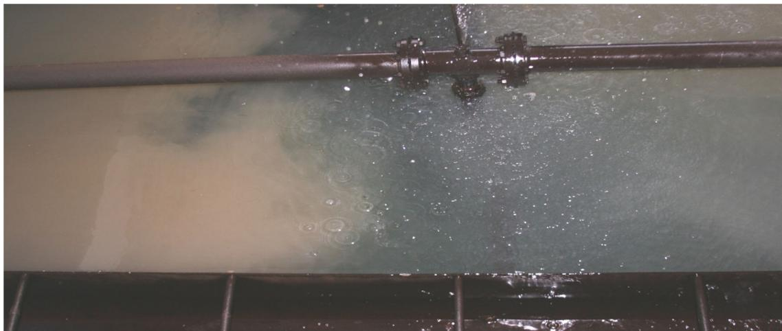
The surface wash system consists of a series of pipes installed in the filter that introduce high velocity water or air jet action into the upper layer of the filter. This jet action will generally be supplied by rotating arms that are activated during the backwashing of the filter.
