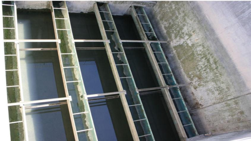
In this photograph, you can see the water lines on the wall of the filter. The deeper the water the more head pressure exerted on the filter media.
