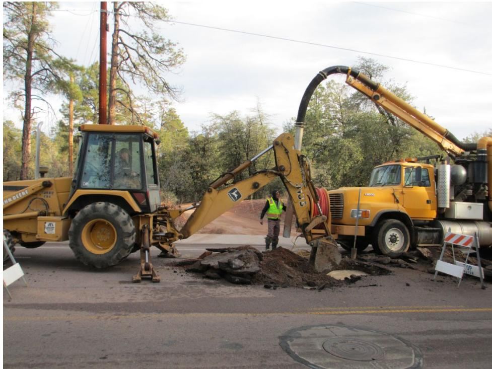
In this case, a sewer vecto was utilized to expedite removal of water and spoil. Utilizing a vecto is a great tool, but is dangerous. It is easy to lose tools and injure personnel if the vecto is not properly managed. The vecto is powerful enough to lift large stones and even a 200 pound man.
