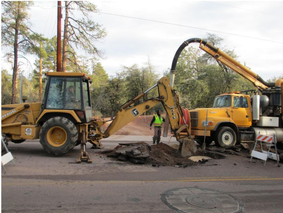
In this case, a sewer vector was utilized to expedite removal of water and spoil. Utilizing a vector is a great tool, but is dangerous. It is easy to lose tools and injure personnel if the vector is not properly managed. The vector is powerful enough to lift large stones and even a 200 pound man.
