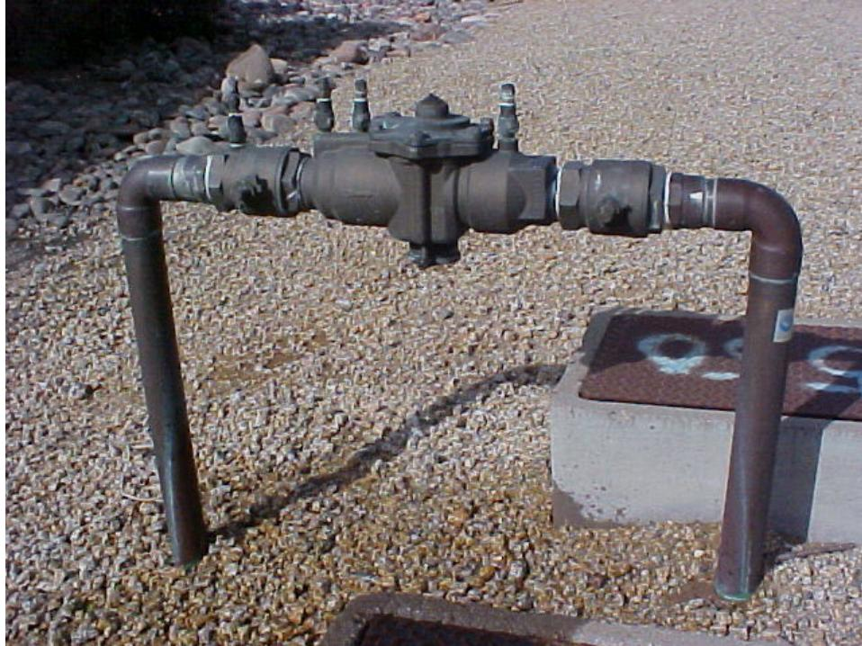
Leaky RP--have your assemblies tested annually or more often. Re-test after repairs and problems. A RP should not leak more than 1 or 2 minutes any more than that, there is a problem, a piece of debris or a stuck check is causing this RP's hydraulic relief port to dump.
