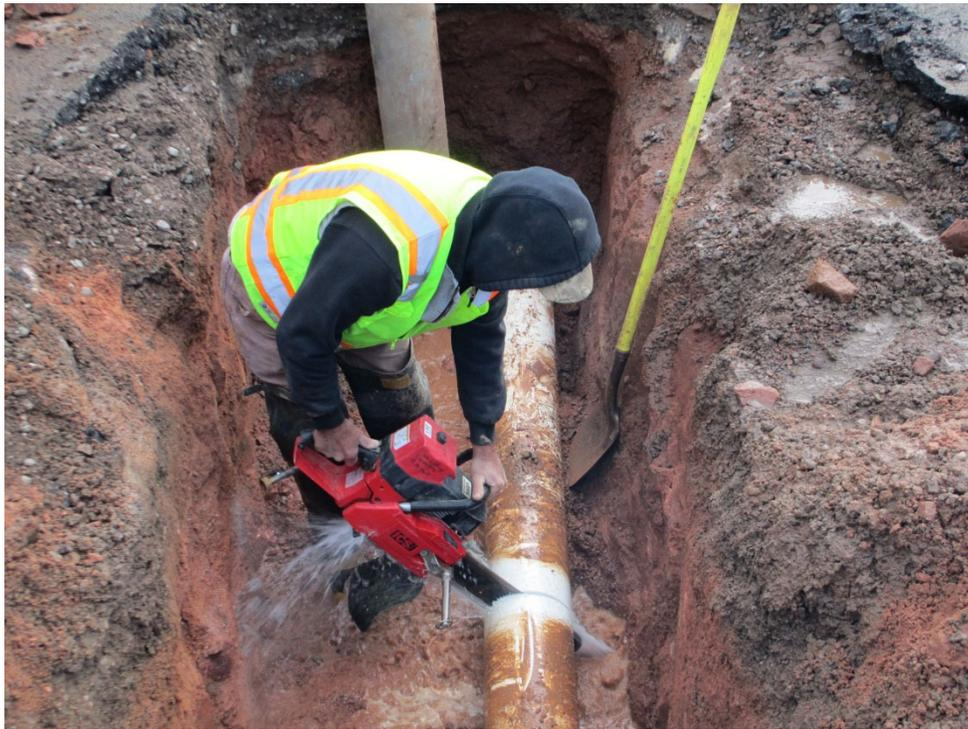
Any work with a chainsaw or powersaw should include proper safety equipment including proper eye protection, face shield, and hearing protection. The blue pipe is an eight inch plastic C900 and will be utilized for the repair.
