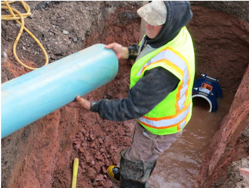
You will notice the blue Hymax coupling is being utilized instead of a clamp or flex coupling. This coupling is easy to use and has only two bolts and a special two-part gasket for odd size pipe.
