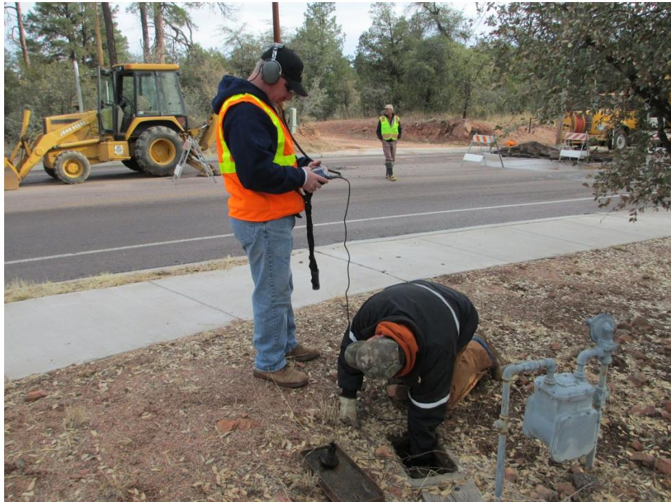
These men are listing to a stop to find a difficult leak. Some hydrophones magnify the sound and others use a meter to locate the leak. Many old-timers use a short piece of copper tubing and have good results.
