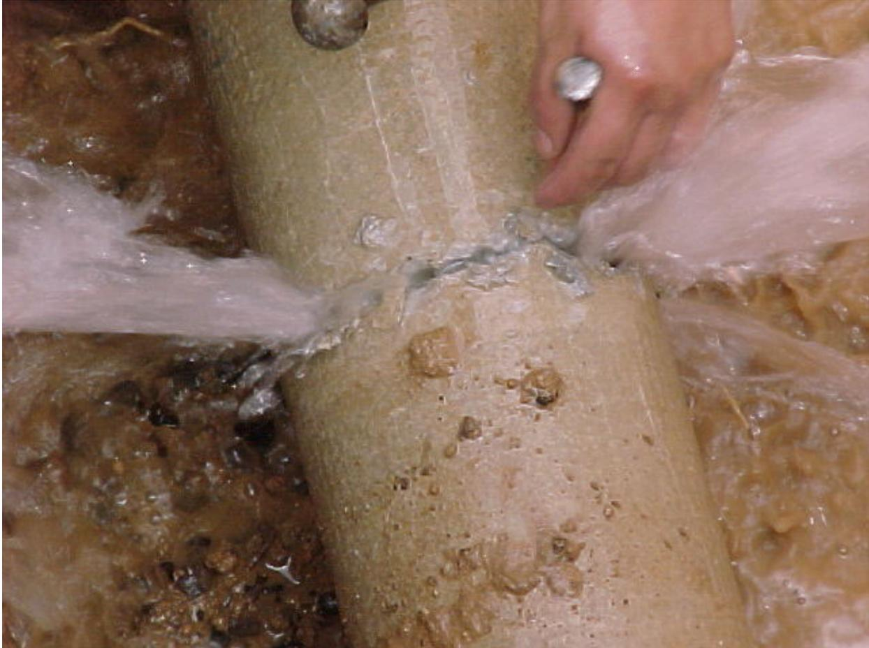
Using a chisel and keeping the ACP wet in order to cut the pipe, if possible Duct tape the pipe before cutting it.
