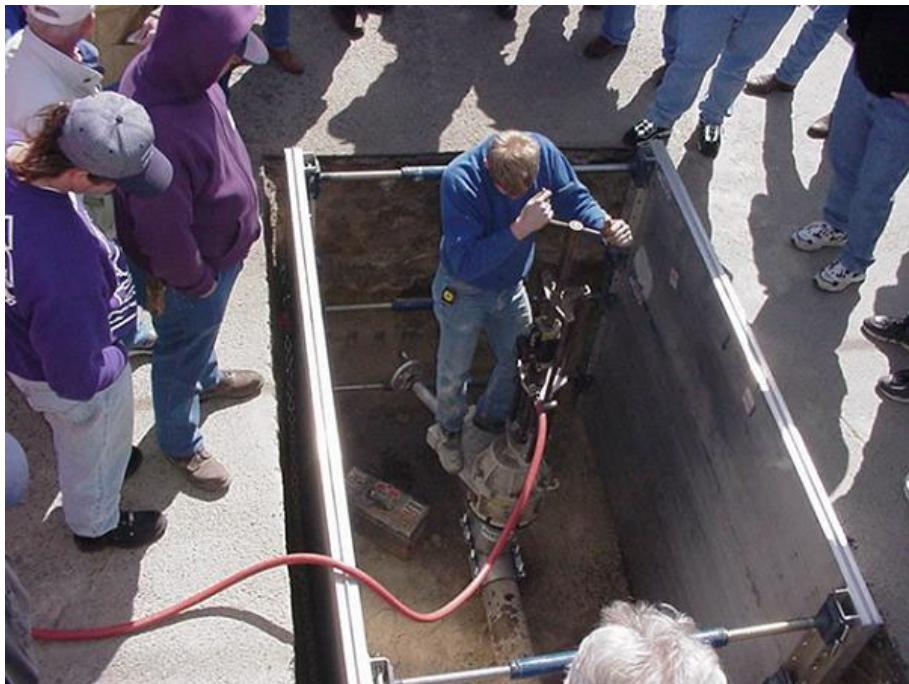
Hydro-Stop valve insertion machine
