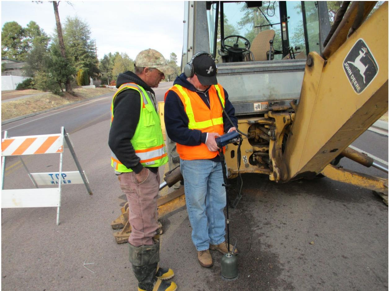
In this photograph, we see two men checking the results of a hydrophone. In areas of thick blacktop, it is difficult to locate small service leaks and slow water main breaks. A hydrophone is a microphone designed to be used underwater for recording or listening to underwater sound.
