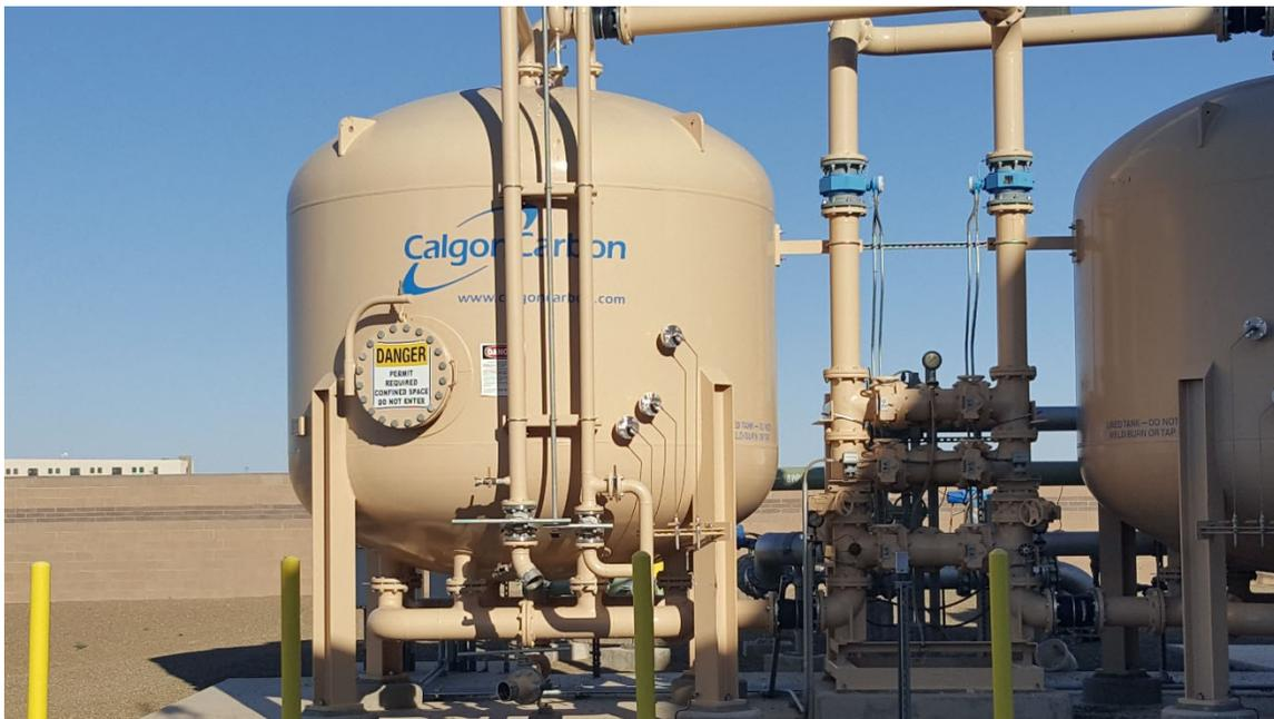
Granular Activated Carbon (GAC) vessel
