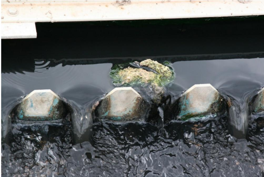
Caked grease (scum) stuck on a primary clarifier weir. Scum is normally scraped off and not sent to the downstream aeration tank.
