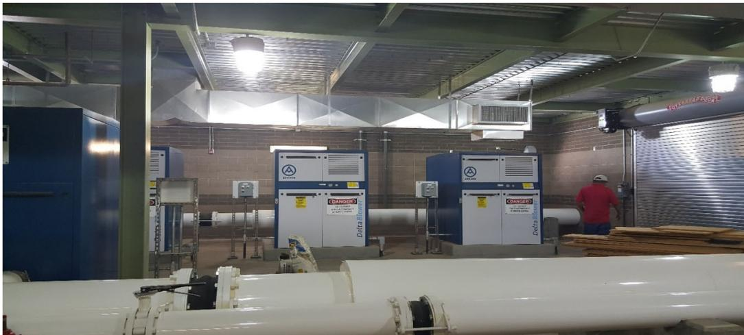
The above photo shows pipes and enclosed blowers as part of the aeration system. These areas are generally underground or in large buildings.
