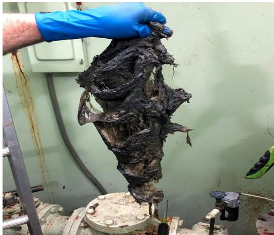
**Debris Removal:** An operator pulled wipes from the headworks that should not be flushed and clearly clogs equipment.
