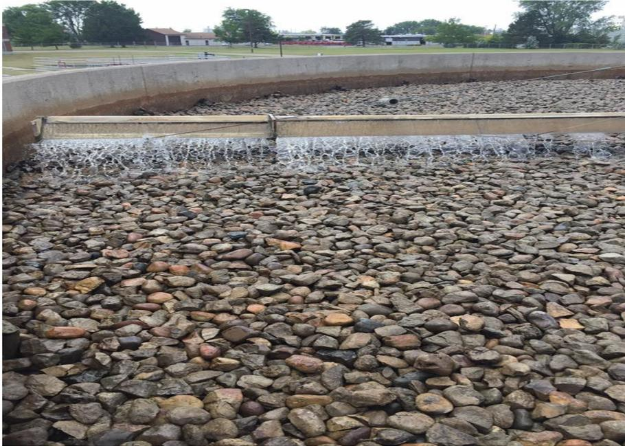
A TF consists of permeable medium made of a bed of rock (As seen above), slag, or plastic over which wastewater is distributed through the armature to trickle.
