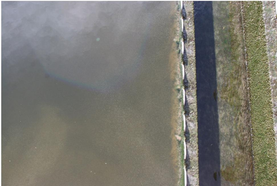
**Pin floc** being carried over the secondary clarifier weir due to a process upset. Ideally, the secondary effluent will be very clear. Excessive algae growth will create several different problems.
