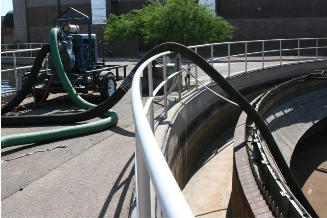
This circular clarifier has been dewatered with a portable pump
