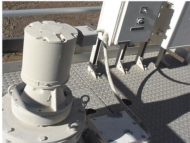
For the motor on this fixed bridge, aeration motor speeds are usually in the 1,800 rpm range. This speed is reduced to the 30 to 70 rpm range with gear reducers.
