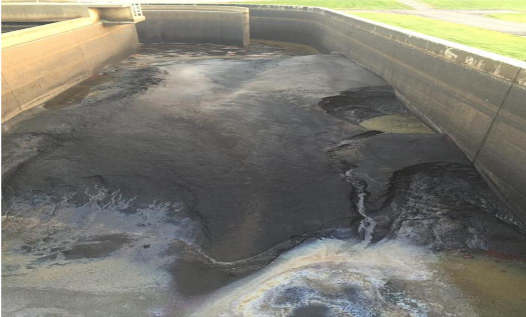
The results of not having grit removal. Filling part of an oxidation ditch aeration tank.
