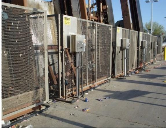
**Mechanical Bar Screens:** Operators should pick up trash that has blown off the automatic rakes.
