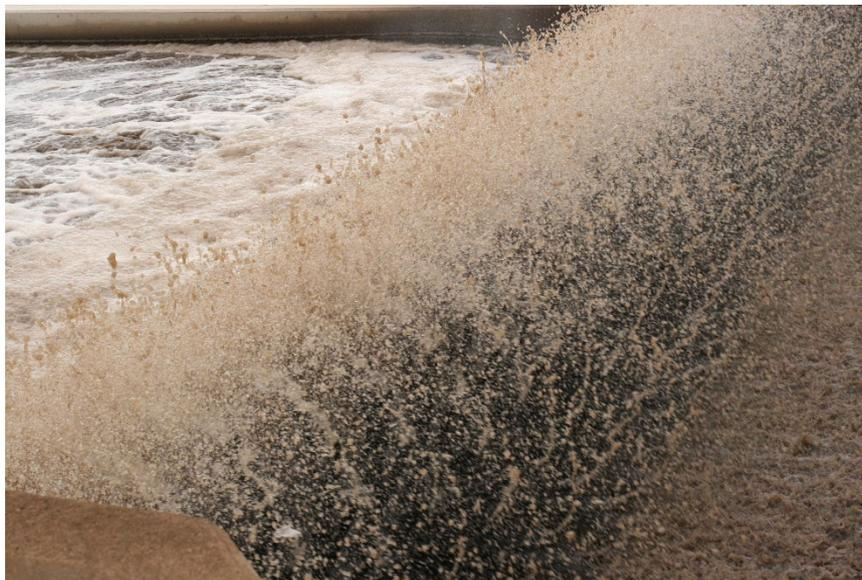
The rotor used above is for increase oxygen and mixing in an oxidation ditch.
