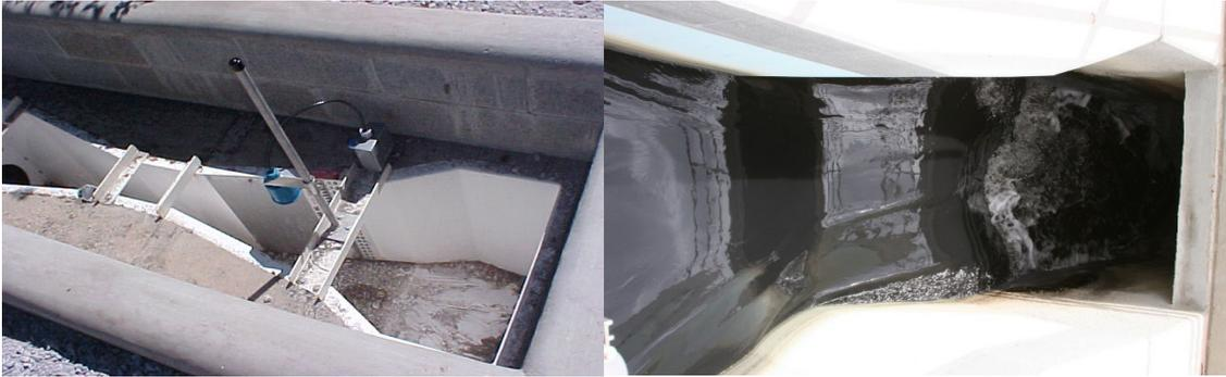
Sonic head (level) detection in the flume is used for flow measurement. Flow rates can be and used for flow weighted composite samples. Another application using sonic head level detection are weir boxes. Often referred to as a splitter box as illustrated below.
