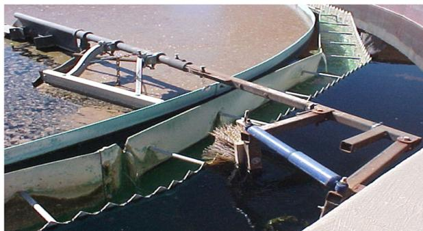
Typical scum removal equipment on the weir. Another important part of the secondary clarifier is the effluent weir, launder and pipe.
