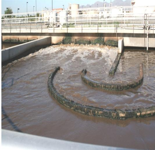
Oxidation ditch baffles slowing down the flow.
