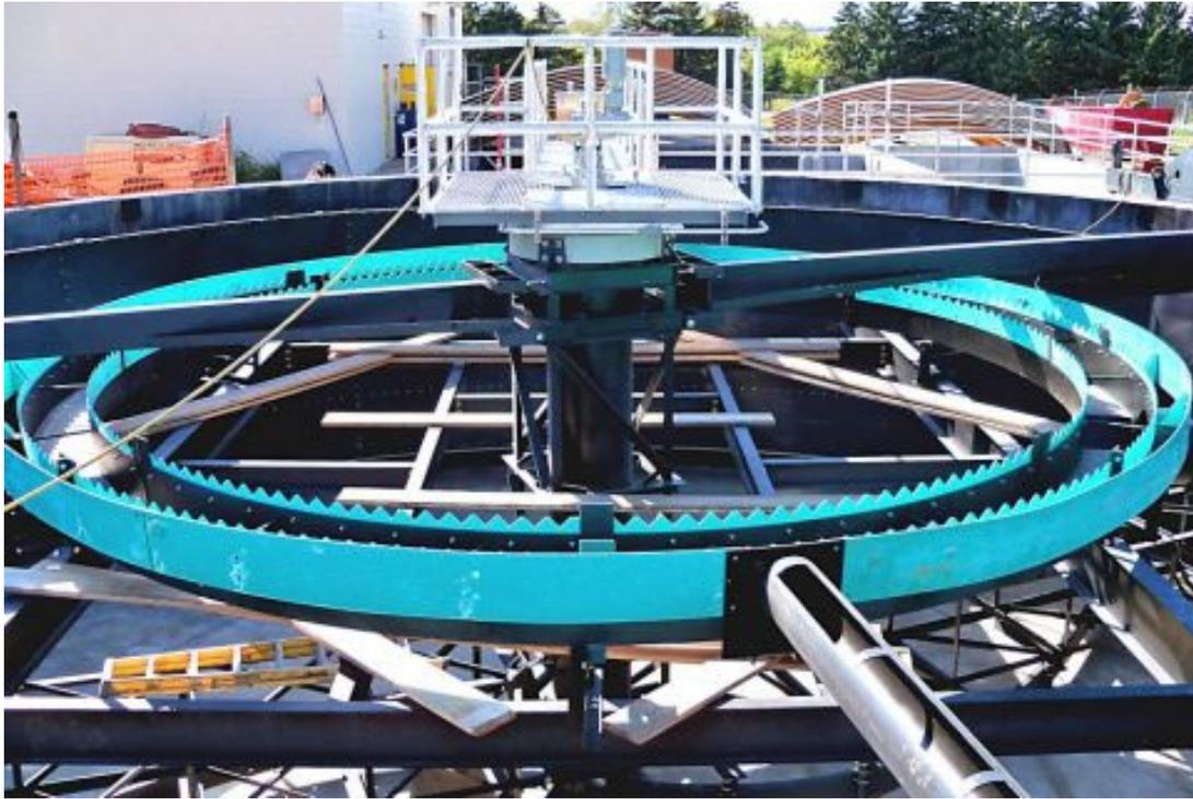
Holes in the bottom of the channel allow the influent to flow into the clarifier. The channel helps distribute the influent flow over the clarifier surface. Peripheral feed clarifiers may have either center take-off or peripheral.
