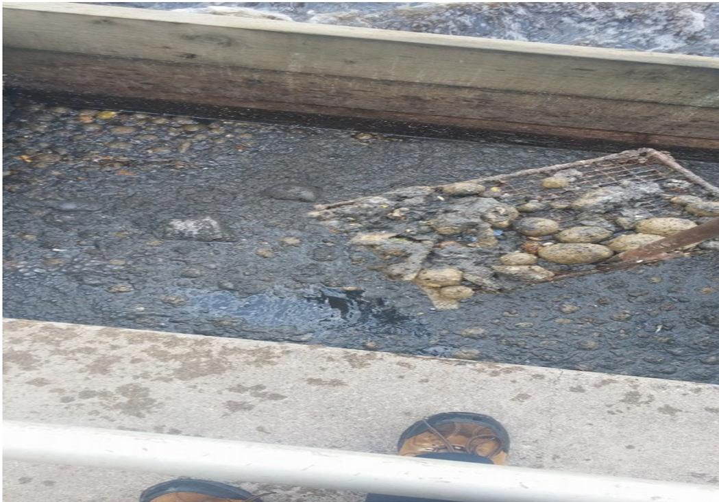
A buildup of grease balls in an oxidation ditch.
