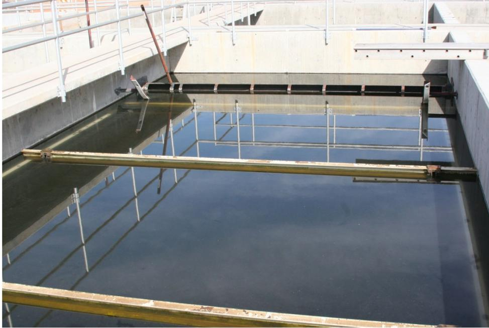
A **rectangular clarifier** used in the secondary settling process. Operation changes should be employed if a dark brown foam develops on the aeration basin, primary option is to increase the wasting rate.
