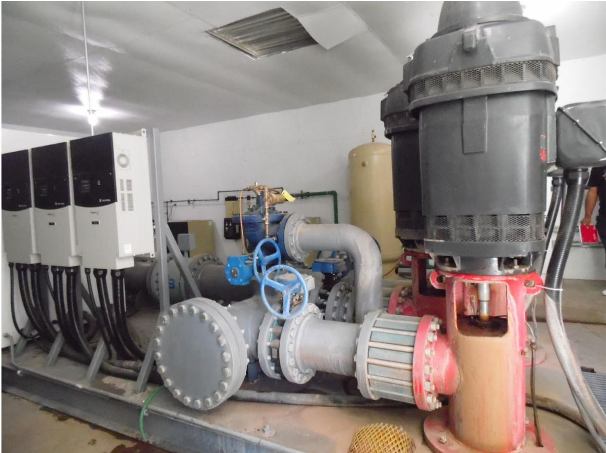
An **electric motor** is an electrical machine that converts electrical energy into mechanical energy. Most electric motors operate through the interaction between the motor's magnetic field and electric current in a wire winding to generate force in the form of rotation of a shaft.
