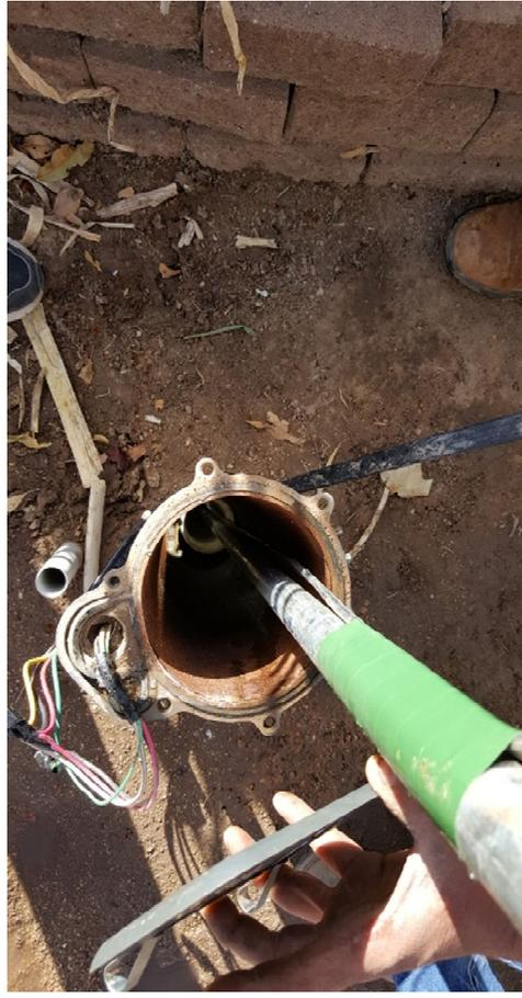
The discharge side of the pipe has a tee that seats on a saddle down below ground to prevent freezing.
