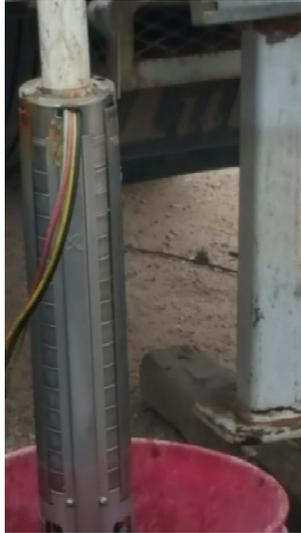
The PVC pipe is threaded into the pump assembly. The PVC is special pre-threaded pipe.
