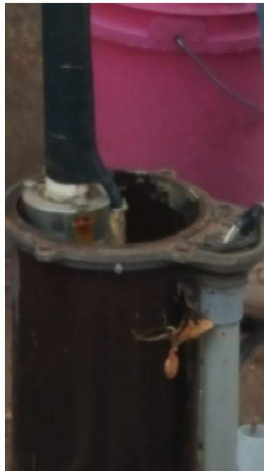
This pump has 16 stages and a 4 inch impeller. Rule of thumb, if you take the diameter of the impeller squared ( 4 x 4 ) and times it by the stages you will get the lift in feet. For example  $4 \times 4 \times 16 = 256$  ft of lift.
