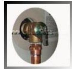
All domestic water heaters are required to be equipped with a relief valve as a safety feature to prevent damage from excessive pressure and temperature. There is always danger that this valve may become frozen or corroded from long disuse. For this reason, it is advisable to trip the lever of this valve manually every two or three months to be sure it will operate freely if an emergency arises.
