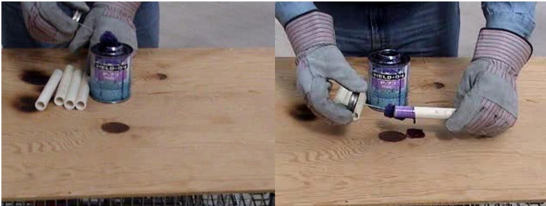
3. Apply a heavy, even coat of CPVC primer (if necessary) to the fitting. Remember, Ladies first. Use the right applicator for the size of pipe or fittings being joined. The applicator size should be equal to 1/2 the pipe diameter. It is important that a satisfactory size applicator be used to help ensure that sufficient layers of cement are applied.
