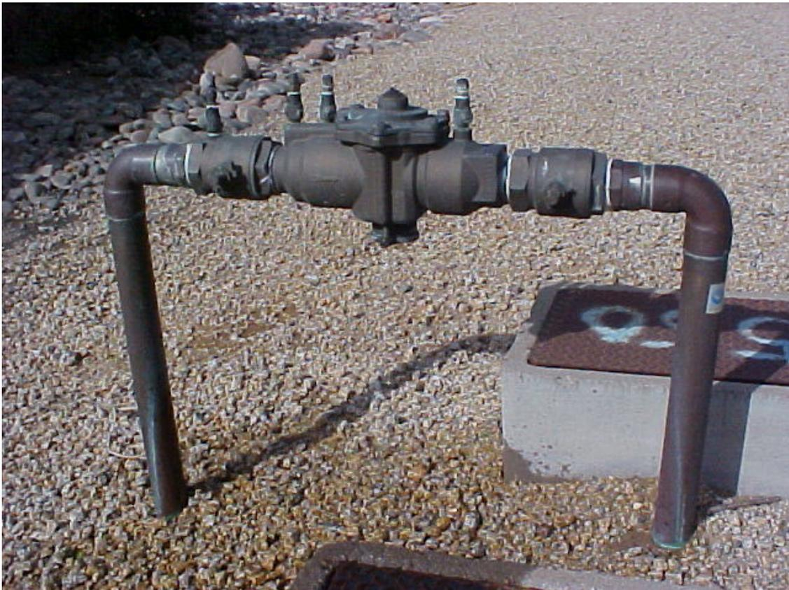
Leaky RP probably has some debris in the pressure differential area or in the hydraulic relief valve area.
