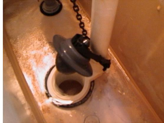
When we press the handle on the tank (not shown here), the flapper valve is opened and the water stored in the tank is released into the bowl at a very fast rate causing the water level in the bowl to rise and overflow rapidly. The rising water seeks its own level and overflows down the trap creating a siphon that literally sucks the water out of the bowl.
