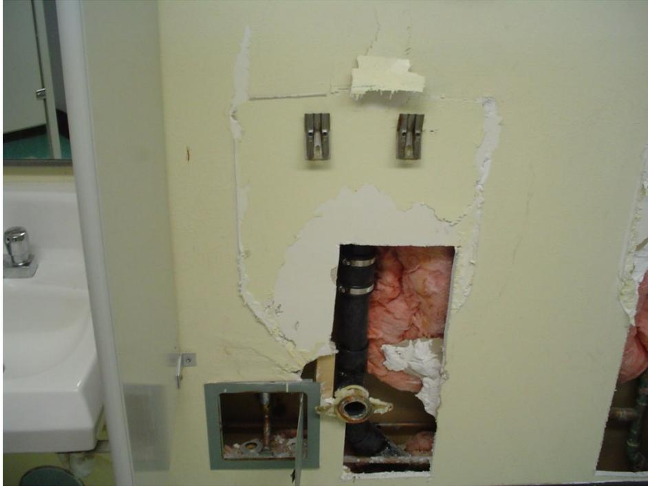
Prepare for extensive wall damage when retrofitting to a waterless urinal. You may need to replace tiles and drywall. Notice the square box on the right hand side, this is a trap primer for the floor drain. The trap primer keep a small amount of water to keep the drain's trap wet to prevent sewer odors from coming up.
