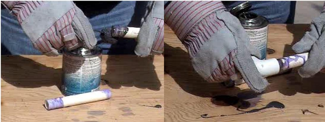
**5.** Apply a heavy, even coat of CPVC cement (if necessary) to the fitting. Remember, Ladies first; then apply to the pipe end. Stir the cement or shake can before using. Using the proper size applicator for the pipe size, aggressively work a full even layer of cement onto the pipe end equal to the depth of the fitting socket -do not brush it out to a thin paint type layer, as this will dry within a few seconds.
