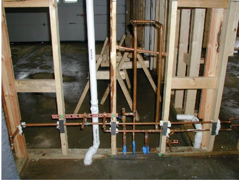
Lavatory or bathroom set-up with a Dirty Arm and possible water softener loop.
