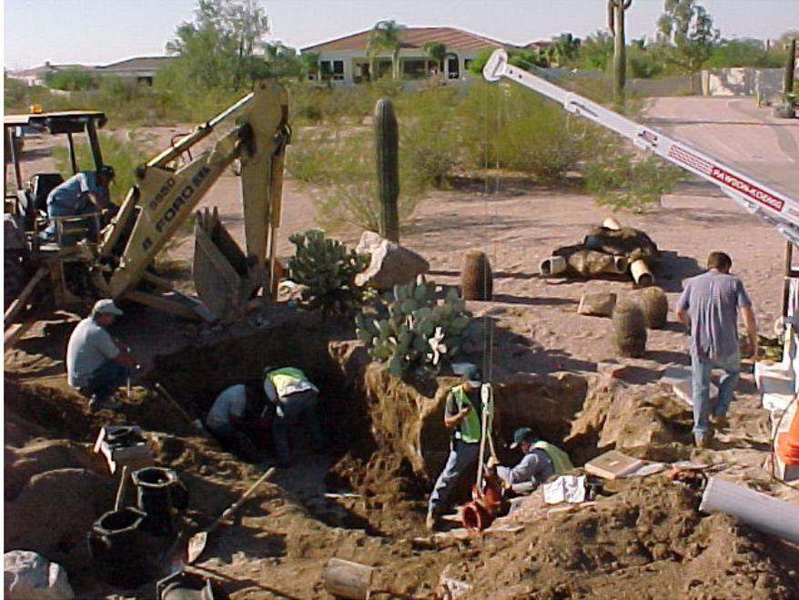
Top photograph, two gate valves blew out, you can see the kickers or thrust blocks in the back ground. Bottom photograph, a tapping machine and a new gate valve. These tapping machines are very expensive.
