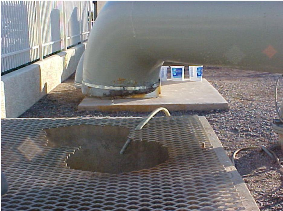
Notice the larger pipe is an approved air gap, but what about the smaller drain in the rear?
