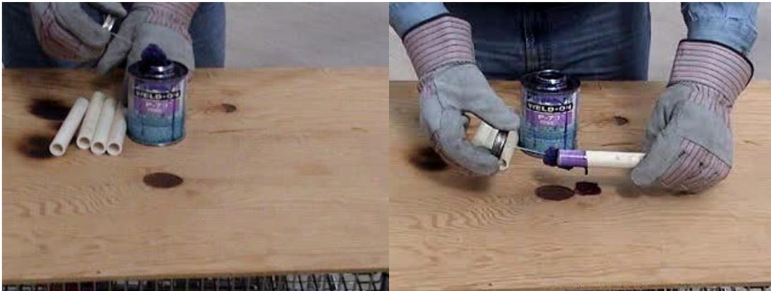
3. Apply a heavy, even coat of CPVC primer (if necessary) to the fitting. Remember, Ladies first. Use the right applicator for the size of pipe or fittings being joined. The applicator size should be equal to 1/2 the pipe diameter. It is important that a satisfactory size applicator be used to help ensure that sufficient layers of cement are applied.
