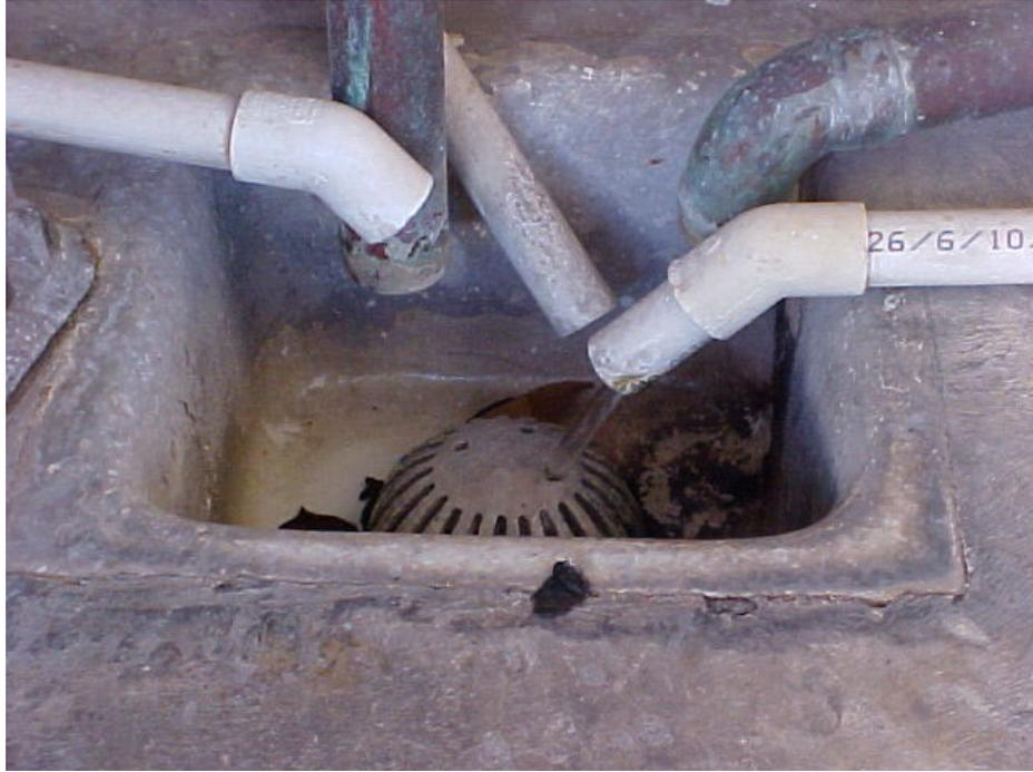
Which of these ice machine drains are approved air gaps?
