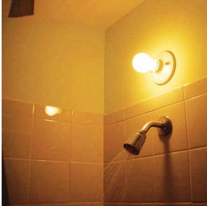
Top photograph, never install electricity near a water outlet.
