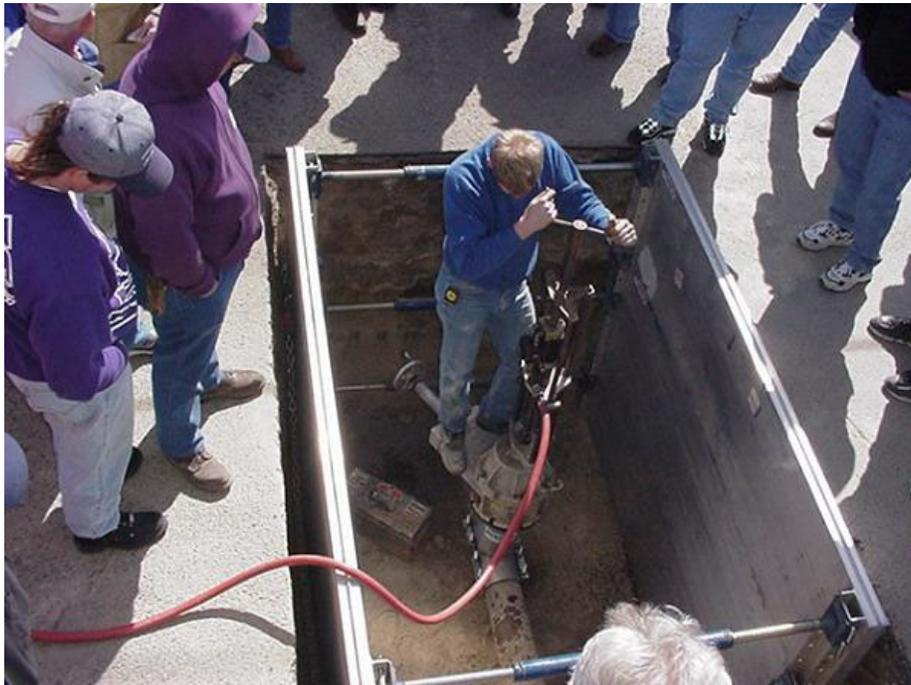
Hydro-stop valve insertion machine
