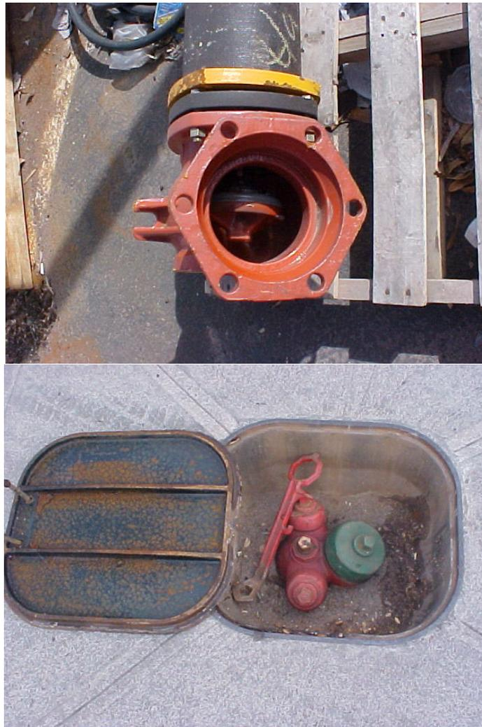
Bottom of a dry barrel fire hydrant--there is a drainage hole on the back of this hydrant, sometimes referred to as a "weep hole". Below is an "Airport Runway" type of hydrant.
