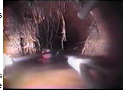
joint, tree roots will penetrate the opening to reach the nutrients and moisture inside the pipe. This phenomenon continues in winter even though trees appear to be dormant.
