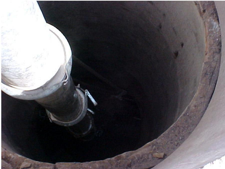
A Vactor clearing a Manhole.
