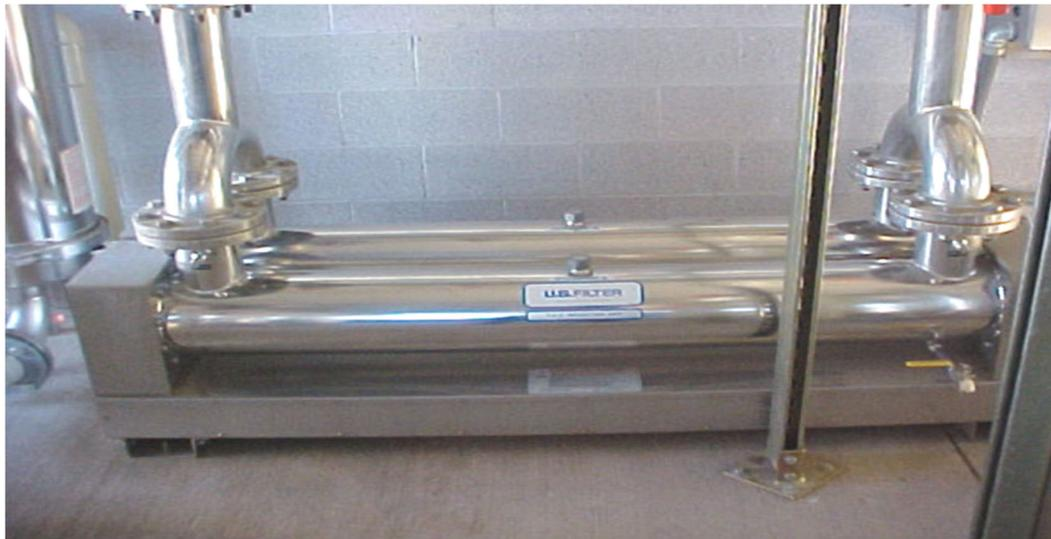
The lamp itself does not come in to contact with water, the lamp is placed inside a quartz tube, and the water is in contact with the outside of the quartz tube. Quartz is used in this case since practically none of the UV rays are absorbed by the quartz, allowing all of the rays to reach the water. Ordinary glass cannot be used since it will absorb the UV rays, leaving little for disinfection.
