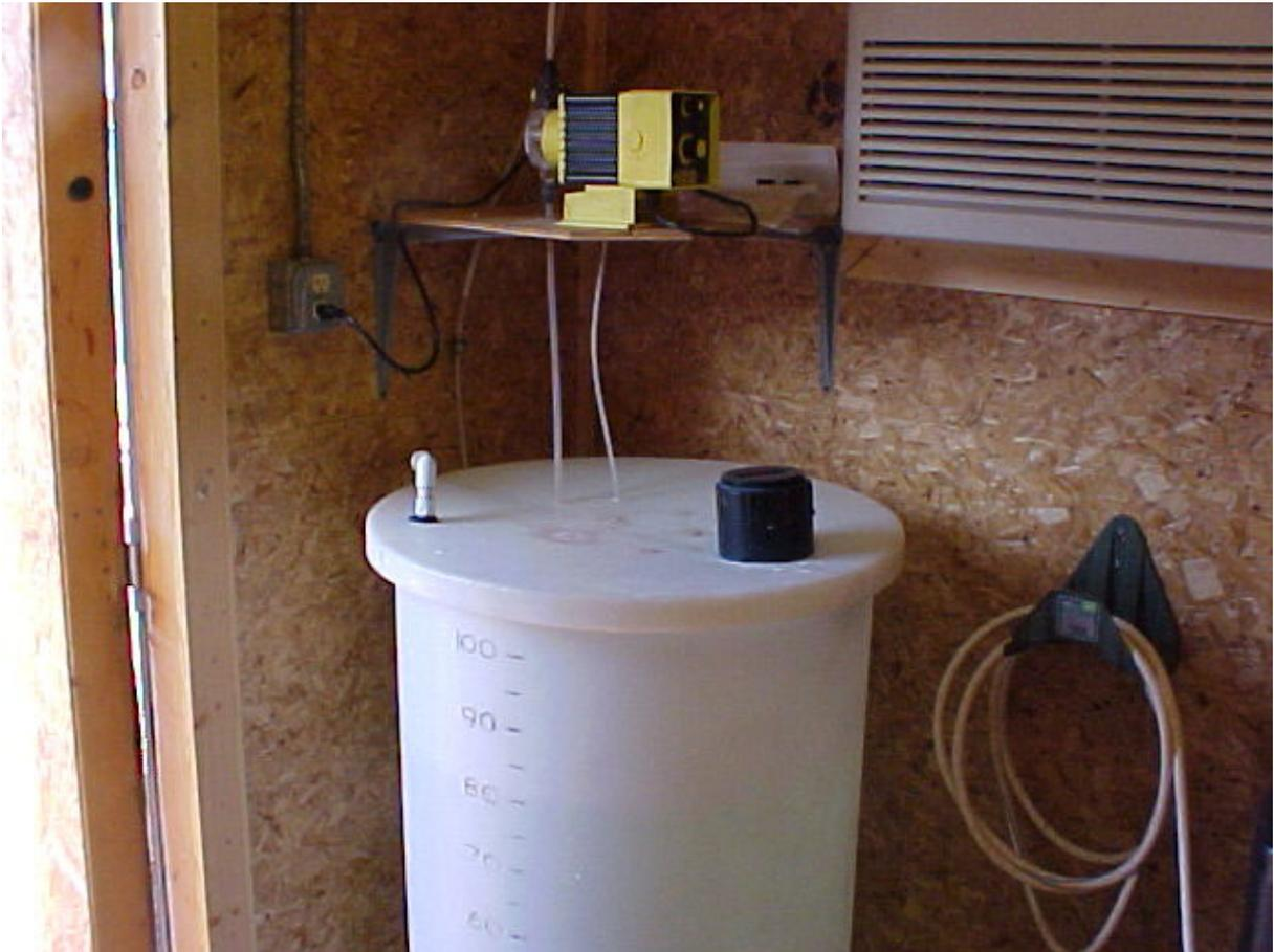
Small chlorine solution tank, normally found on small wells or post-chlorination areas in the distribution system
