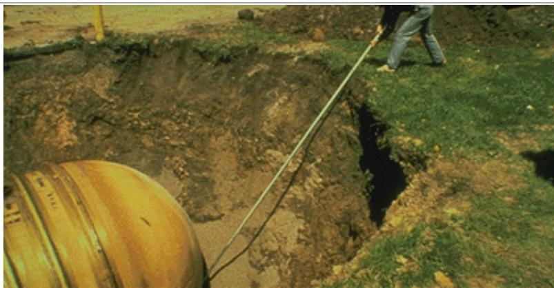
Installing a FRP tank.
