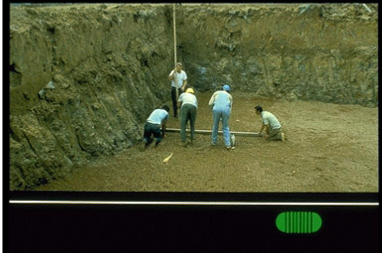
Inspecting the depth and grade of an UST excavation.
