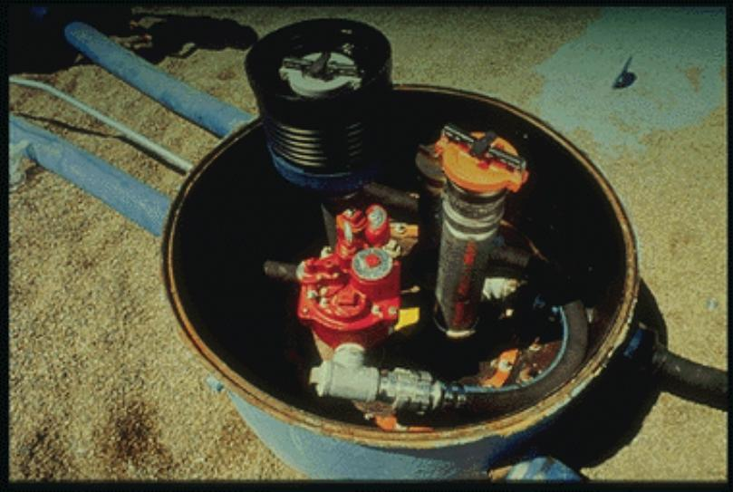
Open manway showing catch basin and pressurize piping (without line leak detector installed [yet?]).
