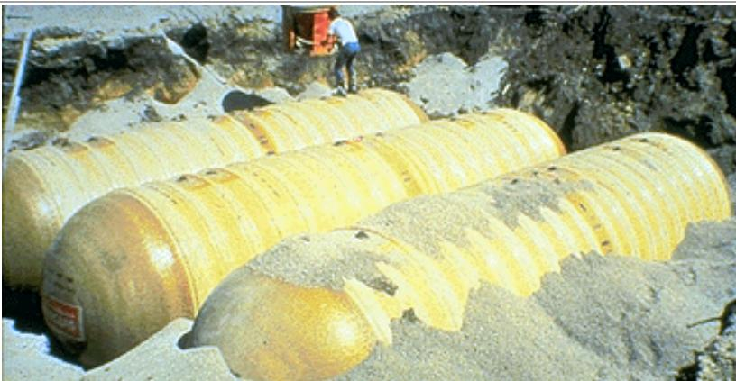
Backfilling new FRP tanks.
