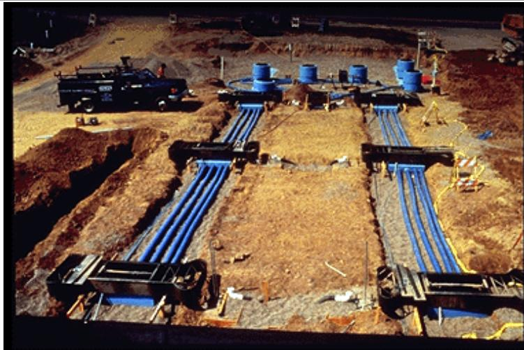
New piping and overfill protection at a new installation.
