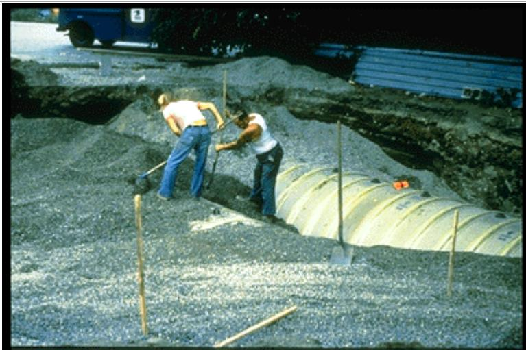
Backfilling FRP tanks.
