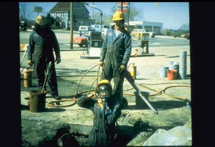
Entering a partially exposed UST using proper confined space entry techniques.
