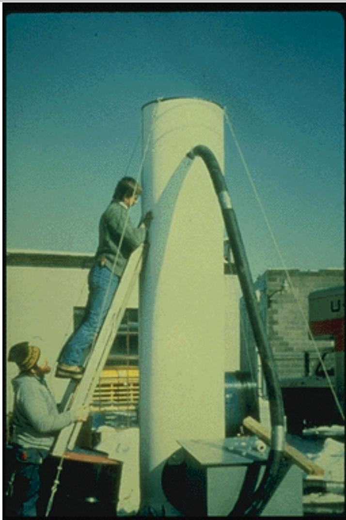
Air-stripping tower for treatment of contaminated groundwater.
