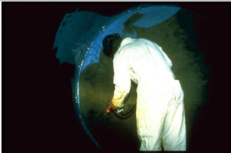
Applying the coating to the inside of a properly prepared UST.
