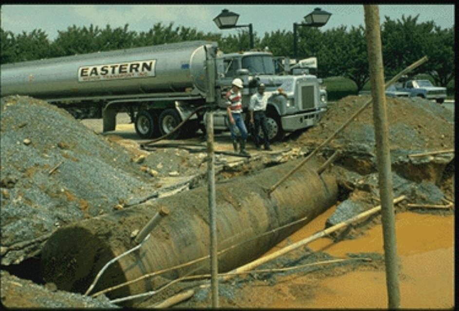
Rainwater which partially filled the UST excavation caused an UST to float and roll over to one side complicating removal.
