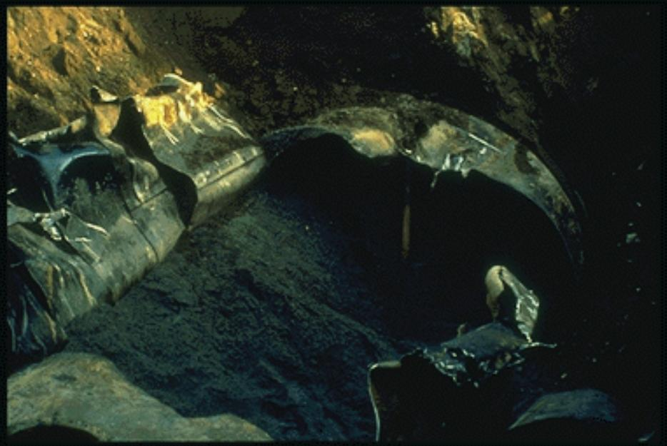
A partially excavated UST being filled with an inert material for disposal-in-place.
