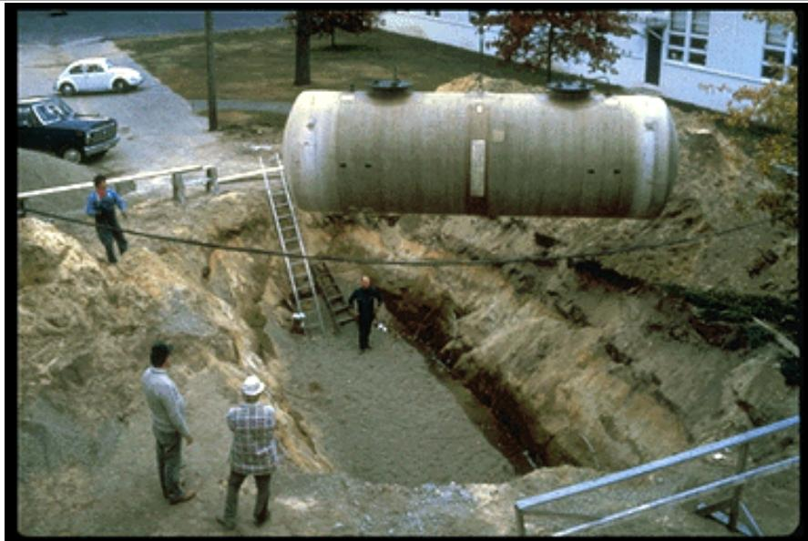
Lowering a fiberglass tank into an excavation.
