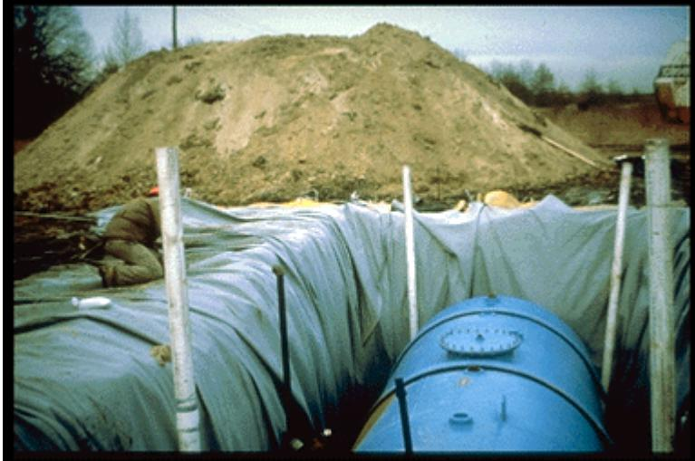
A steel tank installed in a lined excavation.
