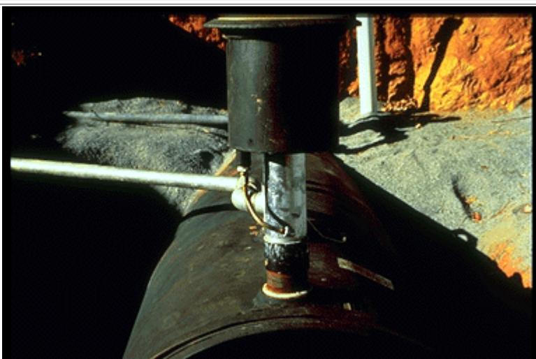
A spill bucket on a newly installed steel UST.
