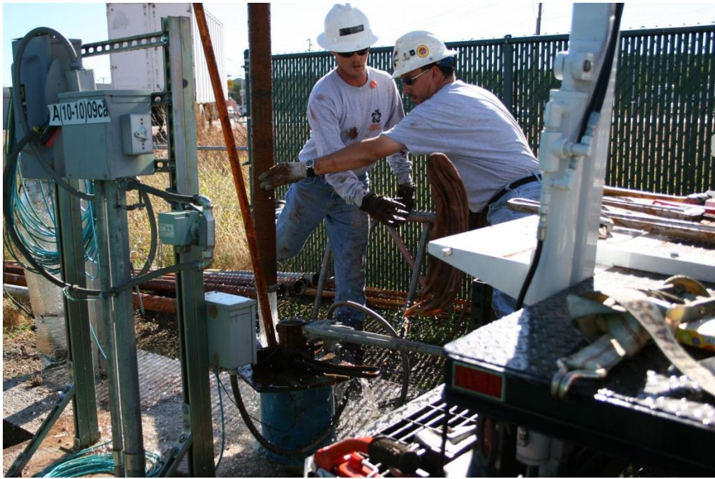
Top, this crew is removing a pump from a contaminated groundwater well in hopes of re-building and cleaning the well to increase the water production. The water is then sent to the granular activated carbon (GAC) vessels in the lower picture for final cleaning before being delivered to water customers. This well was contaminated from the dry cleaning chemical known as Perc (PCE) or fugitive Tetrachloroethylene from a nearby Dry Cleaner facility.
