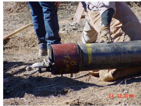
Cutting Shoe: The Cutting Shoe is welded to the bottom of casing before installation.
