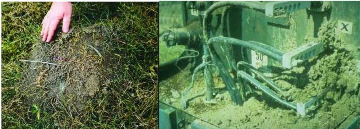
Fire ant mound; right side is Fire ant damage to an electrical transformer.
