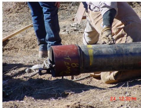
The Cutting Shoe is welded to the bottom of casing before installation.
