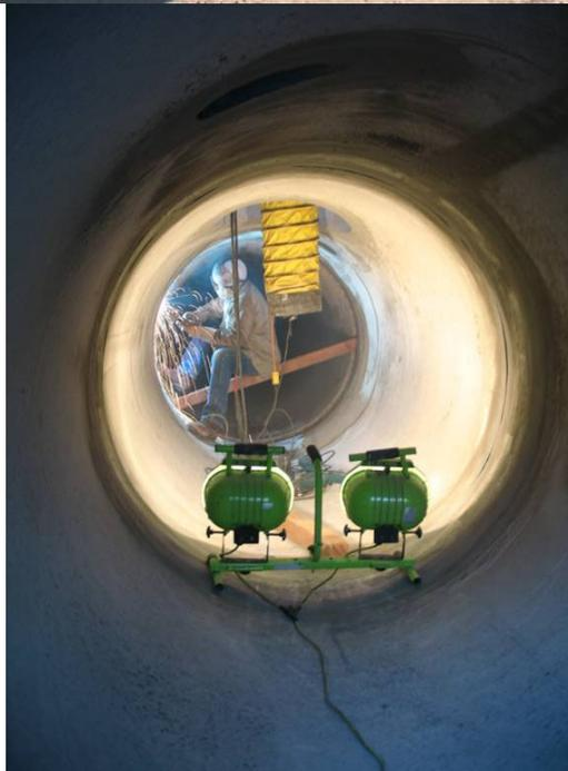
A broken 54-inch Butterfly valve and a worker inside the water main preparing the interior surface. Notice, this is a Permit Required Confined Space. A Hot work permit is also required.
