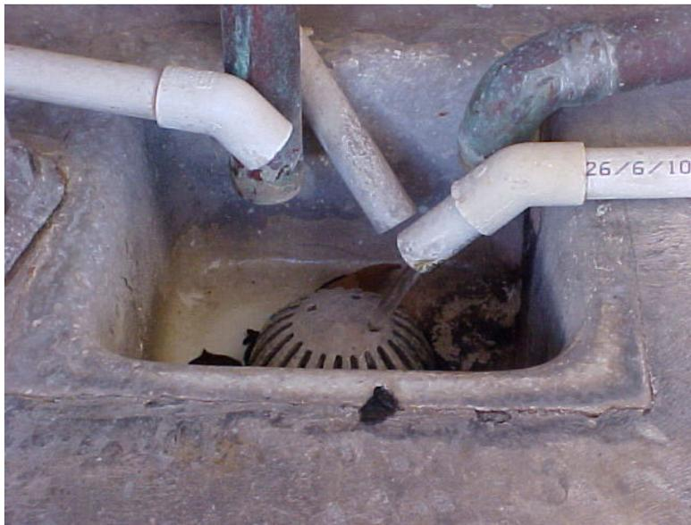
Which of these ice machine drains are approved air gaps?
