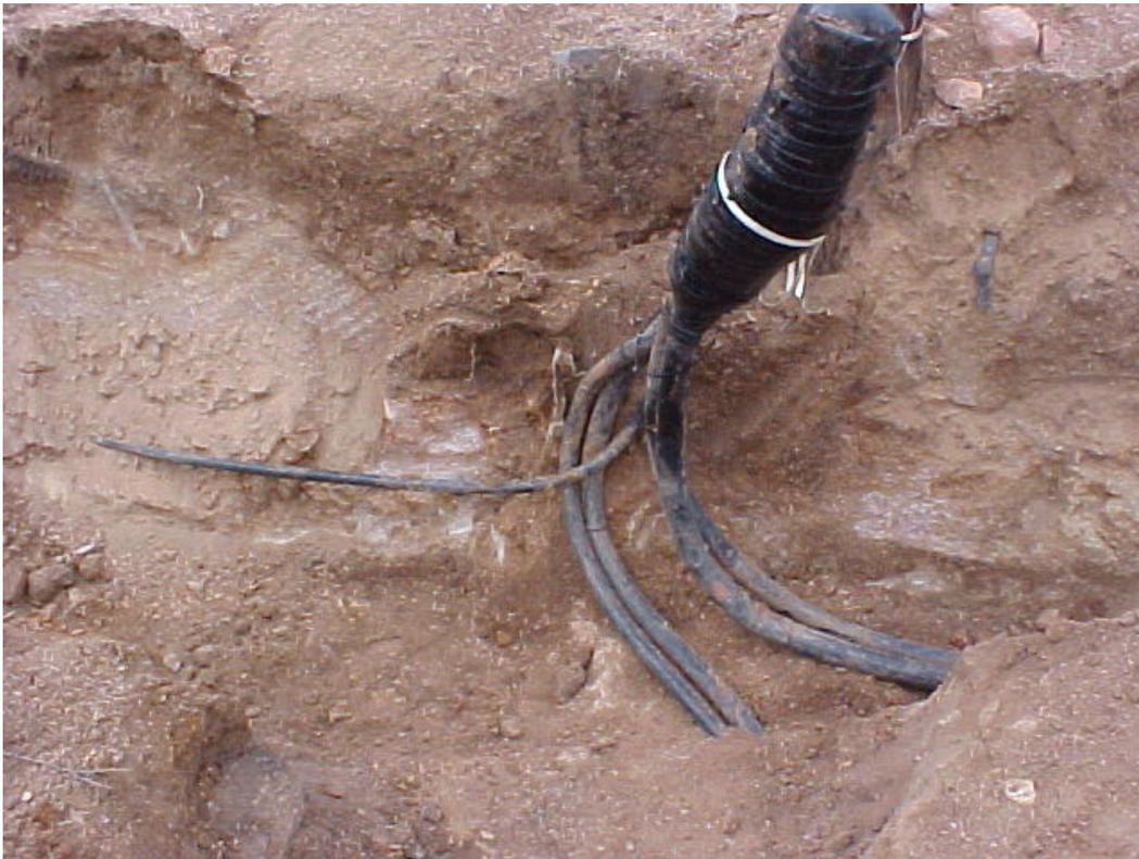
Buried Telephone Cables. Always hand dig around this stuff. There will be ties that you cannot even use a shooter shovel because of the damage that may be caused.
