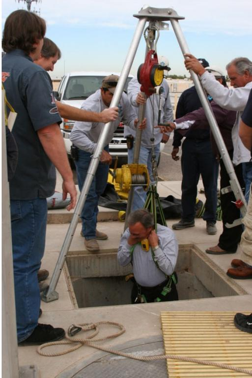
Dramatic rescue simulation using the tripod-retrieval system.
