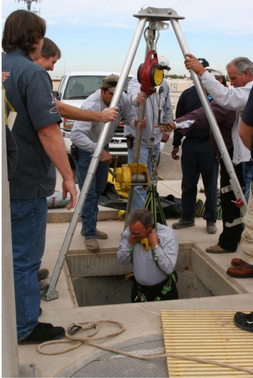
Dramatic rescue simulation using the tripod-retrieval system.
