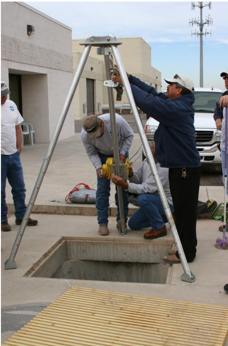
Tripod-retrieval assembly in use for an entry into one of the many confined spaces.
