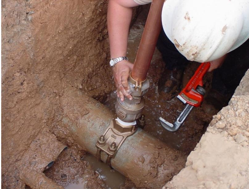
A water service worker installing a new copper water service line on an asbestos cement water main. Notice the bronze saddle with a corporation stop, a compression type fitting and a locking nut to secure the copper pipe to the corp. Bottom photo, the saw blade hole saw type tapping machine which was used to tap the main for the new service. This was completed with the water main under pressure so that other customers on the main did not have their water service disrupted due to the new service.
