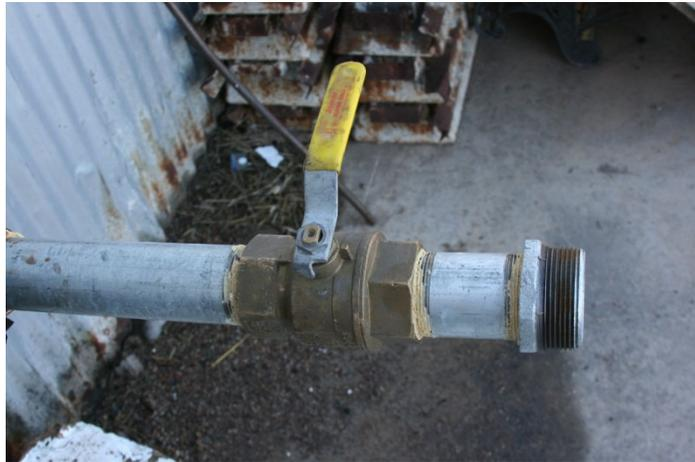
Most ball valves are the quick-acting type. They require only a 90-degree turn to either completely open or close the valve. However, many are operated by planetary gears. This type of gearing allows the use of a relatively small handwheel and operating force to operate a fairly large valve. Always follow standard safety procedures when working on a valve.
