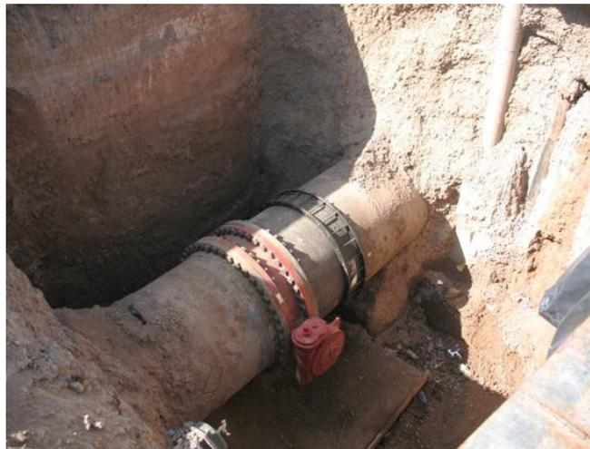
54 inch Butterfly valve on a huge transmission line. Nice job but no shoring, ladder or valve blocking.
