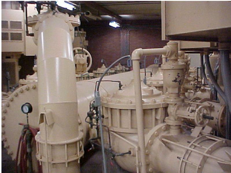
Looking inside of a booster pump station, notice the PRV and air relief valve.
