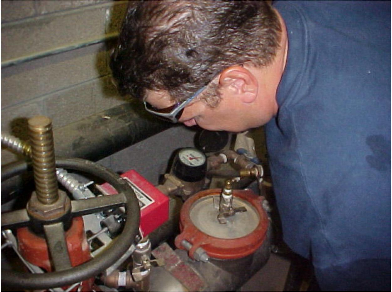
A Certified Backflow Tester examining a Double Check Detector Check fire line assembly. Notice the water meter which will detect any unauthorized water usage that is being used in the fire line. Yes, people can steal water through a fireline.
