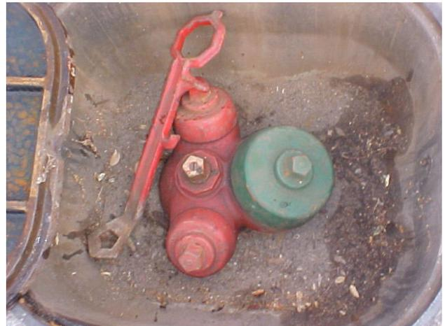
Left photograph-- the bottom of a dry barrel fire hydrant, there is a drainage hole on the back of this hydrant, sometimes referred to as a "weep hole". Right photograph-- an "Airport Runway" type of hydrant.
