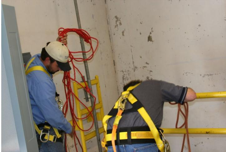
Example of a "**D-Ring**" and fall protection harness used when entering a confined space. The D-Ring provides a compatible anchor point for connecting devices such as lanyards or retractable lifelines. The shock absorbing lanyard provides a deceleration distance during a fall to reduce fall arrest forces for extra protection against injury.
