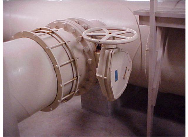
The valve should be installed in the closed position to ensure that the laminated seal in the disc is not damaged during installation.
