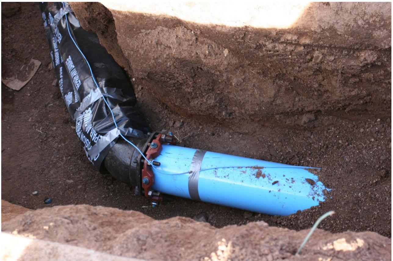
Photo of proper PVC to Ductile pipe with tracer wire and plastic installation. Notice restraining flang and missing poured kicker.
