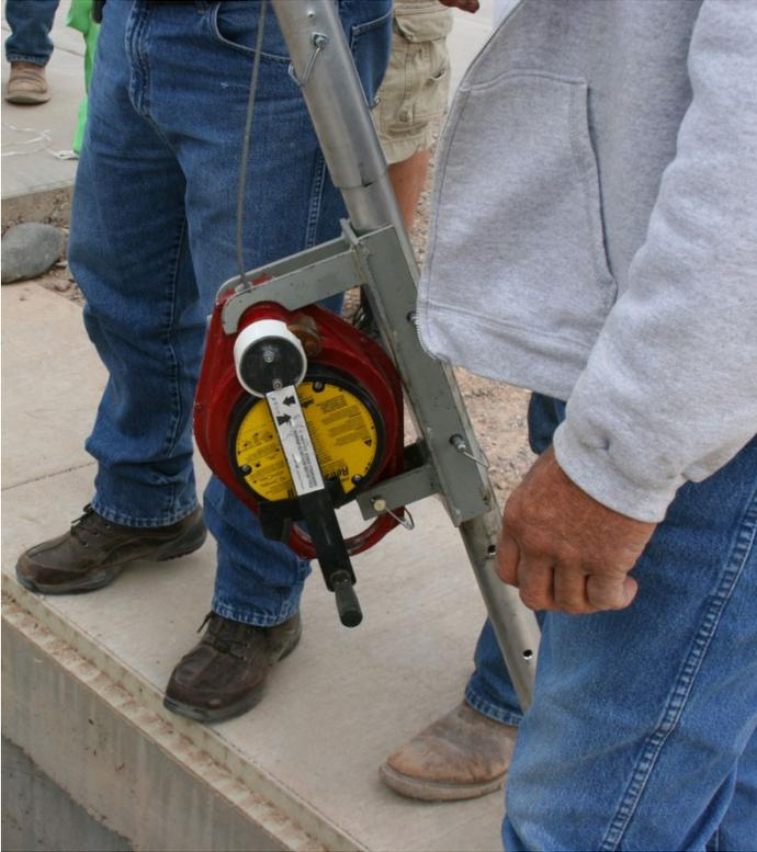
Checking the cable tension and inertial locking mechanism of the retrieval assembly.
