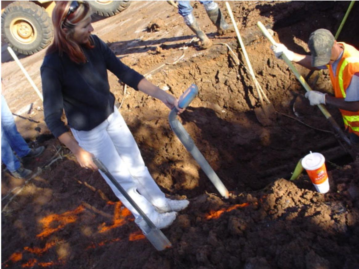
Always wait for the buried utilities to be marked before excavation begins. Believe it or not, this crew dug 9 feet deep before the Locator showed up and marked fiber optics in the same trench.
