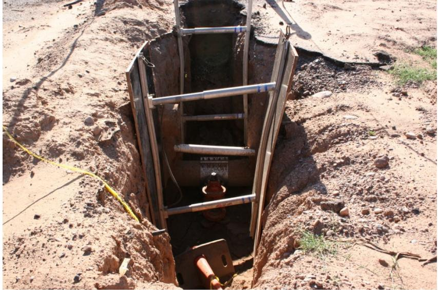
Within the OSHA regulations are Appendixes C and D, with tables and limitations for use of timber shoring and aluminum hydraulic shoring as a support system. Other shoring systems may be used if they are accompanied by tabulated data signed by a registered professional engineer or a specific shoring plan has been developed and signed by a registered professional engineer.
