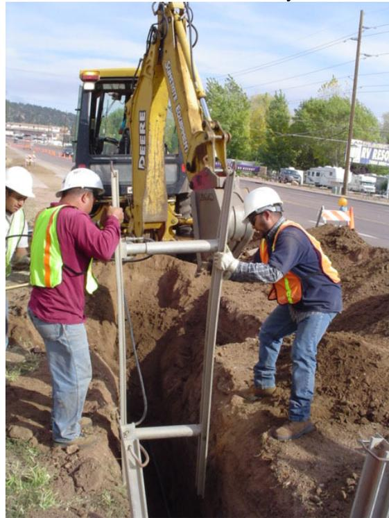
When the shores are hydraulically activated to the same pressure (psi) shown on the pump gauge, then each cylinder is exerting a uniform axial compressive load on the trench walls. For many types of cohesive soils, the load is dispersed within the trench walls into an arching effect. It is from this arching effect, used in conjunction with the rail strengths, that the horizontal and vertical distance between crossbraces (hydraulic cylinders) is calculated.
