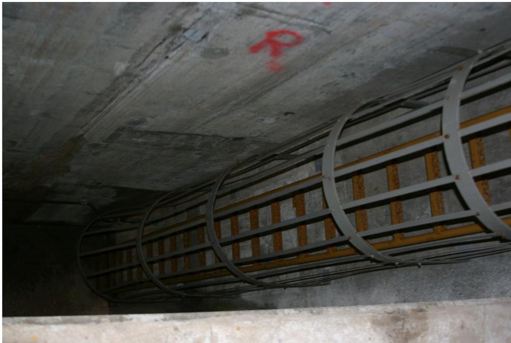
**Scenario.** A fixed ladder drops deep inside a permit required or type II confined space. One man goes inside and passes out from hazardous fumes. A second man goes in and dies within seconds trying to help his buddy.
