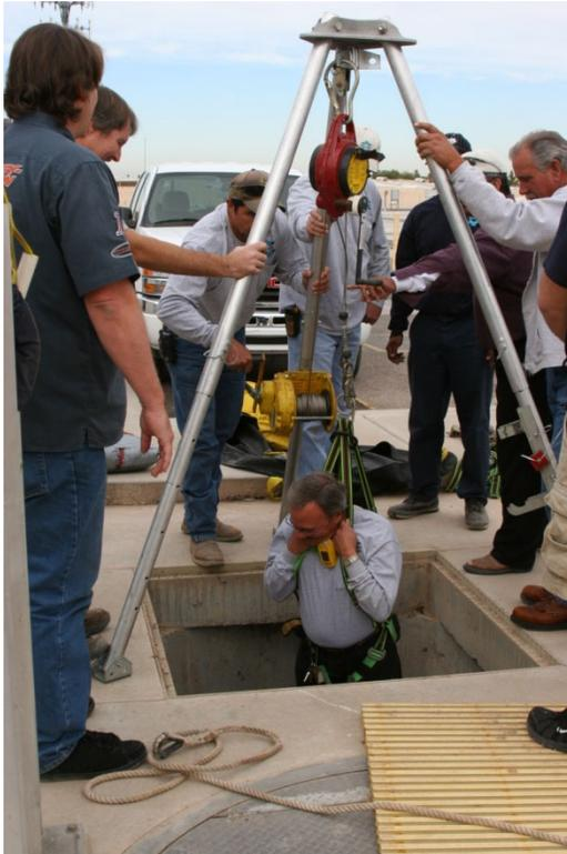
Dramatic rescue simulation using the tripod-retrieval system.
