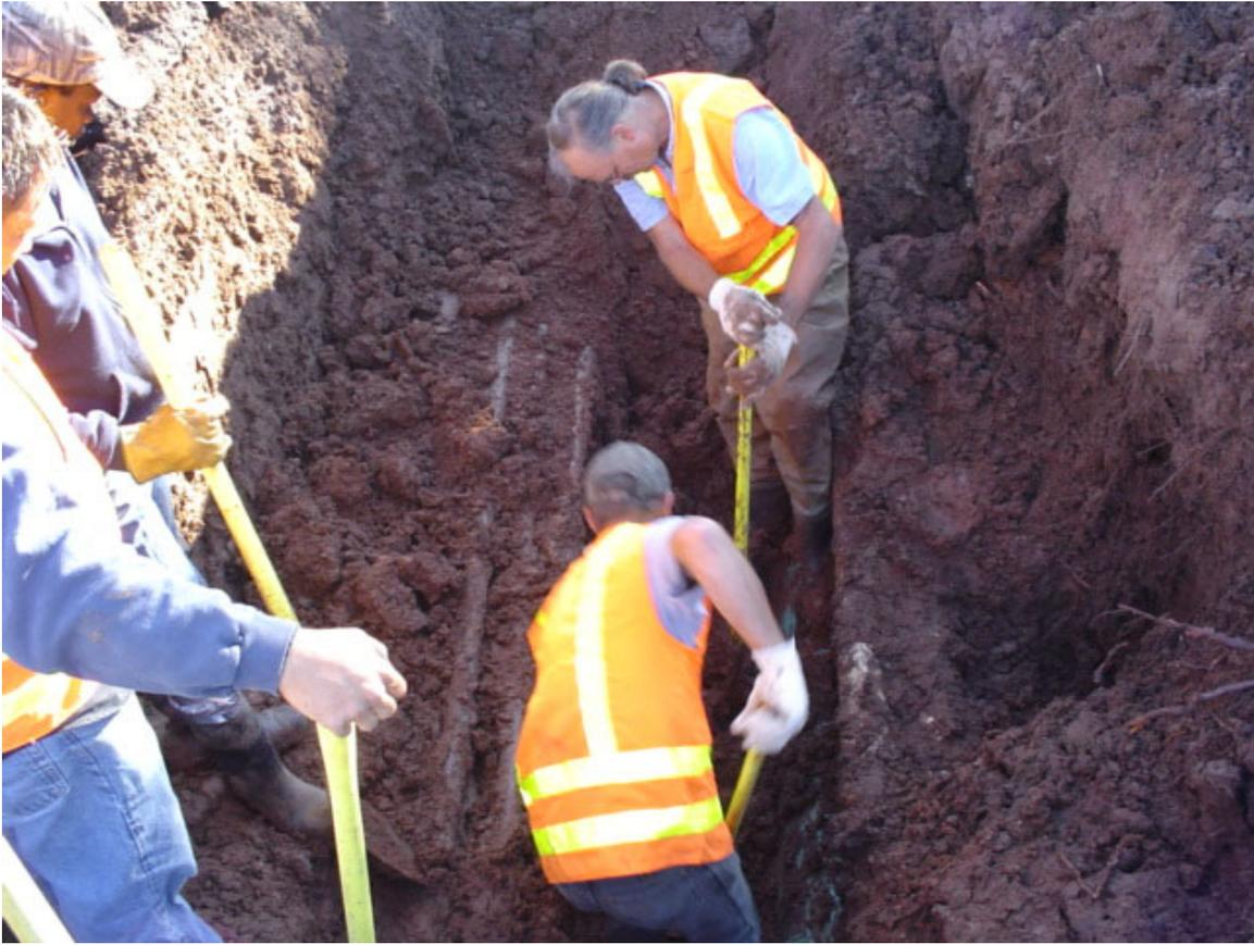
How would you make this excavation safe to work inside? The trench is 9 feet deep. OSHA Violations include no hard hats, no ladders, and no daily inspection form.
