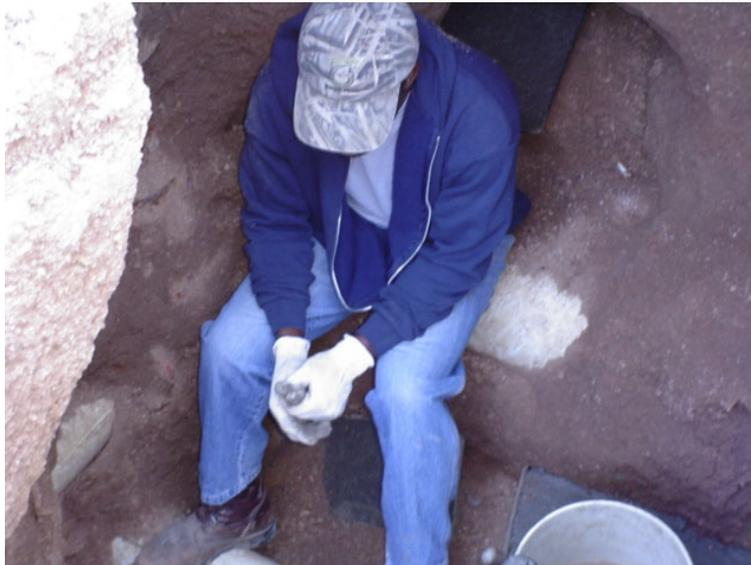
**OSHA Violation.** It is difficult to see, but this poor soul is inside a death trap. He is in a deep trench sitting in a bell-shaped hole, sitting on a sewer main. He has good shade from a steel plate that is covering the road with cars driving on top. No protection at all. There was a ladder about 50 feet away. Good luck!
