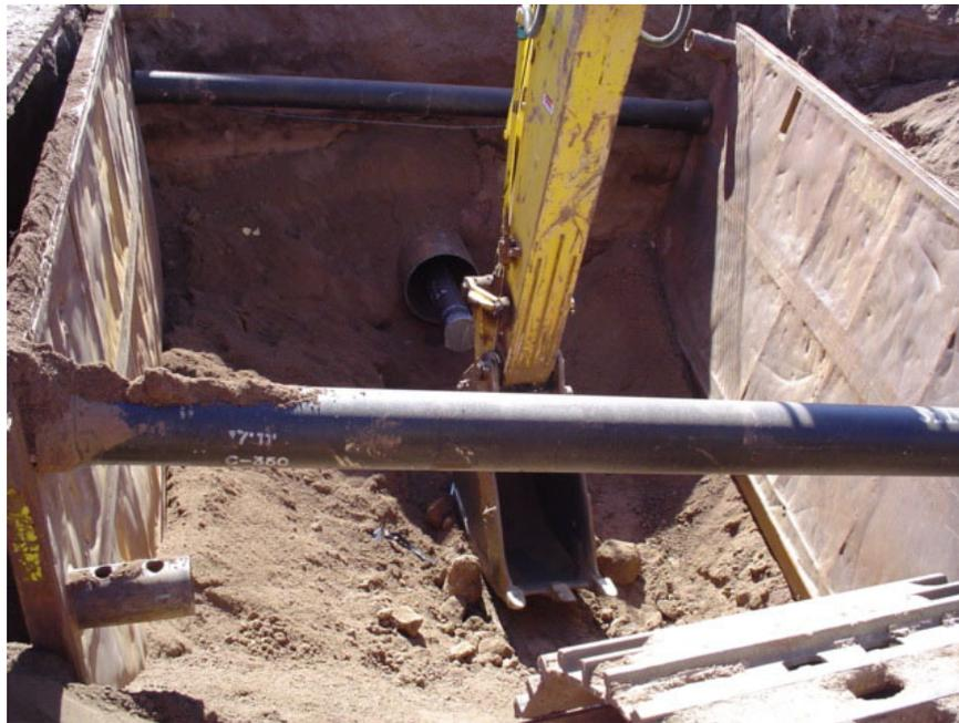
**OSHA Violation--**No ladders, but the best part is the homemade trench box using waterlines as the cross-braces. Remember, trench boxes and shields are a manufactured and engineered safety device that cannot be modified, especially by the competent person. This box collapsed in the hole. Workers must enter and leave the shield in a protected manner, such as by ladder within the shield or a properly sloped ramp at the end.
