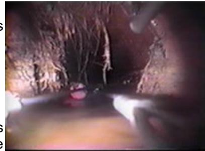
joint, tree roots will penetrate the opening to reach the nutrients and moisture inside the pipe.
