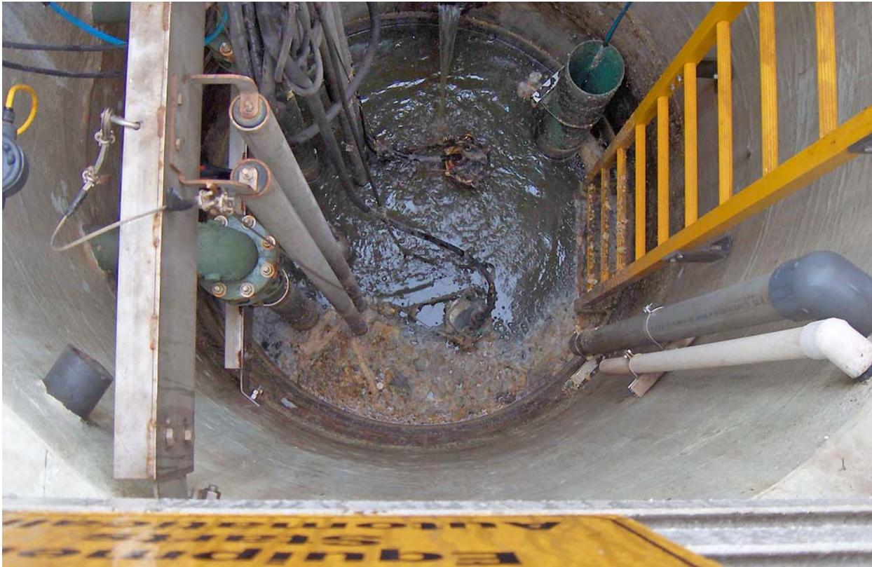
Wet-well maximum detention time in constant speed pumps is typically 20 to 30 minutes. Use of variable frequency drives for pump speed control allows wet-well detention time reduction to 5 to 15 minutes.
