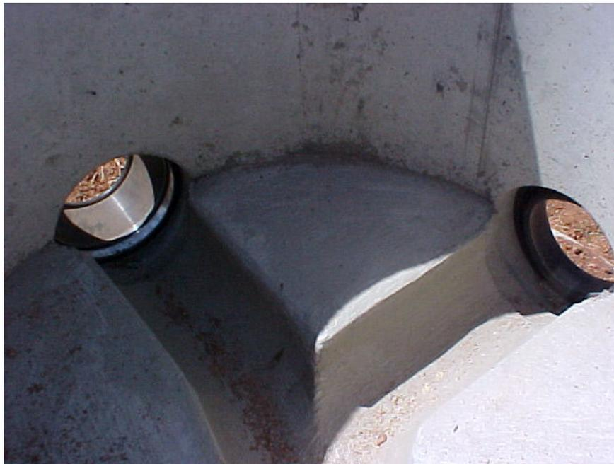
Inside a new manhole, the Invert is the inside bottom of the pipe. The Invert is used to determine the depth which is used to determine the Rise or Slope of the pipe.
