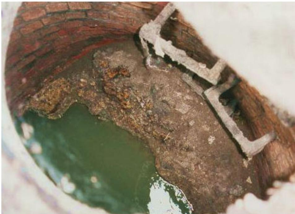
The corrosive effects of Sulfuric acid are created by Hydrogen Sulfide gas.
