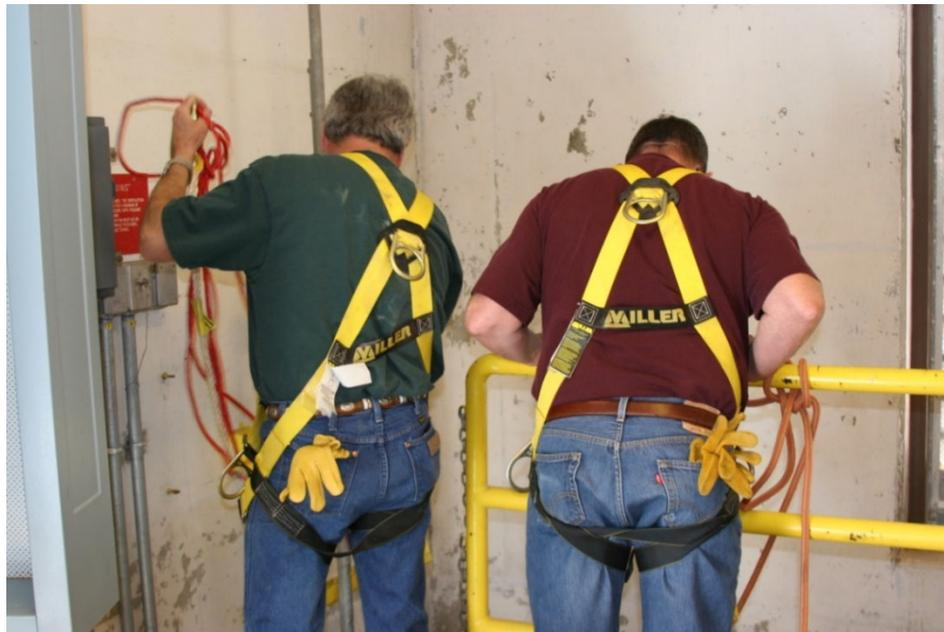
D-Ring on the rear of the harness is necessary for the entrant to be retrieved from the confined space.
