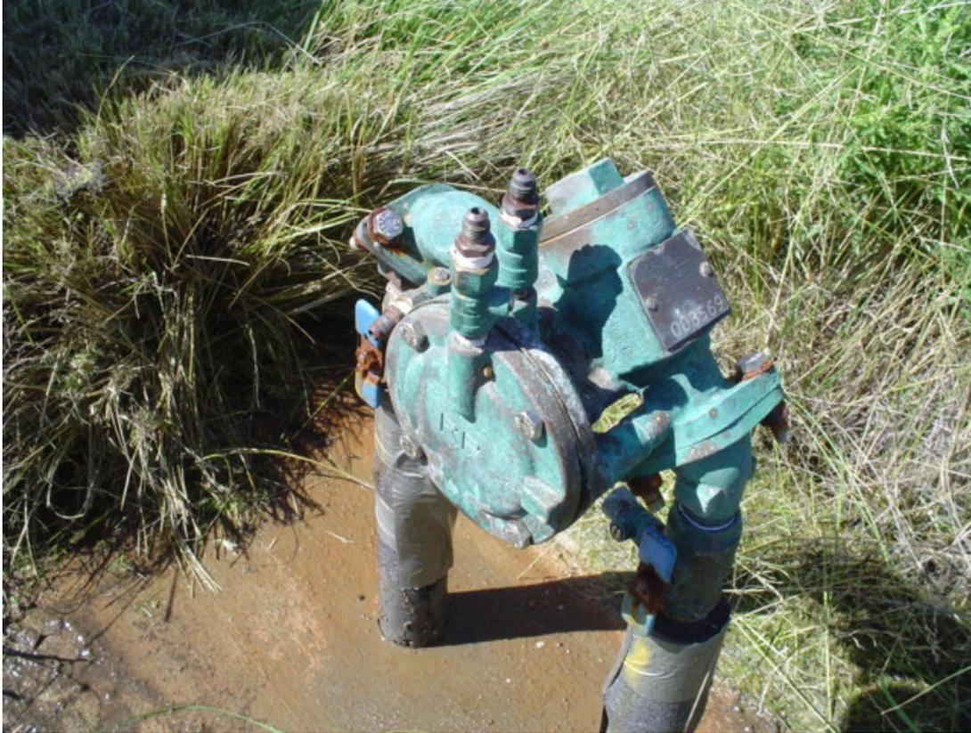
Here is an RP that had never been tested and leaked every day until the grass was 3 feet high and the owner notified the Water Department of a water leak. The water meter reader should have caught this problem in the first couple months.
