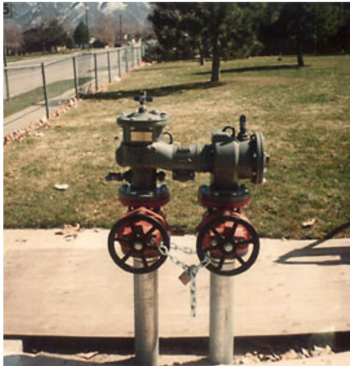
Double Check Backflow Assembly (Notice chain common on OS&Y).
