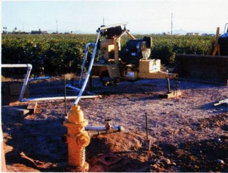
**Direct connection from hydrant to pump.**
