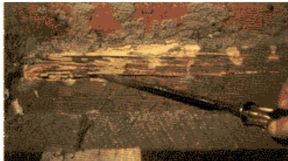
Using a screwdriver to probe and examine termite damage, Subs will go with the grain.
