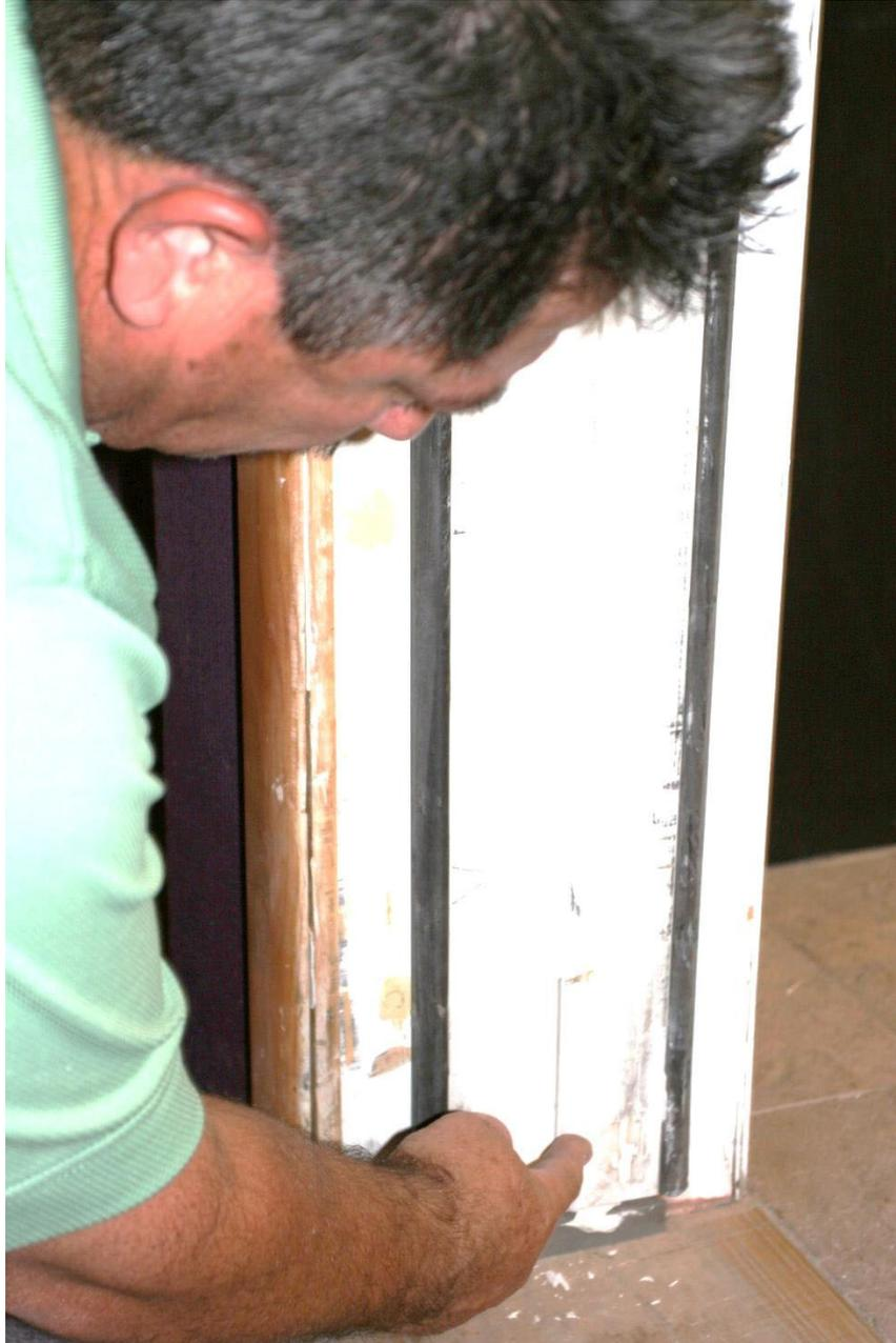
Probing interior wood trim reveals termite damage. Subterranean termites do not reduce wood to a powdery mass, and they do not create wood particles or pellets, as do many other wood-boring insects. Depending upon your State or climate, up to half of your work may be termite management. Termite control is an excellent profit making portion of normal pest control activities, however, it is very labor intensive at times.
