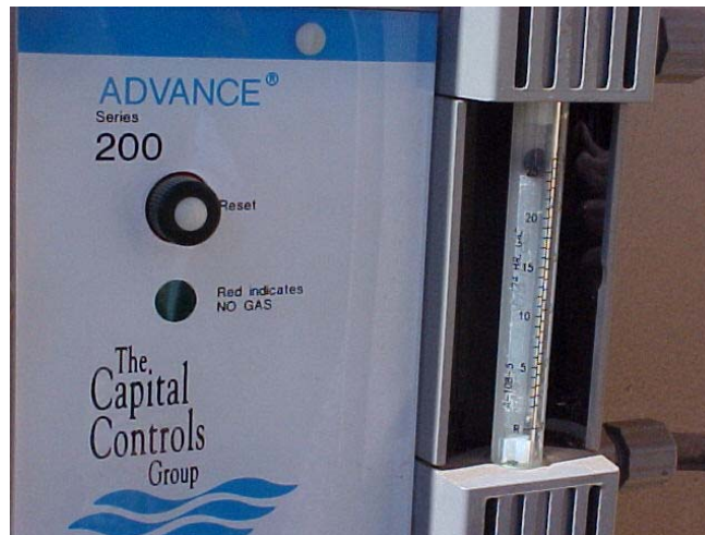
Chlorine measurement devices or Rotameters.
