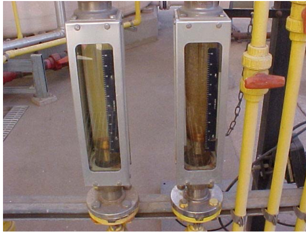
Chlorine measurement devices or Rotameters.
