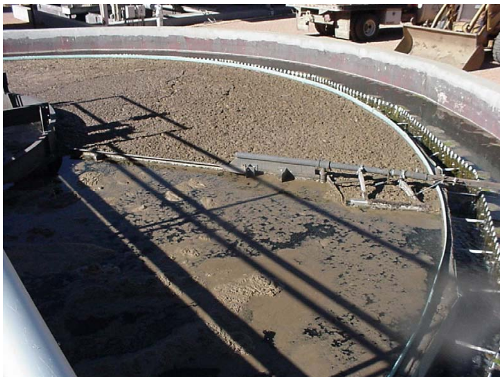
Primary Wastewater Treatment Clarifier
