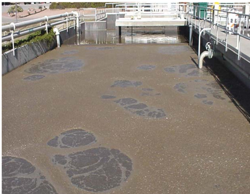
Activated Sludge Aeration Basin, identify by the bubbles.
