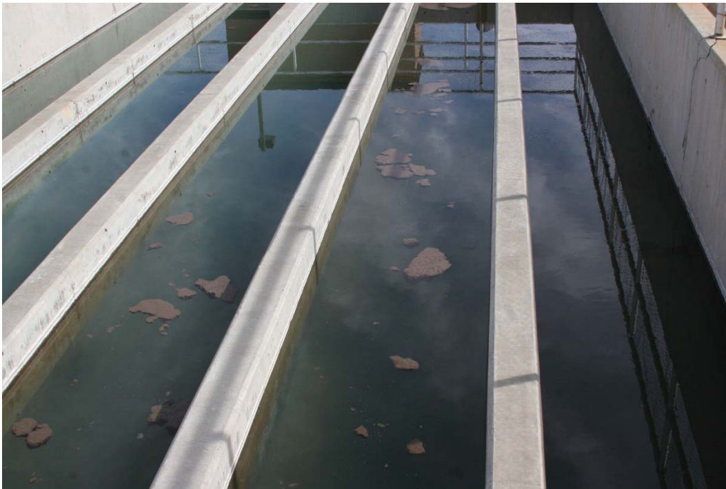
During a slight plant upset, sludge from the filters can be carried over to the chlorine contact channel.
