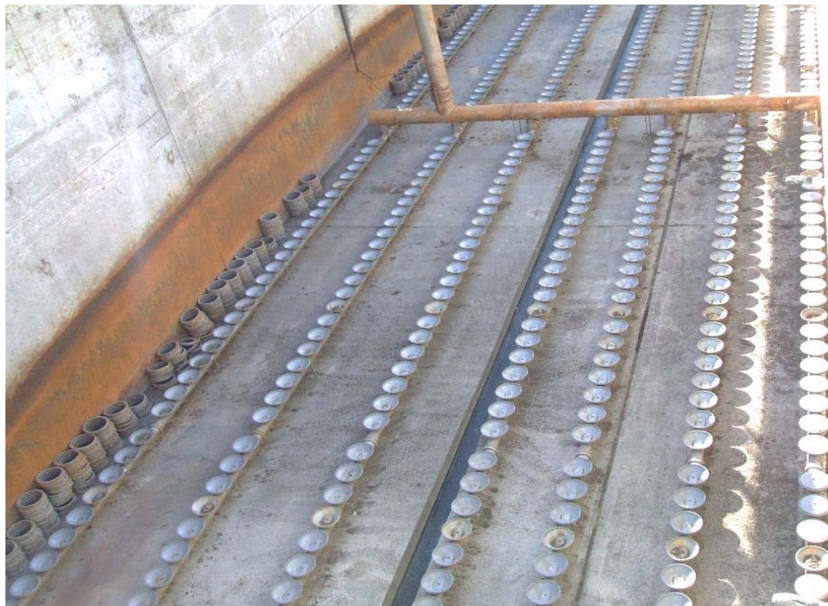
The same area from above photo, but clean and dry, these are porous air diffusers.
