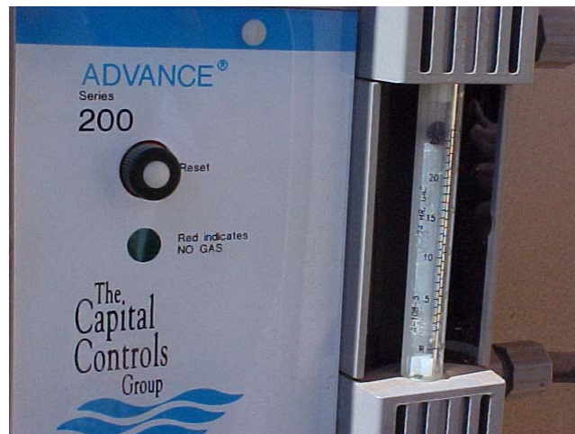
Chlorine measurement devices or Rotometers.
