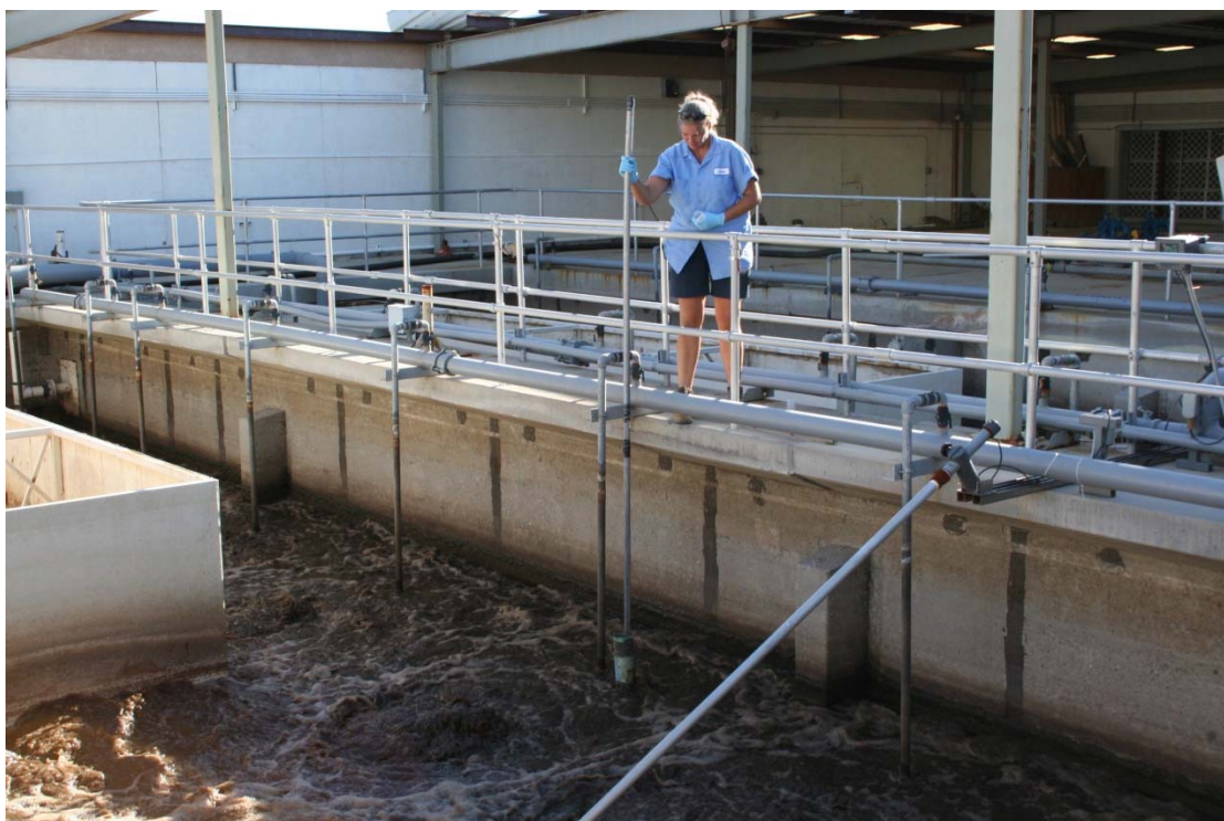
Sequence Batch Reactor Aeration sequence for an SBR.
