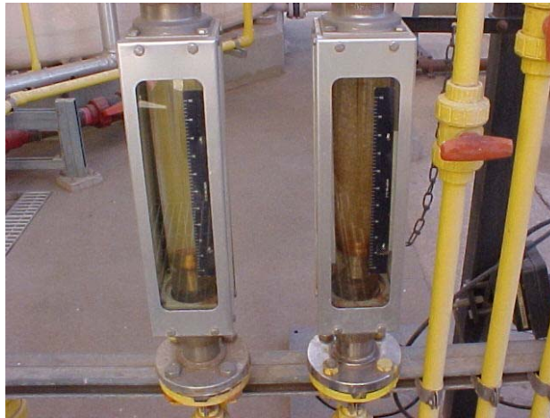
Chlorine measurement devices or Rotometers.
