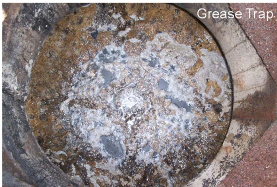
Top photo: Various pump damage from undesirable materials in the sewer system. Bottom photo, heavy grease from not being regularly pumped. Photograph credit John Bougham.
