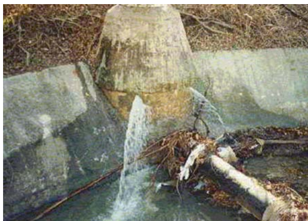
Above, a cracked sewer main, a SSO waiting to happen.
