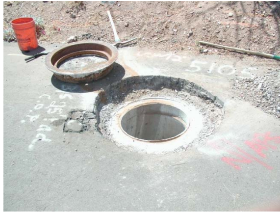
Raising the Ring, jackhammer, install the crown, patch the street.
