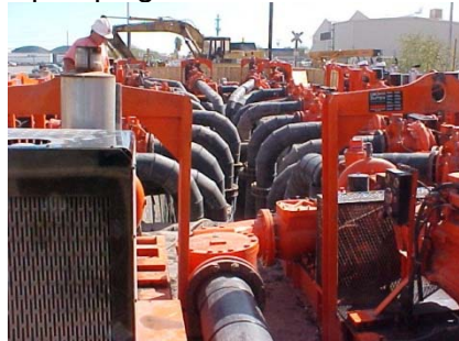
Pumps at a temporary sewer manhole by-pass.
