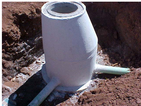
Newly finished Manhole and Laterals.
