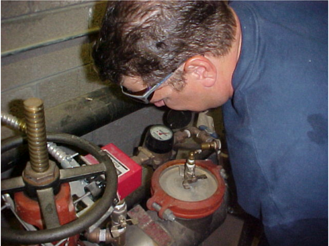
A Certified Backflow Tester examining a Double Check Detector check fire line assembly. Notice the water meter which will detect any water usage that be used in the fire line.
