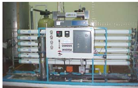
Packaged skid with instrumentation, UV, and softening.
