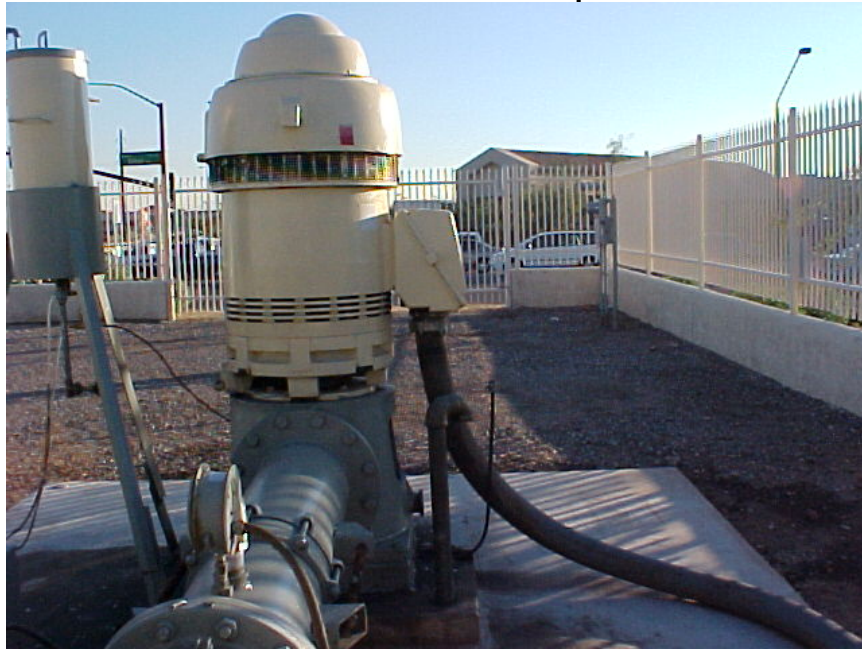
Vertical Turbine Pump
