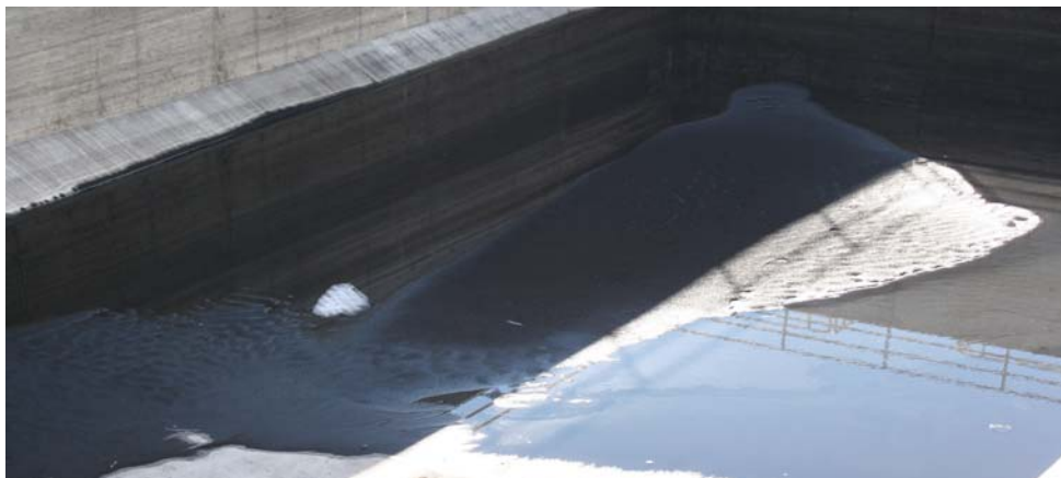
A picture of a backwash basin that has media caked on the bottom.
