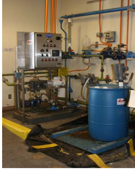
The photograph on the right is dry Polymer and on the left is liquid.
