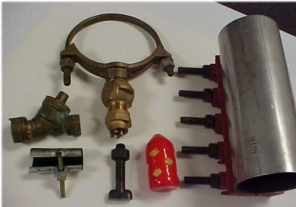
Common distribution fittings. Single check valve, Poly Pig, 1-inch repair clamp, 4-inch full circle clamp, T- Bolt and a corp. and saddle.
