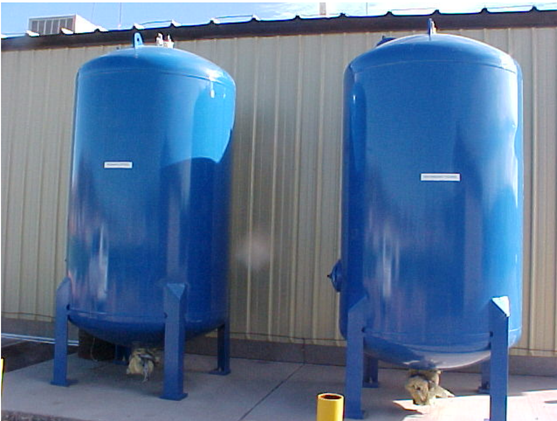
Carbon vessels used for taste and odor control
