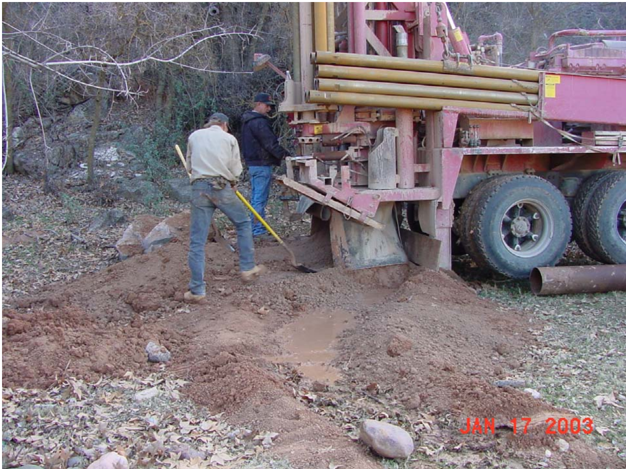
Drilling a new groundwater production well.
