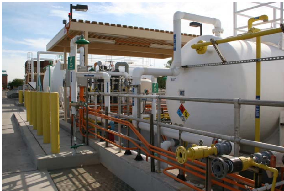
Hydrofluorsilicic Acid Tanks
