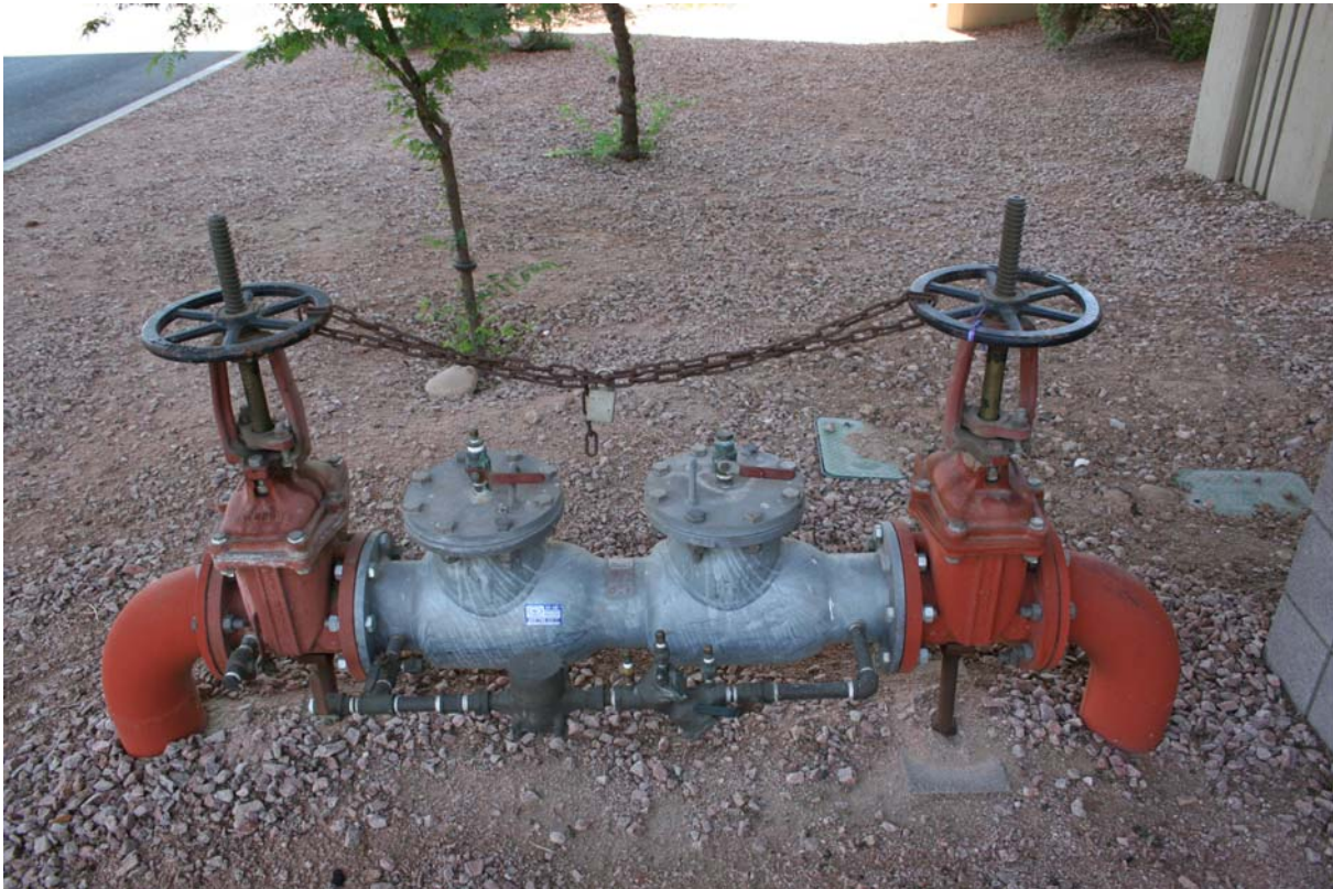
A DC on a fireline with OS& Y valve, notice the little DC with a water meter.
