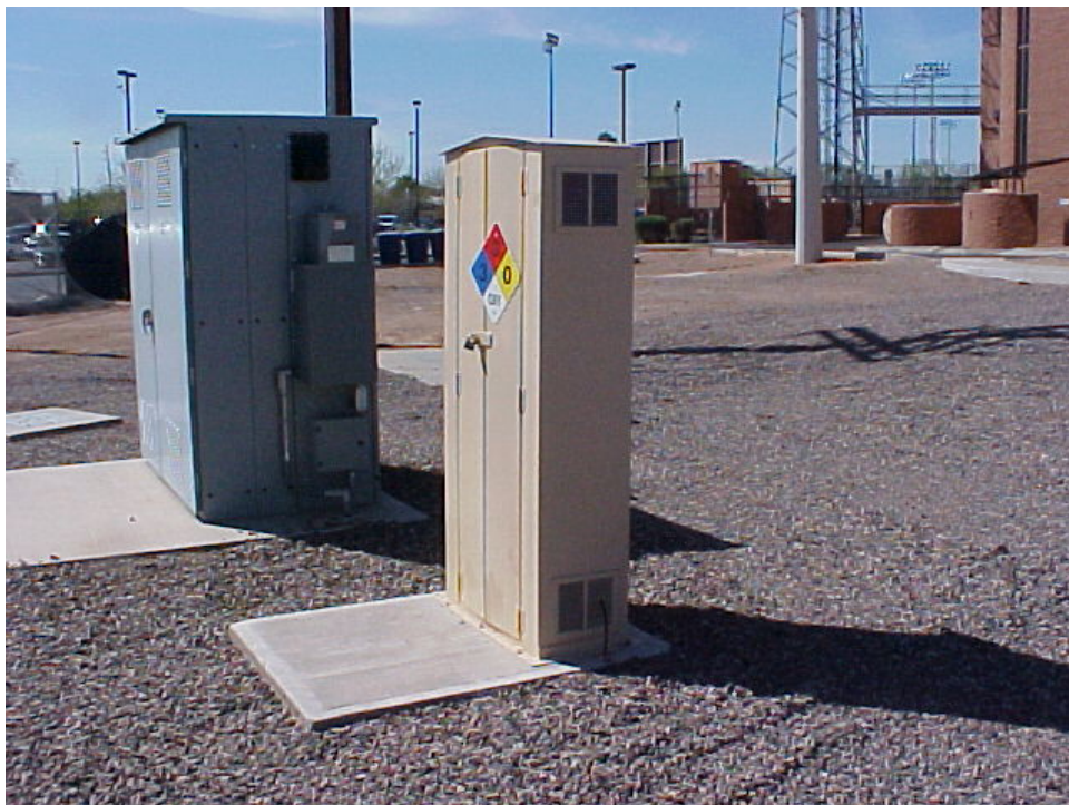
Chlorine storage room--notice the vents at the bottom and top. The bottom vent will allow the gas to ventilate because \text{Cl}_2 gas is heavier than air.
