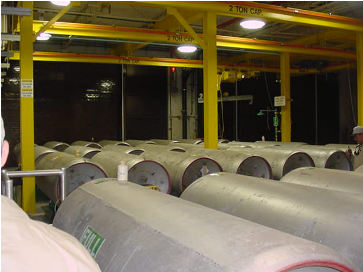
1 Ton Chlorine Containers.
