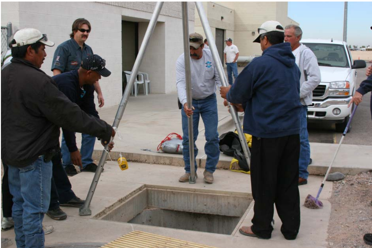
Confined space entry procedures and proper ventilation examples.
