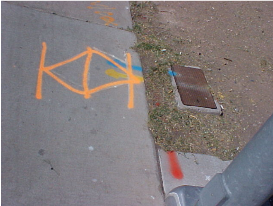
Red-Electricity, Yellow-Gas, Blue-Water
