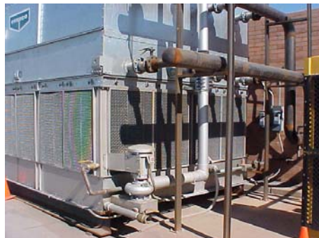
Cooling Tower - A common location of a cross-connection
