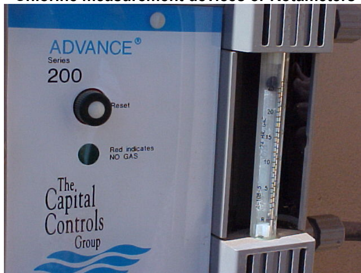
Chlorine measurement devices or Rotameters
