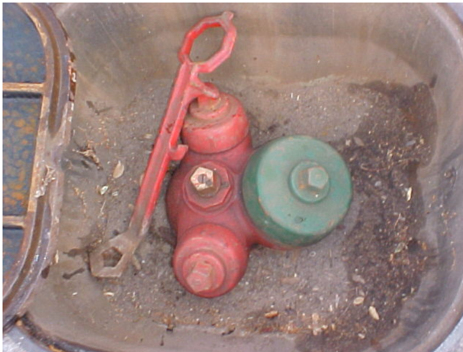
Airport Runway fire hydrant, hidden below the ground surface.
