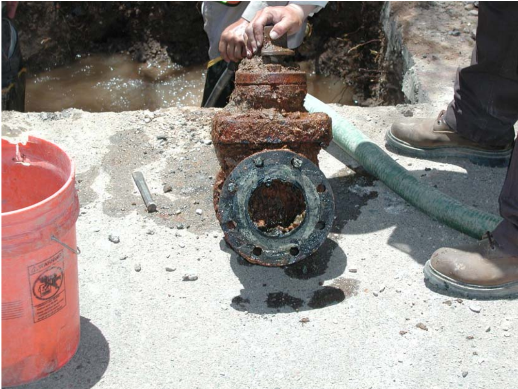
Broken closed Gate Valve with nasty tuberculation.
