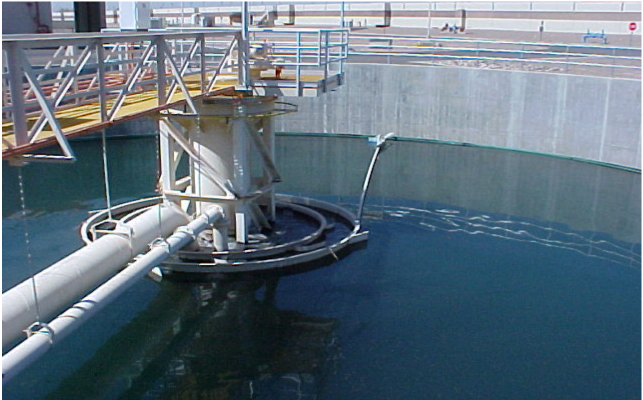
Circular clarifier and collector mechanism
