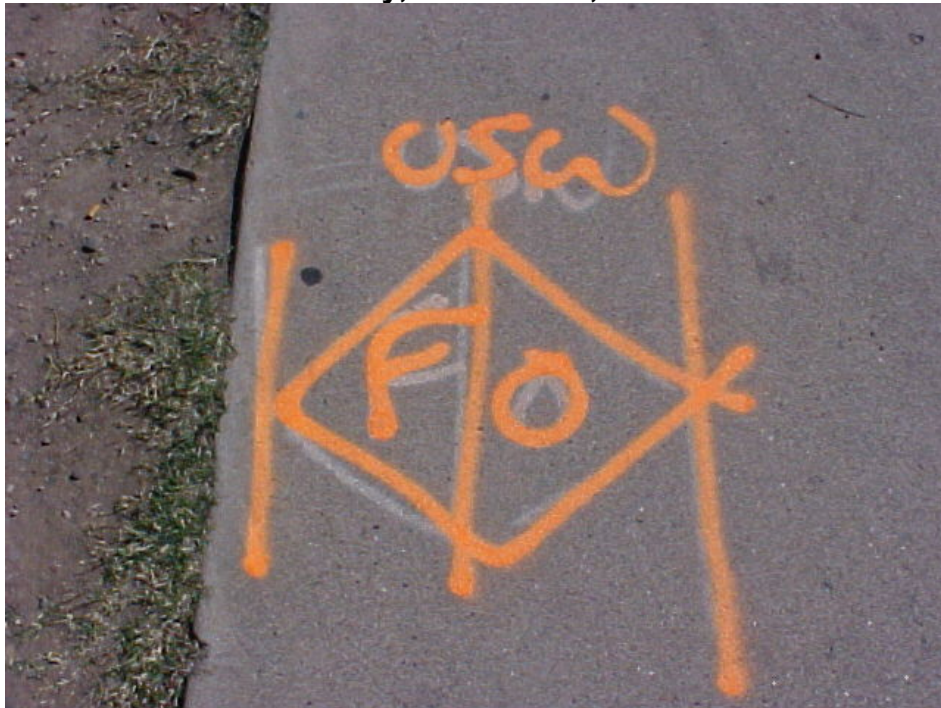
Orange-Telephone & Fiber Optics
