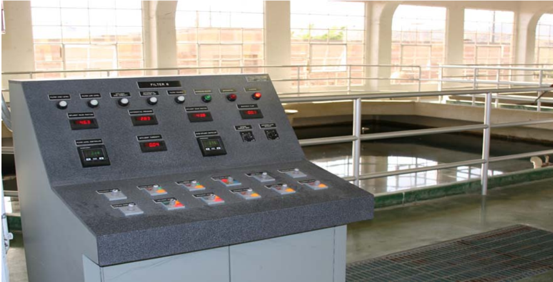
This is a filter control panel.
