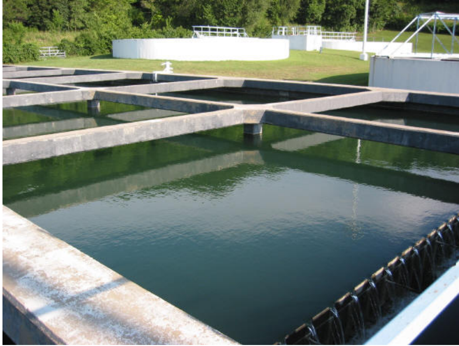
Top Picture - Final Rectangle Sedimentation Basin Bottom - Clarifier
