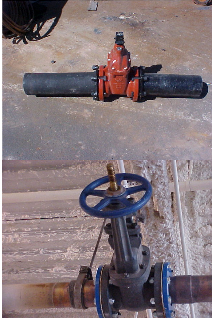
Different types of Gate Valves (Linear)
