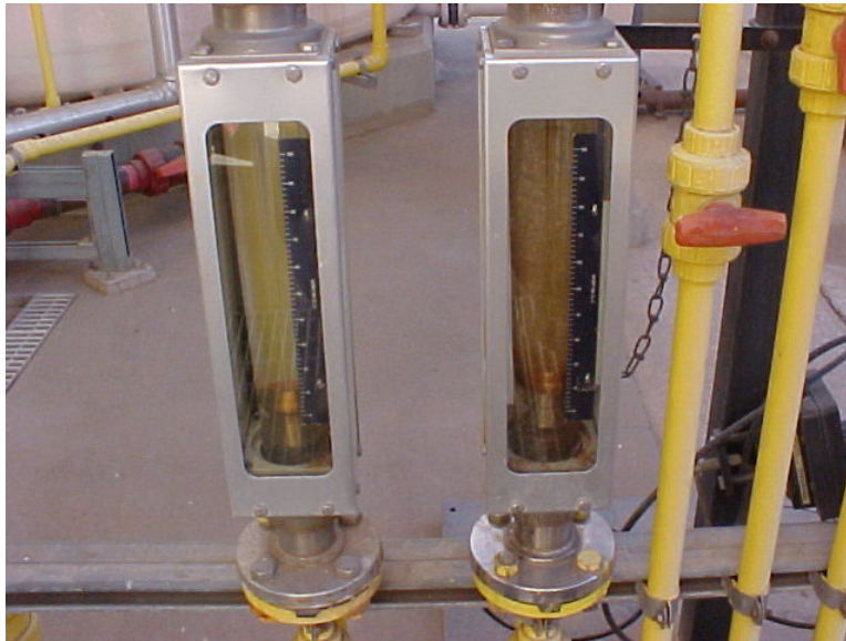
Chlorine measurement devices or Rotameters
