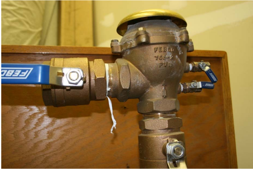
PRESSURE VACUUM BREAKER ASSEMBLY
