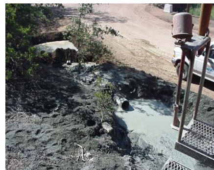
Constructed Mud Pits
