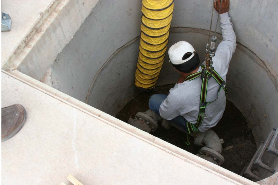
Entering a confined space with proper ventilation.
