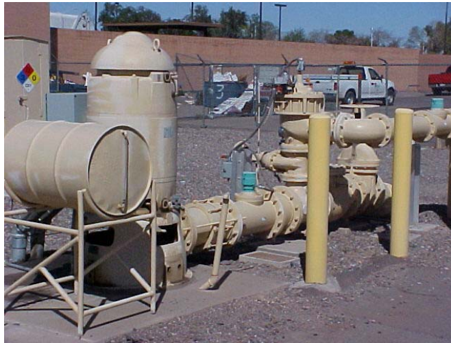
Well with a mineral oil sealed vertical turbine pump.
