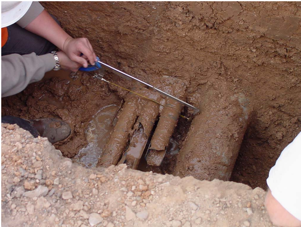
Service worker cutting abandoned utility conduit out of the way. Always call first and get the utility to show up to verify if you are able to cut an abandoned utility. I personally do not trust anything the other utilities will say or put in writing.
