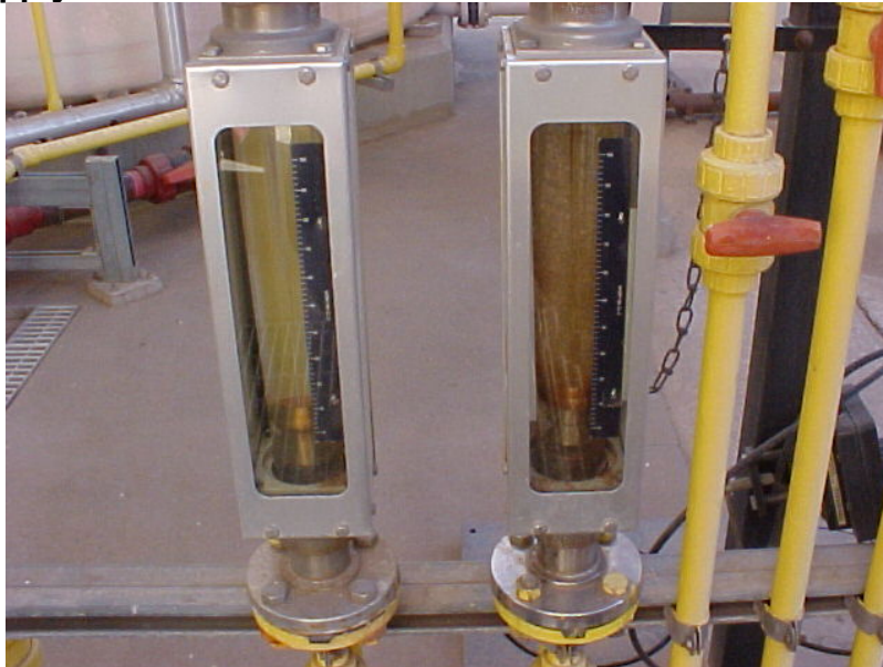
Chlorine measurement devices or Rotometers
