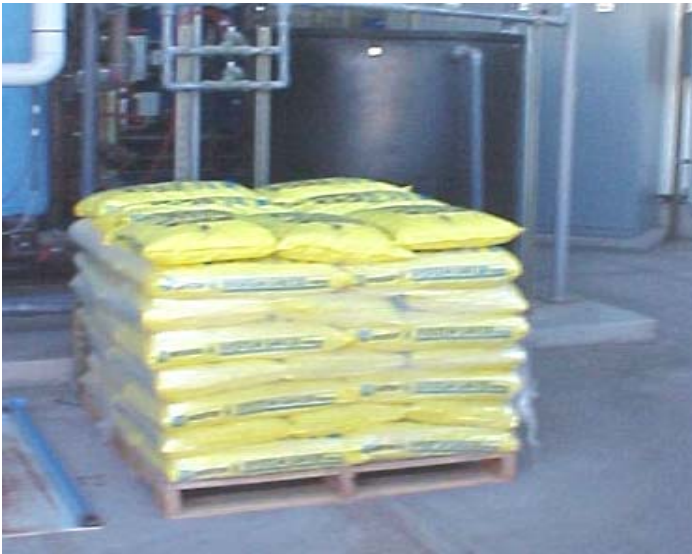
The container behind the salt pallet is a high concentration of salt and water. (Brine)
