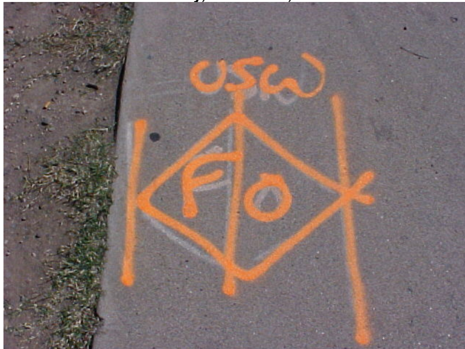
Orange - Telephone & Fiber Optics
