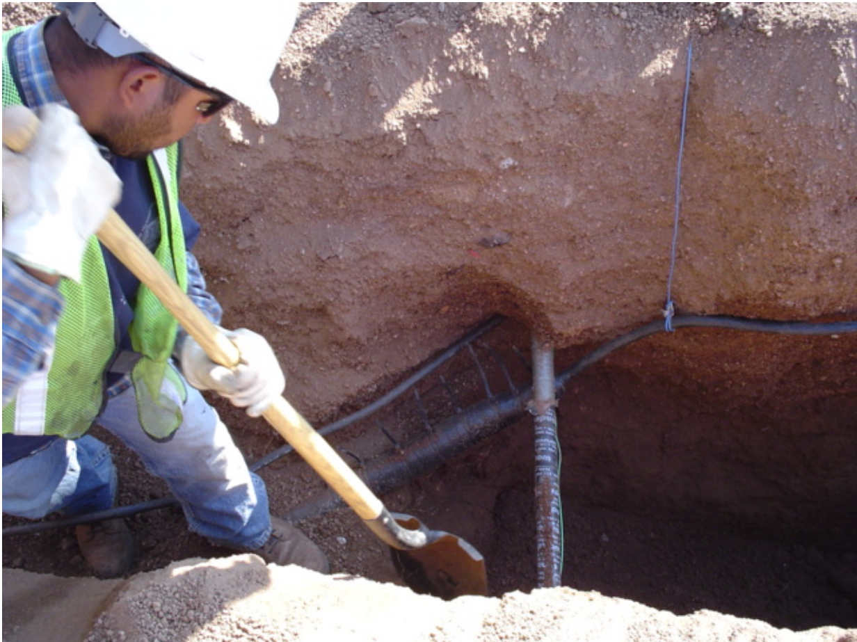
Buried telephone cables
