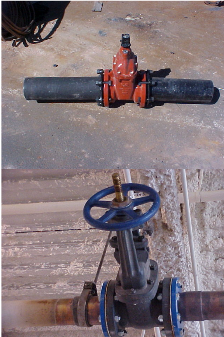
Two different styles of Gate Valves
