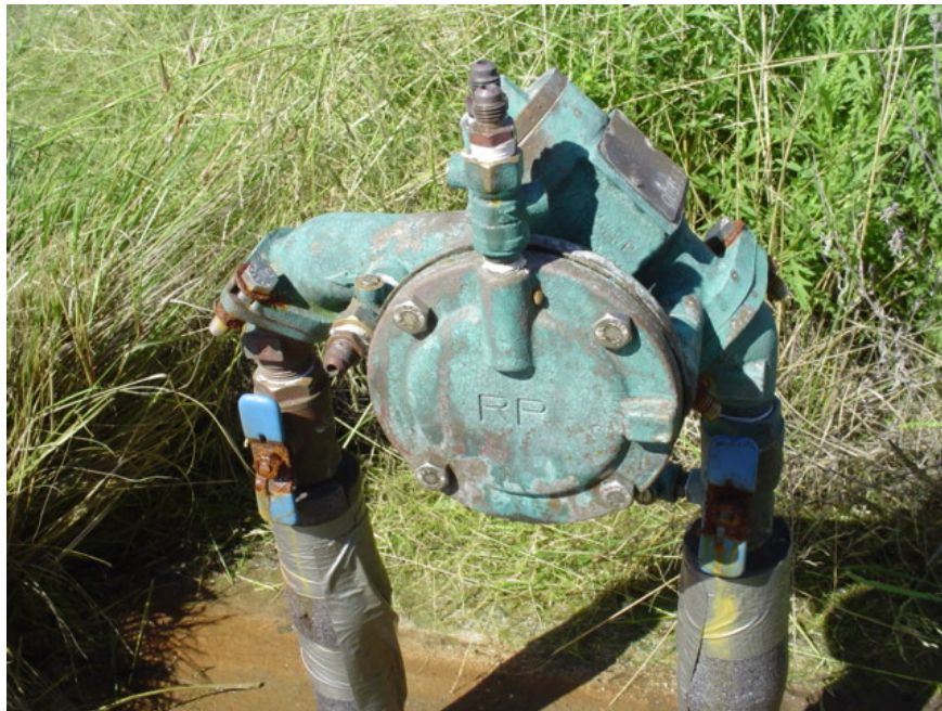
Various Reduced Pressure Principle Backflow Assemblies.
