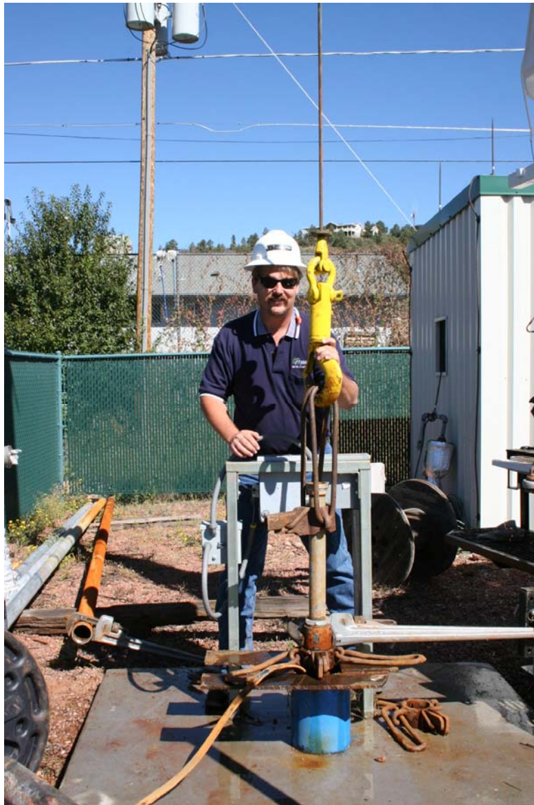
Removing the well casing from a groundwater well.
