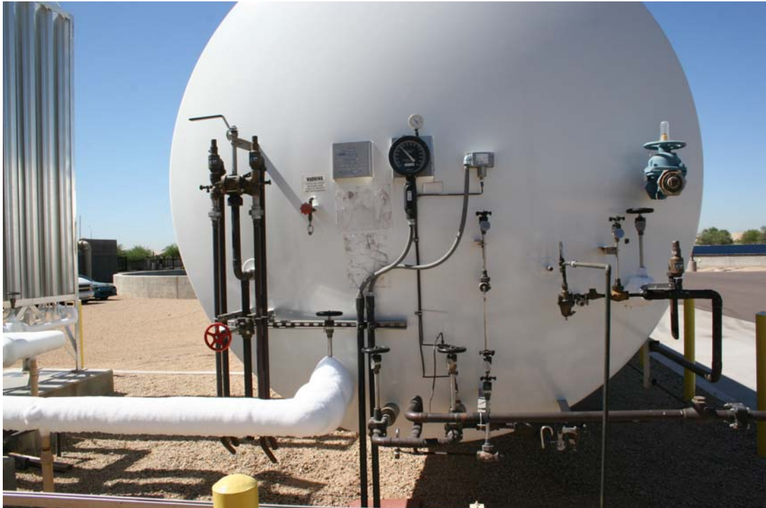
Ozone generator and Oxygen storage tank
