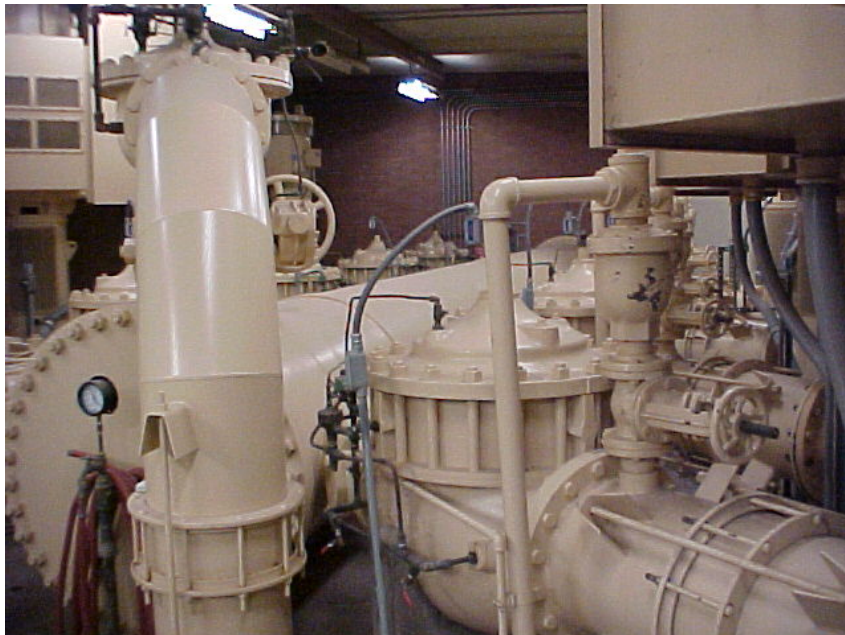
The inside of a booster pump station, notice the PRV and air relief valve.
