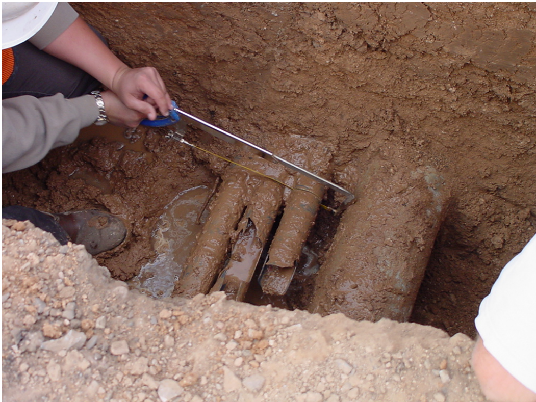
Service worker cutting abandoned utility conduit out of the way.
