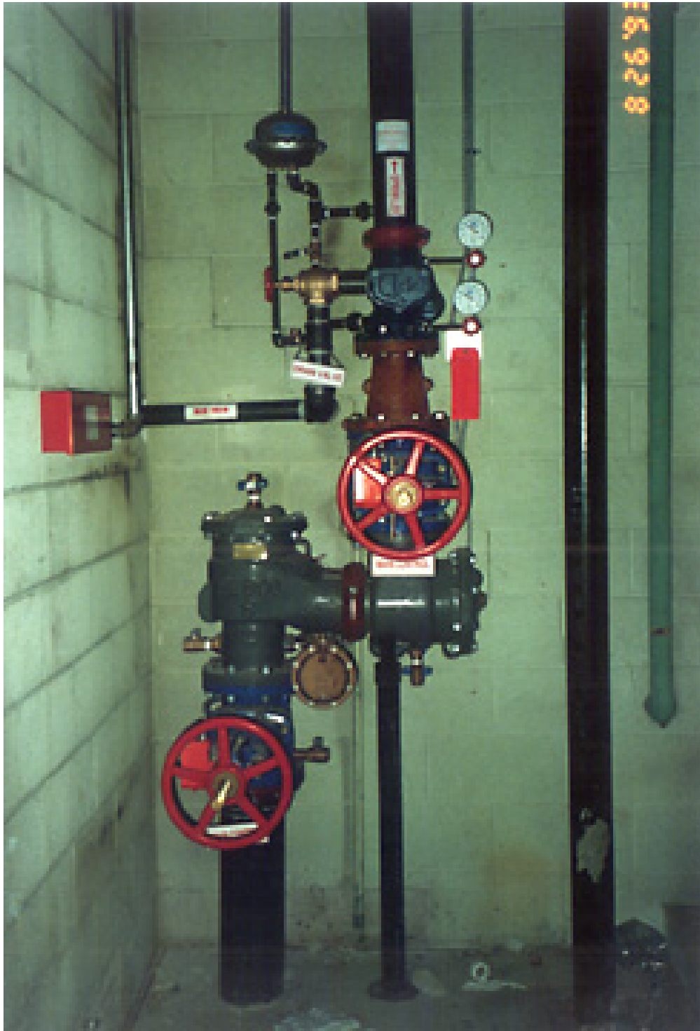
Reduced Pressure Backflow Assembly on a fireline
