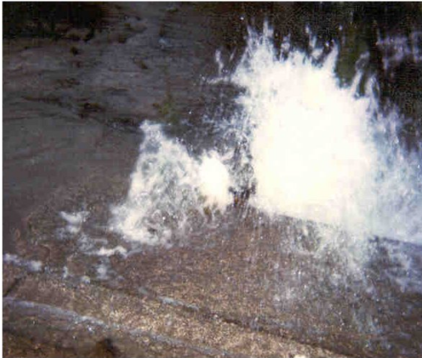
Broken Water Service
