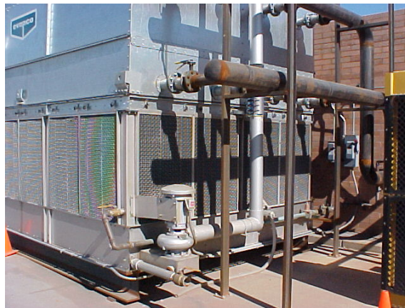
Cooling Tower A common location of a cross-connection
