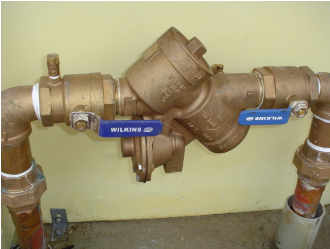
Various Reduced Pressure Principle Backflow Assemblies.
