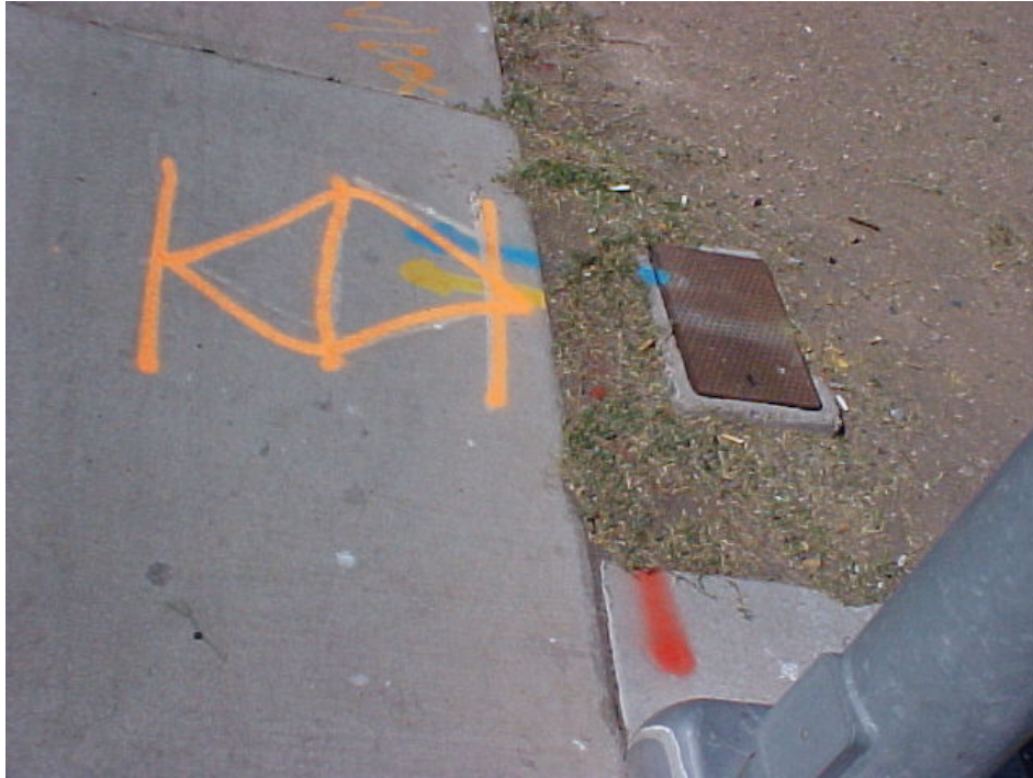
Red-Electricity, Yellow-Gas, Blue-Water
