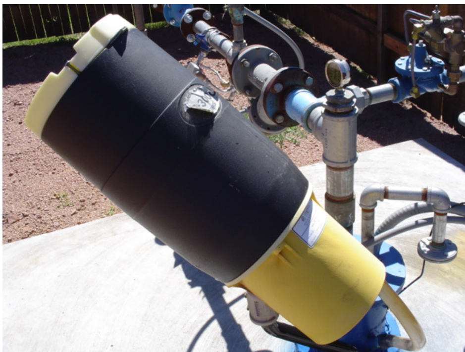
150 pound chlorine gas cylinder. Always tag the empty cylinder and store upright. Bottom, this is a dry chlorine tablet or HTH feeder.
