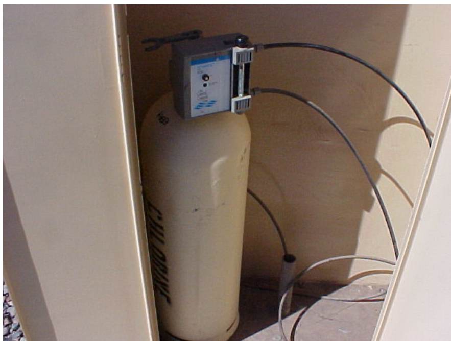
150 pound chlorine gas cylinder. Always tag the empty cylinder and store upright. Bottom, this is a dry chlorine tablet or HTH feeder.
