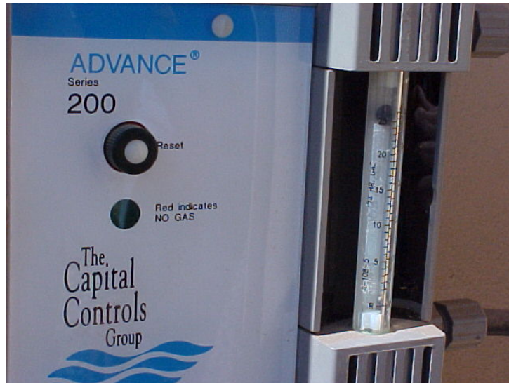
Chlorine measurement devices or Rotameters
