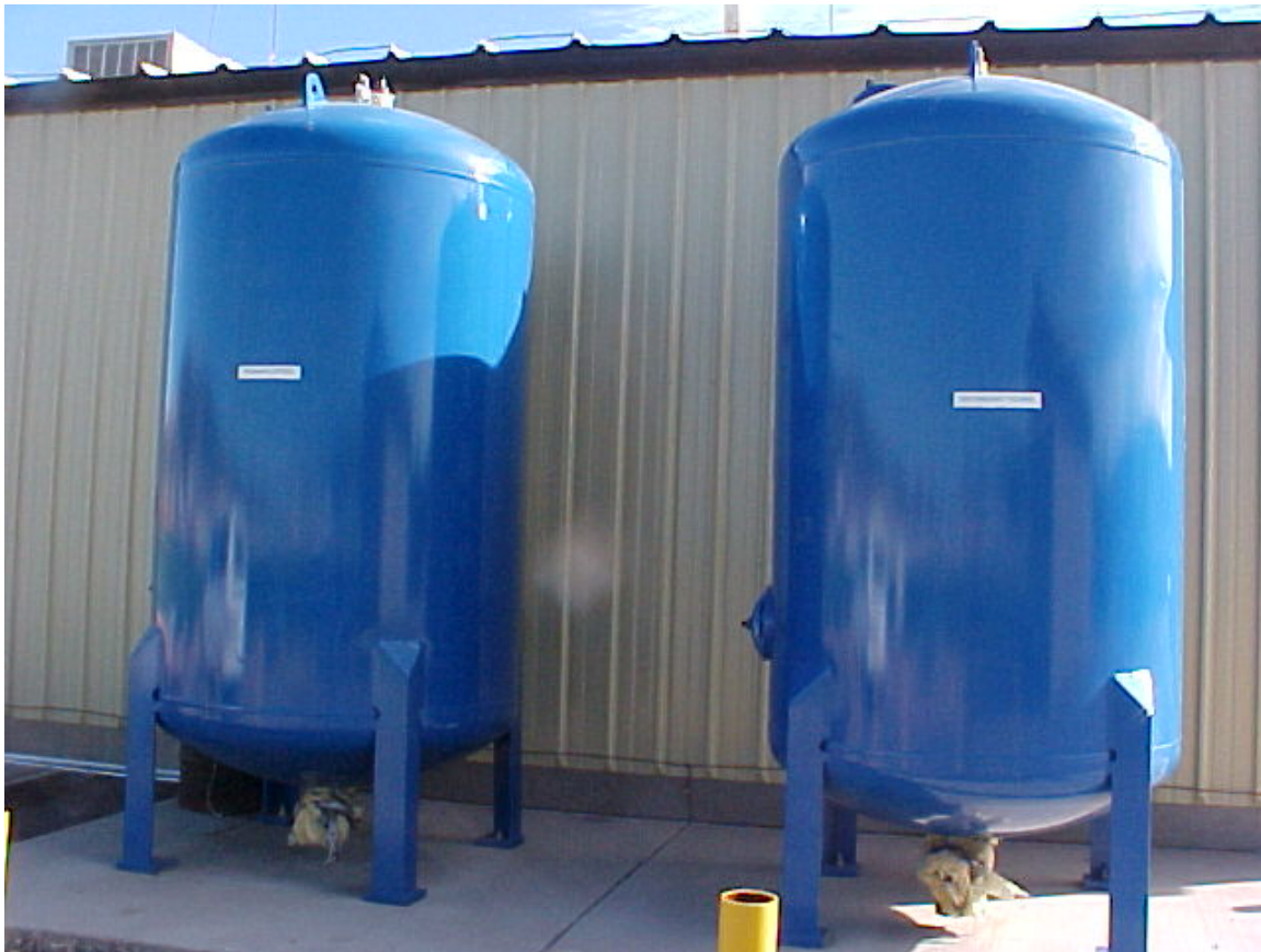
Carbon Vessels used to remove tastes and odors from water.
