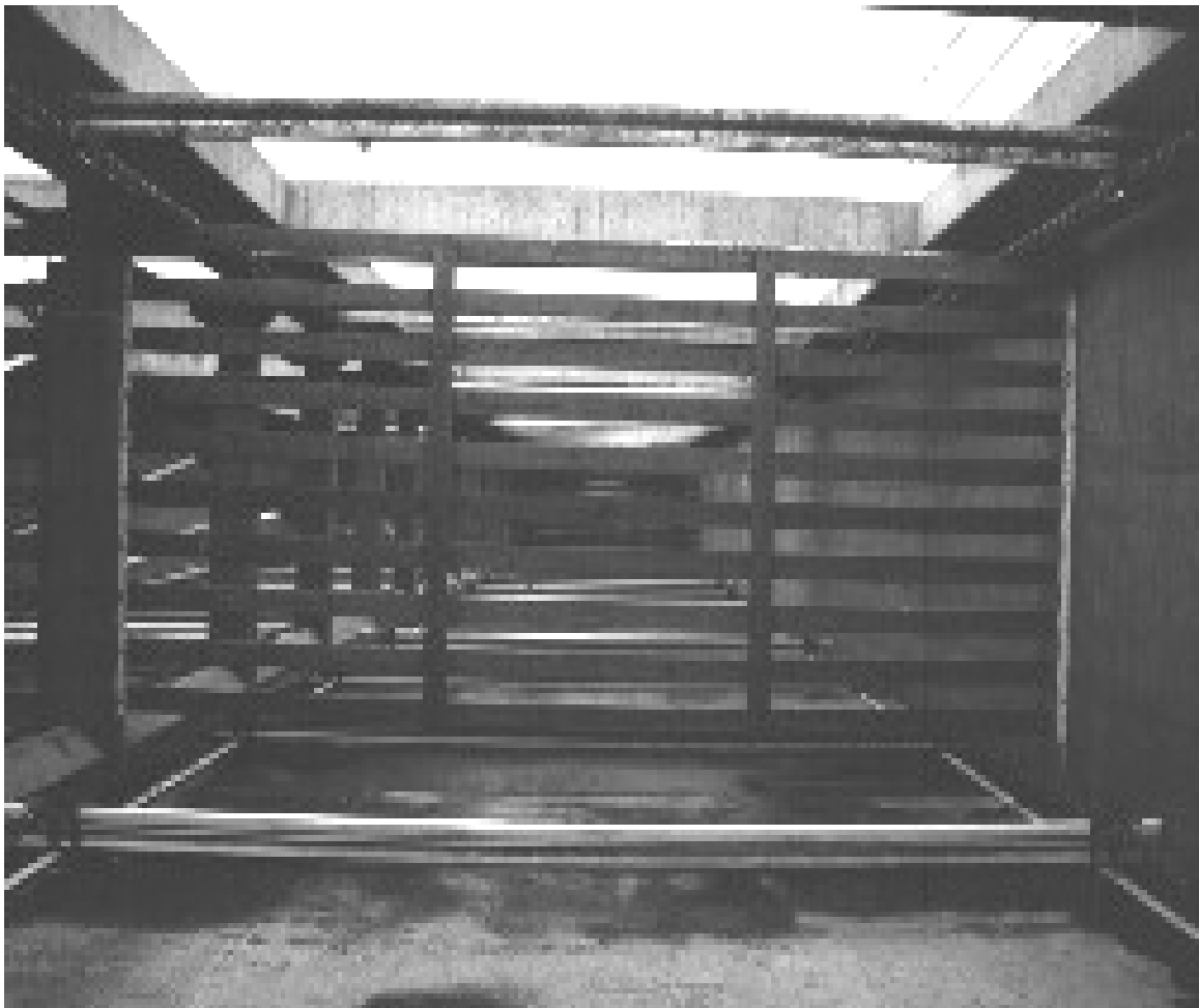
Rectangular basin flights and chains
