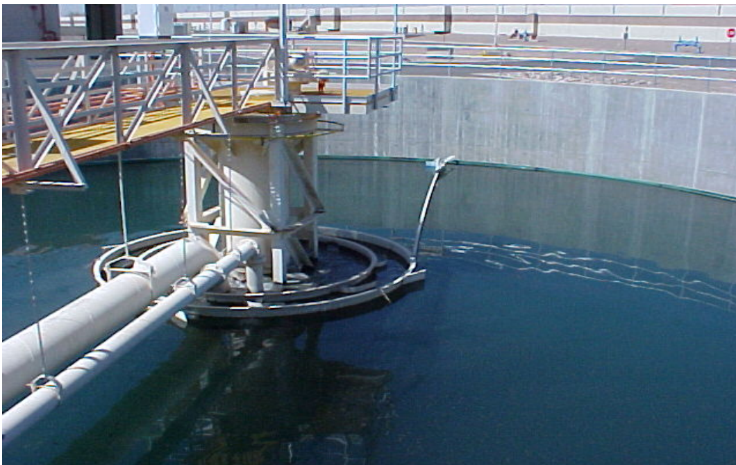
Circular clarifier and collector mechanism
