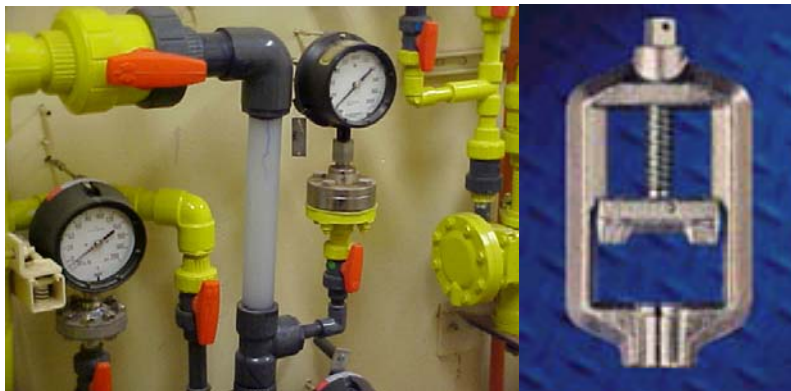
Chlorine Piping and chlorine cylinder yoke
