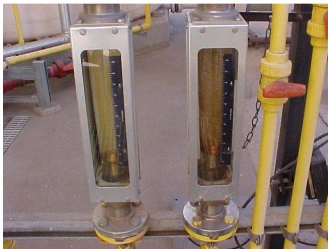
Chlorine measurement devices or Rotameters.
