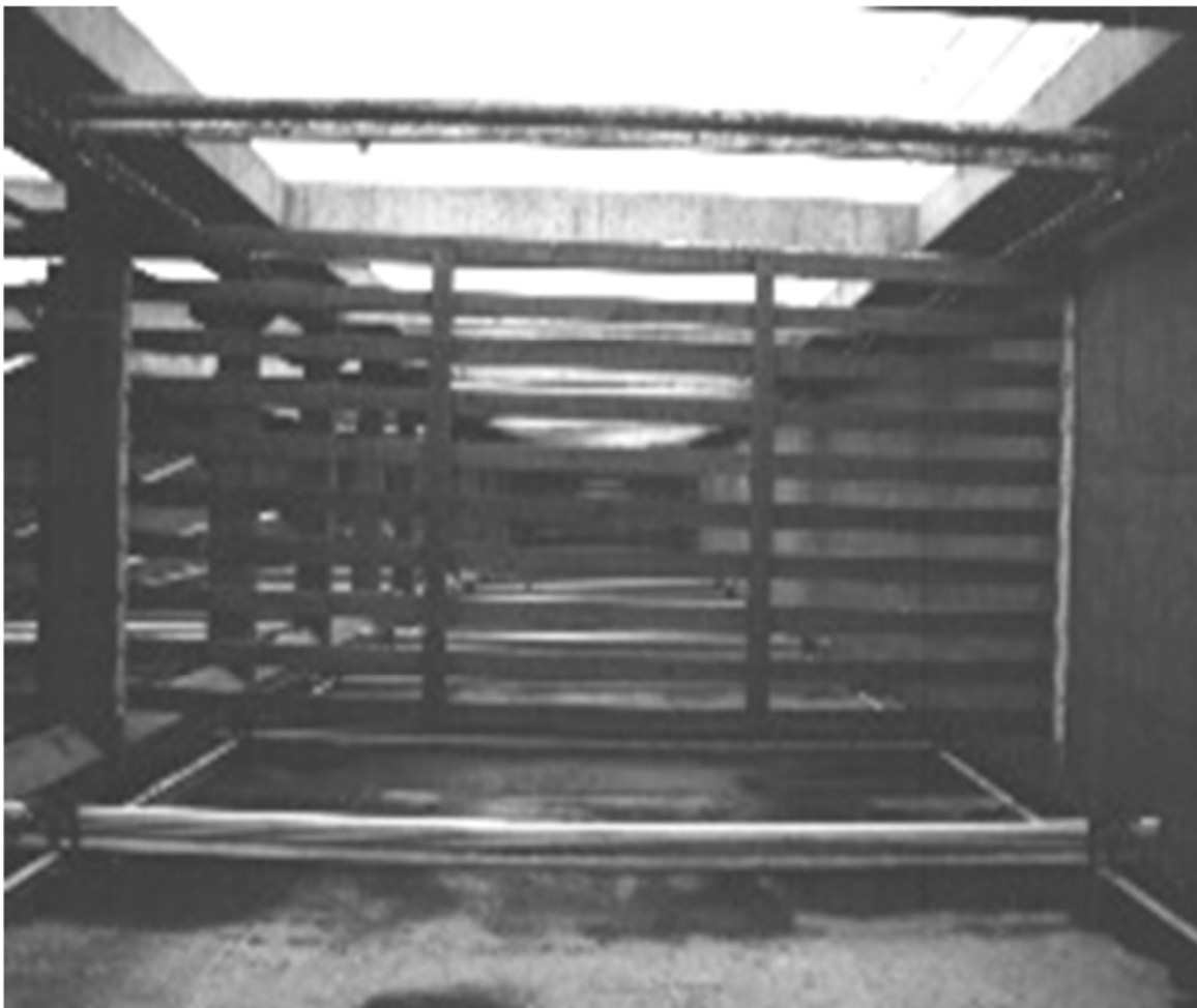
Rectangular basin flights and chains.
