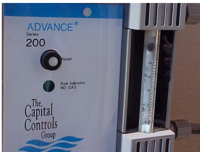
Chlorine measurement devices or Rotameters.
