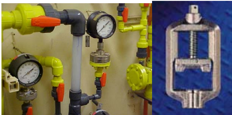
Chlorine piping and chlorine cylinder yoke.
