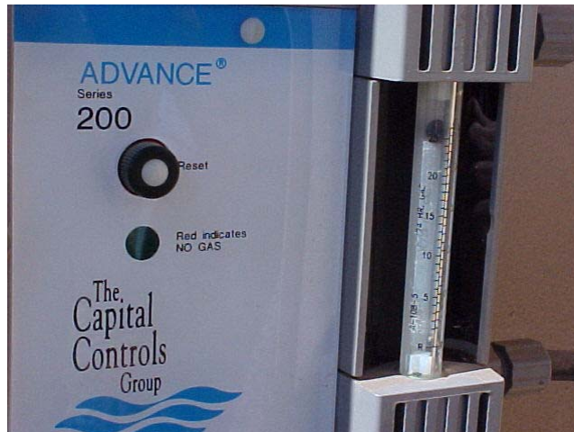
Chlorine measurement devices or Rotometers.
