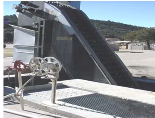
Manual and Mechanical Bar Screens
