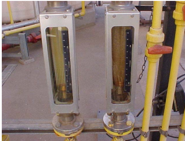
Chlorine measurement devices or Rotometers.
