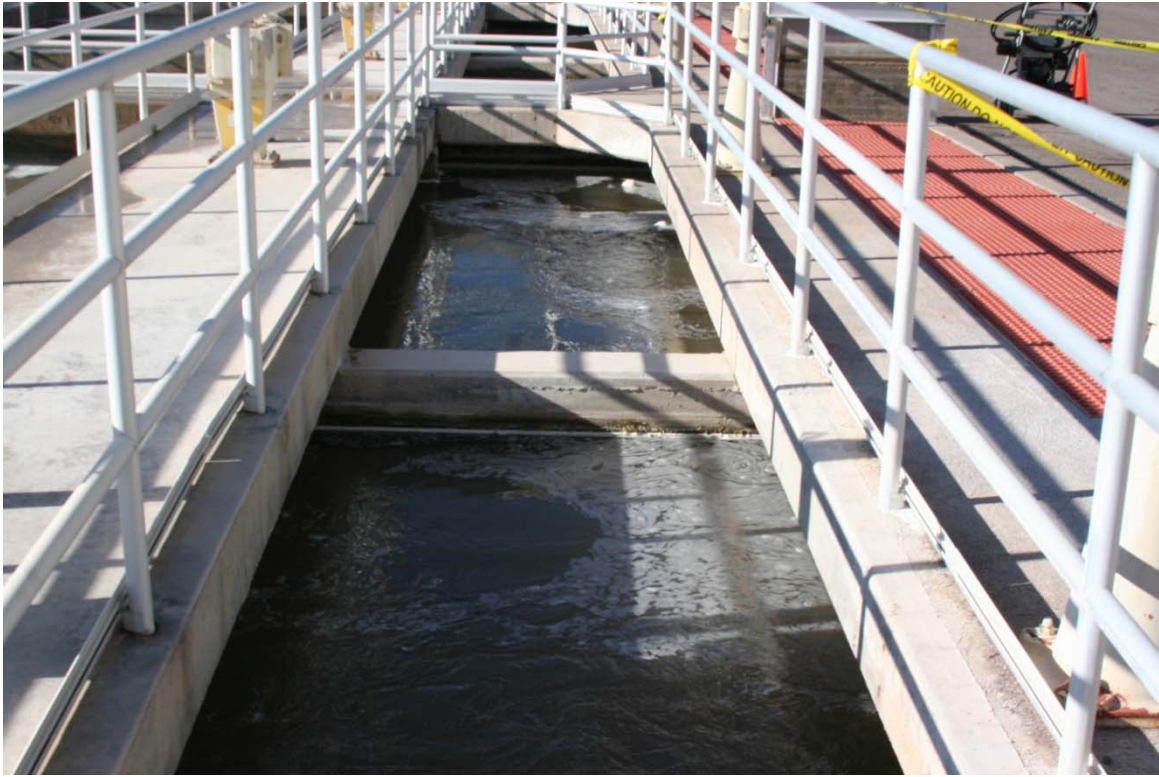
Top- Compartment style Flocculation Basins Bottom – Filter backwash draining filter
