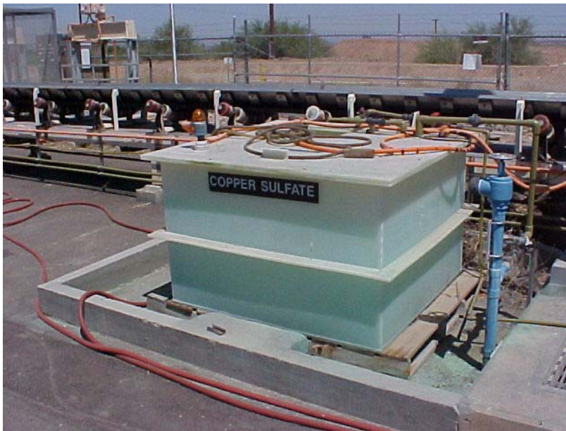
Examples of different types of chemical storage tanks found in water treatment facilities.
