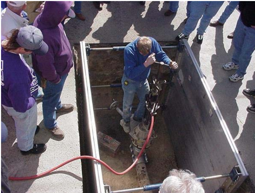
Hydro Stop valve insertion machine
