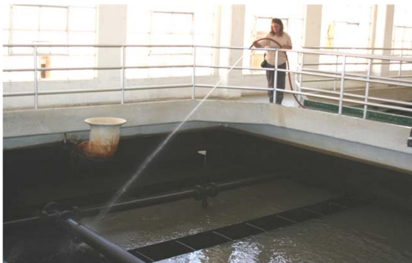
Filter aid being fed at the weirs of sedimentation.
