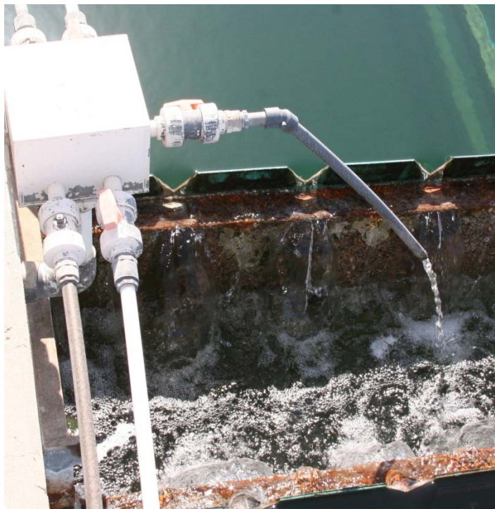
Filter aid being fed at the weirs of sedimentation.
