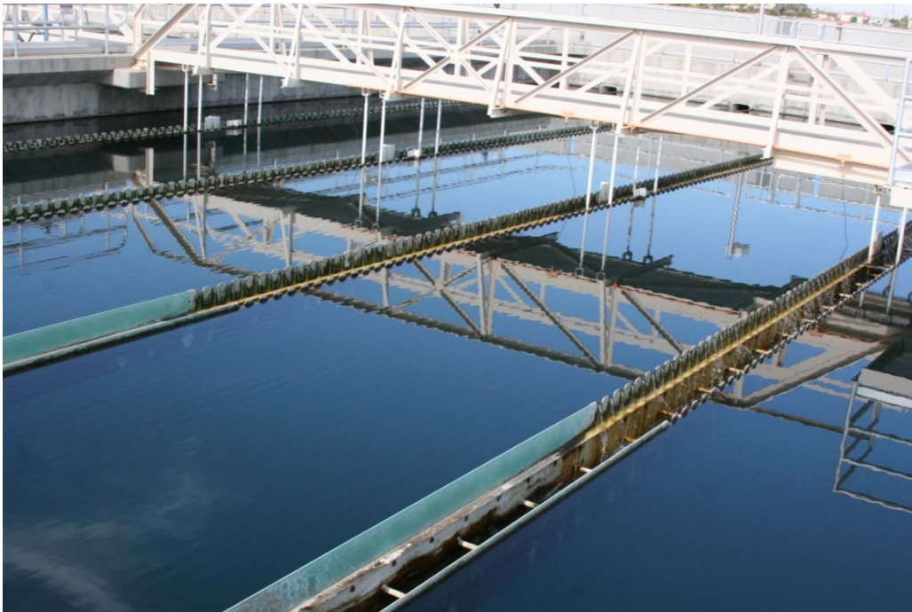
Top- Baffles for slowing water down prior to settling. Bottom- Rectangular sedimentation basins
