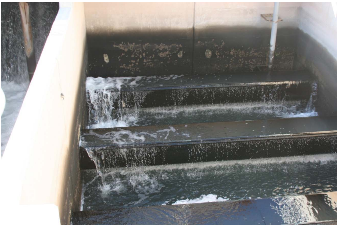
Top- Compartment style Flocculation Basins Bottom – Filter backwash draining filter
