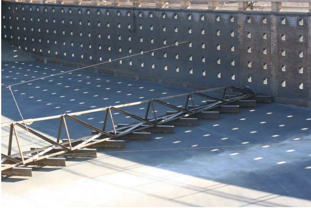
Top- Baffles for slowing water down prior to settling. Bottom- Rectangular sedimentation basins
