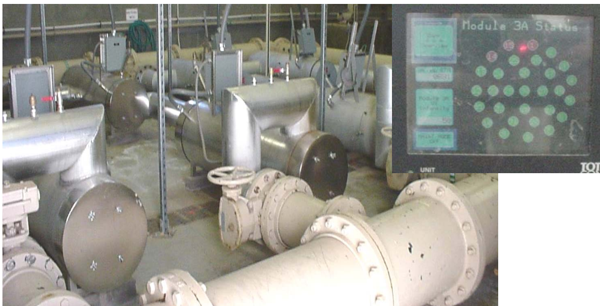
UV Trains and SCADA display
