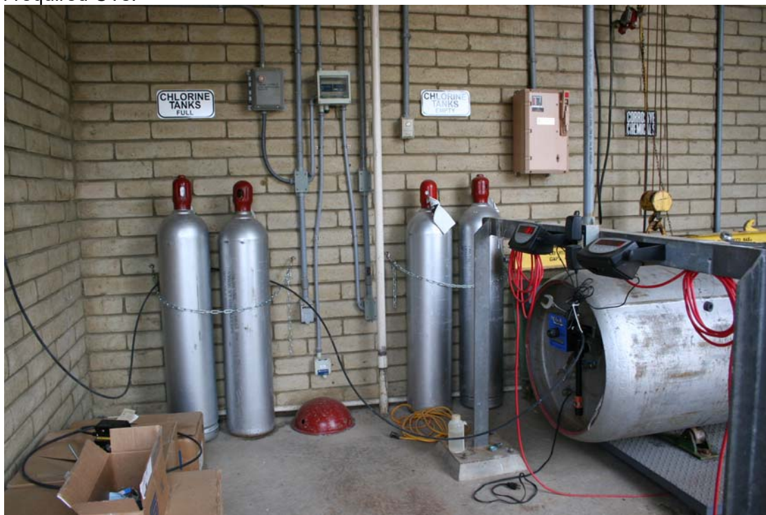
500 pound container and 150 pound cylinders. The 1/2 ton is on a scale. Cylinders stand up right and containers on their sides.
