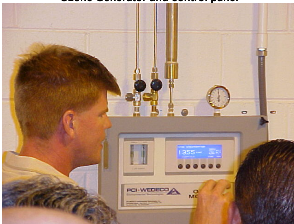
Ozone Generator and control panel
