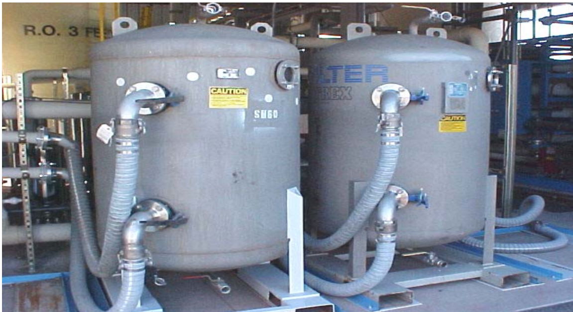
These containers hold the resin for the deionization
