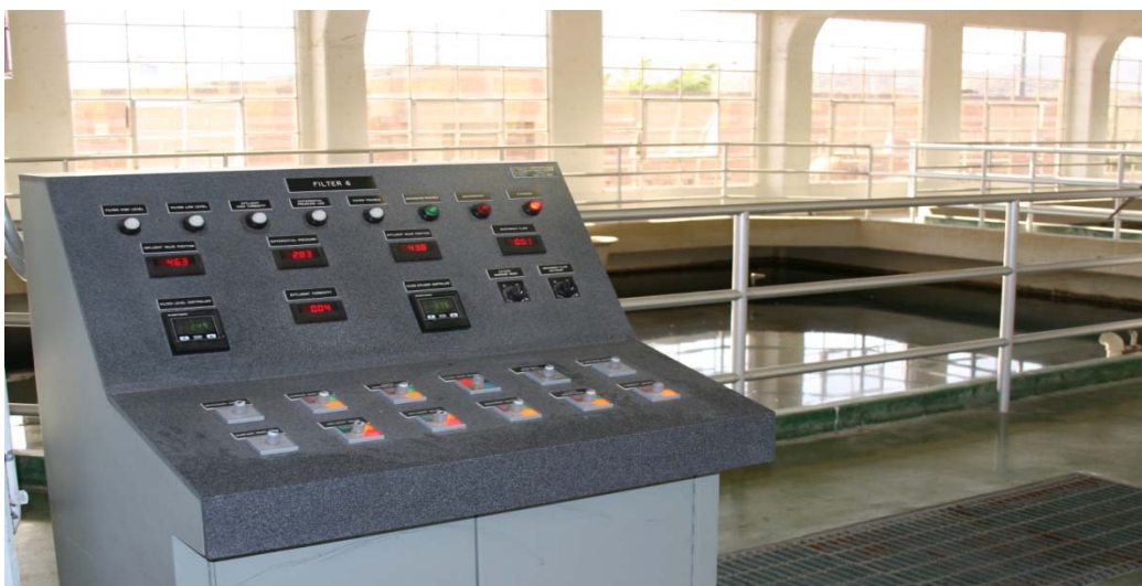
This is a water treatment filter control panel.
