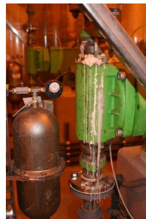
These photographs show an Alum leak. When exposed to air, this chemical becomes crystallized.
