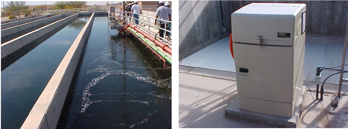
De-chlorination channel and automatic sampler.
