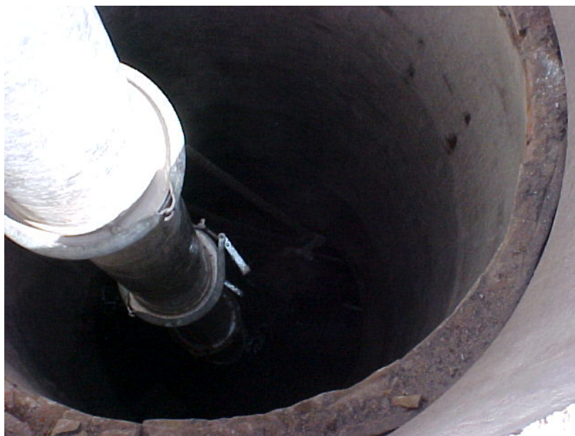
A Vactor clearing a Manhole
