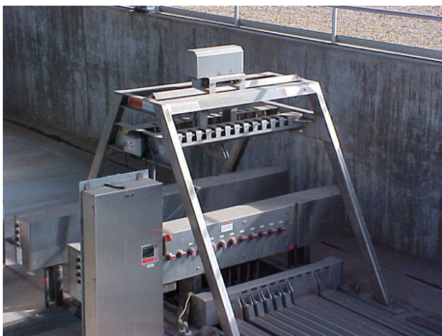
UV light generator and the actual UV light.
