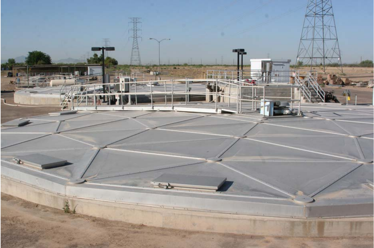
Covered wastewater basins to prevent or control odors.
