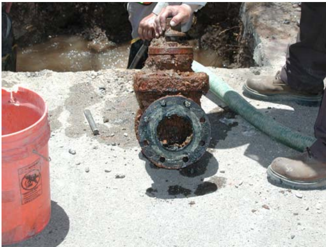
Broken gate valve with Tuberculation
