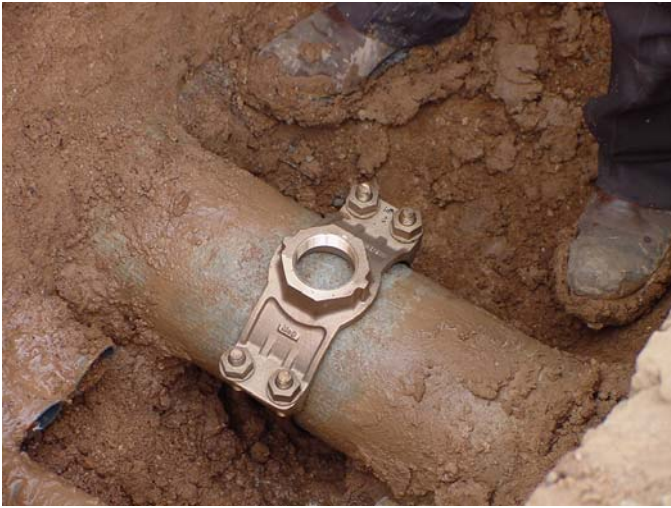
Installation of a new water service line.
