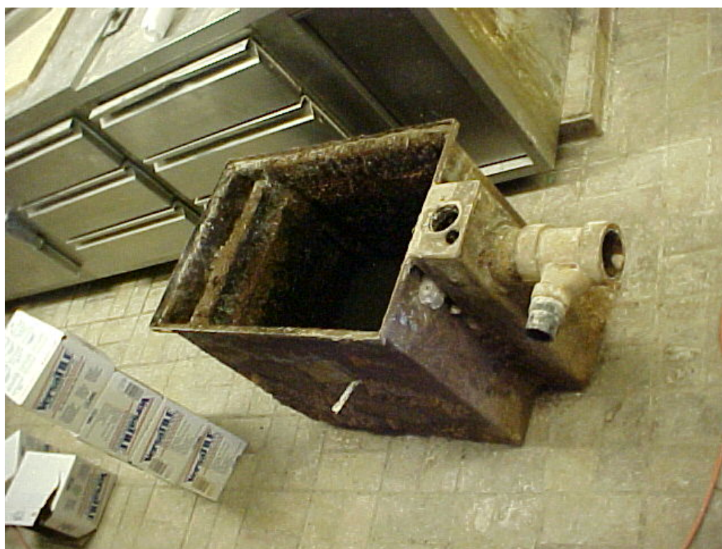
Common and worn out kitchen Grease Trap
