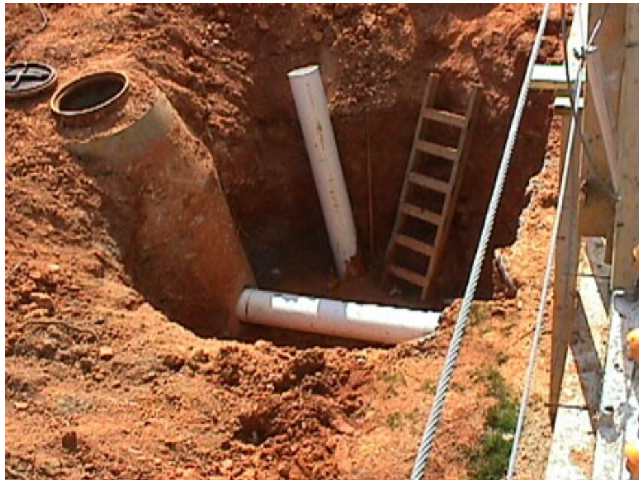
Sewer lateral going into a manhole.
