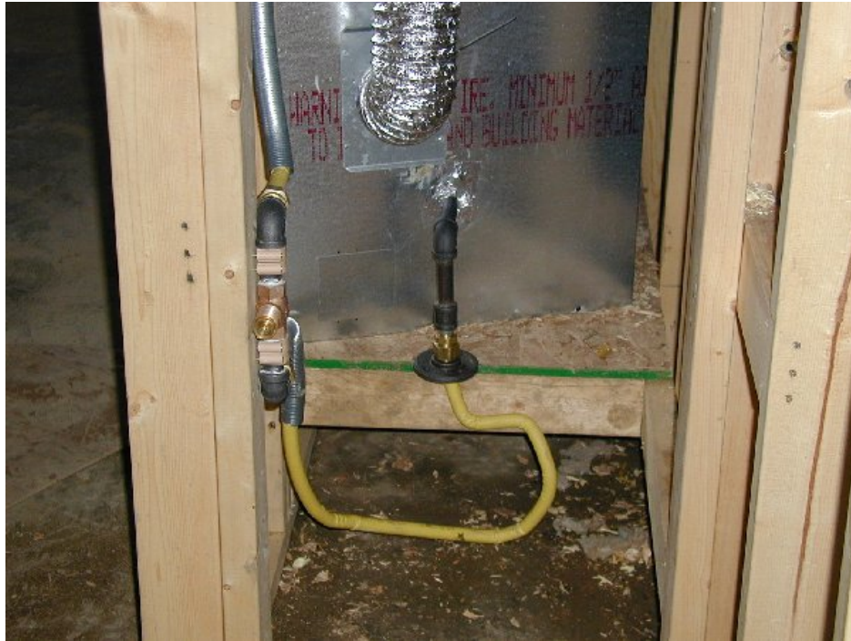
Gas manifold and connector to a fireplace
