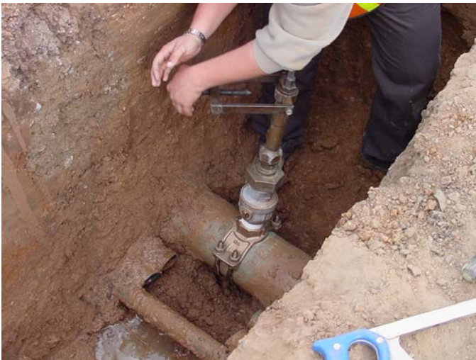
Installation of a new water service line.
