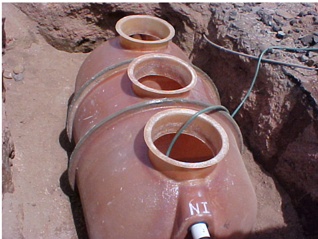
Three Compartment Grease Interceptor
