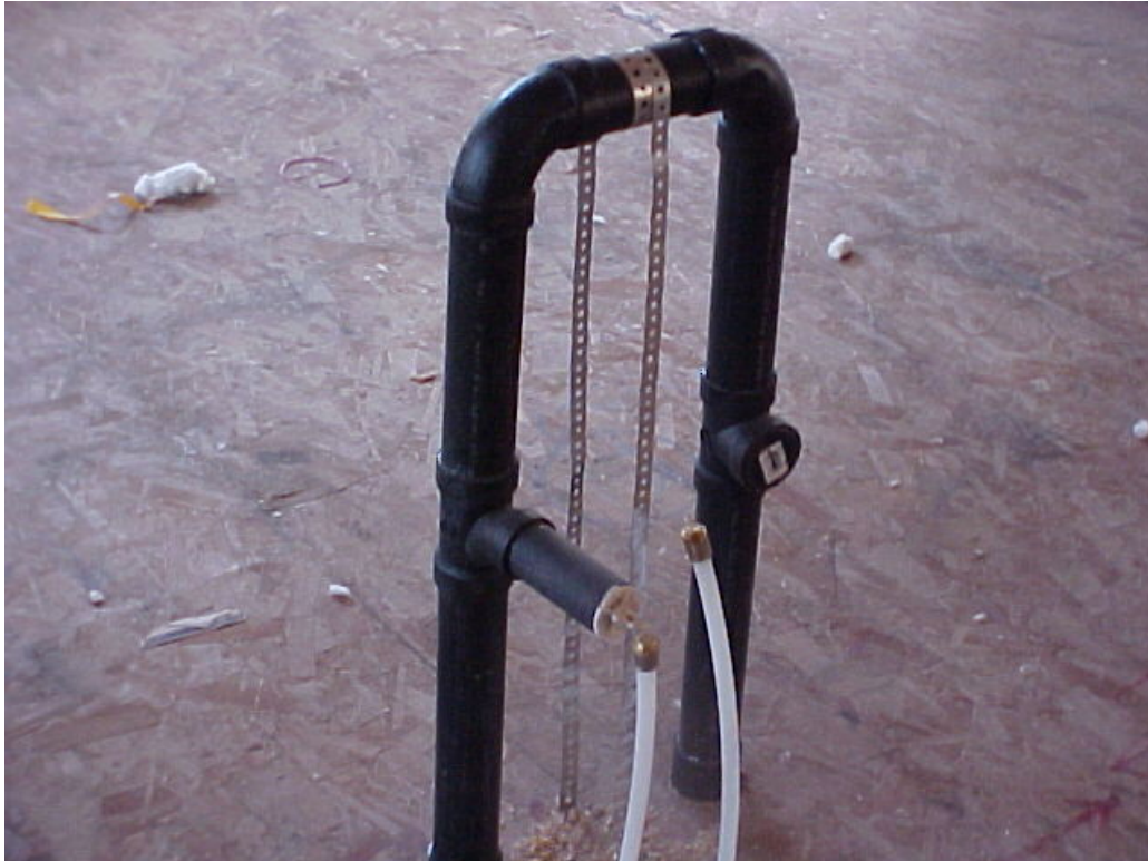
Combination waste and Vent system, Island Sink set-up 2 inch minimum vent The Foot Vent will go up the adjacent wall. Below, nail plate protection is necessary even for copper lines.
