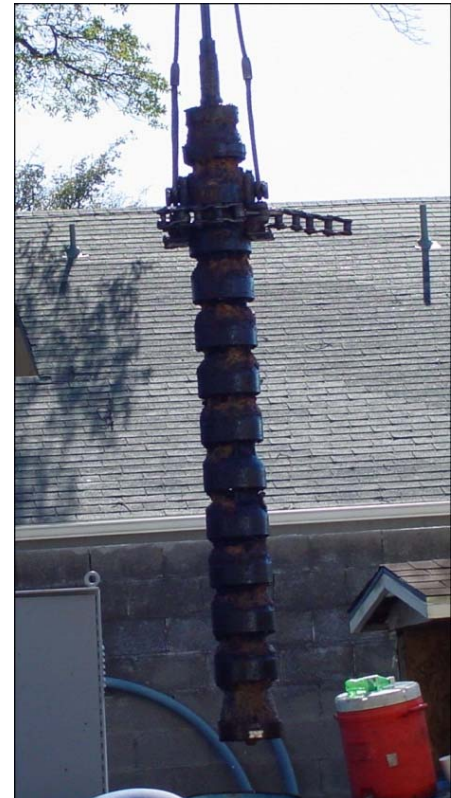
Above, Vertical Turbine Pump Being Removed (notice line shaft)
