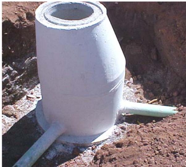
Grout is used to prevent infiltration into manholes.
