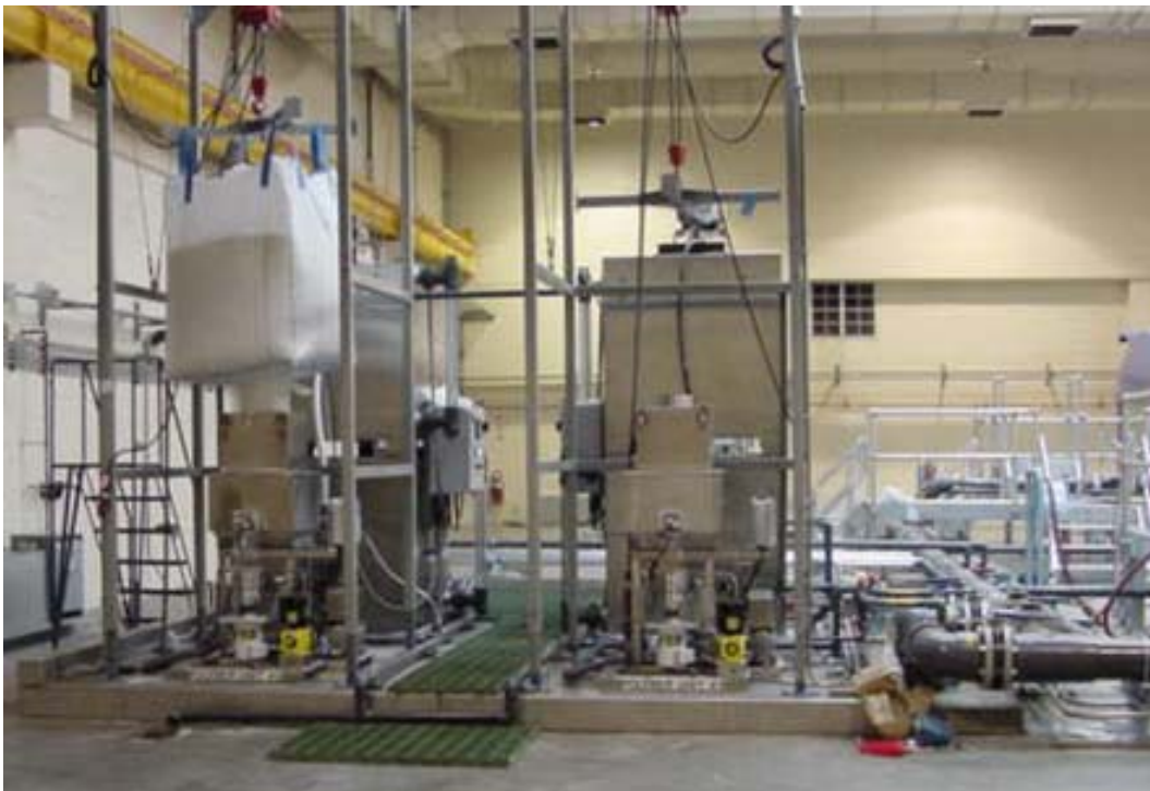
Dry polymer is being added and used for sludge thickening.
