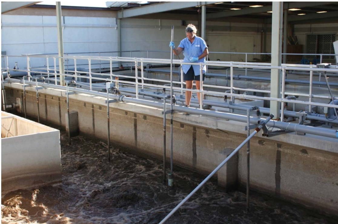
Both photographs show the aeration sequence for an SBR. Sequence Batch Reactor.
