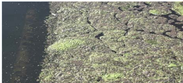
Algae on the Secondary clarifier, this is not a good sign.
