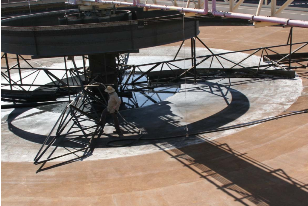
Scraping mechanism inside a clarifier.
