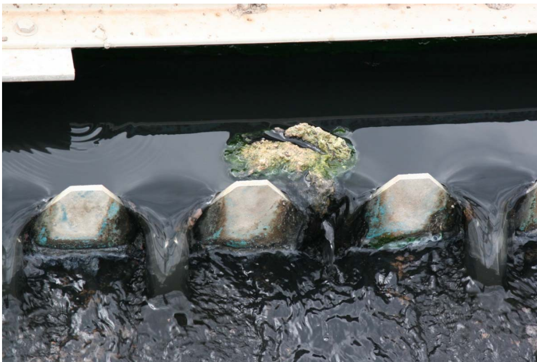
Caked grease stuck on weir.
