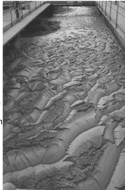
Figure 6. A heavy build-up of trapped Microthrix parvicella foam during winter.
