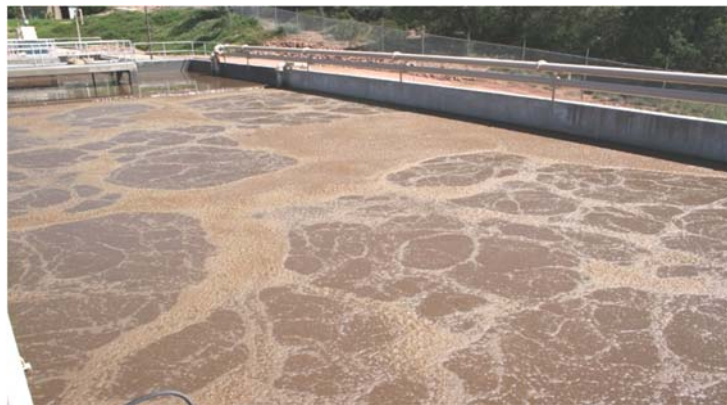
The above photograph shows air being unevenly distributed.
