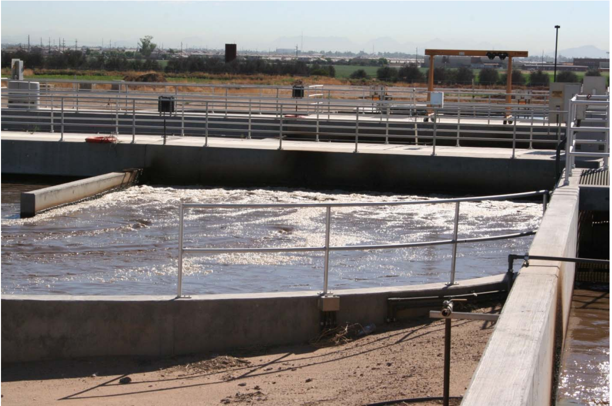
Oxidation ditches are used for nutrient removal.
