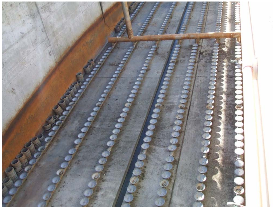
The same area from above photo, but clean and dry, these are porous air diffusers. A rare photo.
