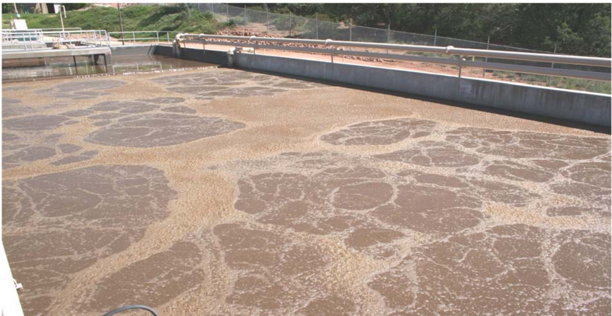
The above photograph shows air being unevenly distributed.
