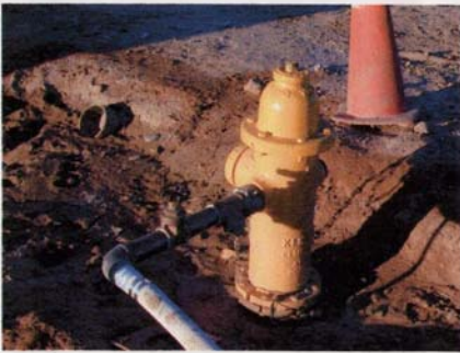
Fitting at hydrant
