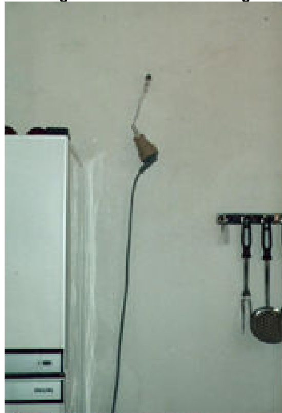
Dangerous Electrical Wiring
