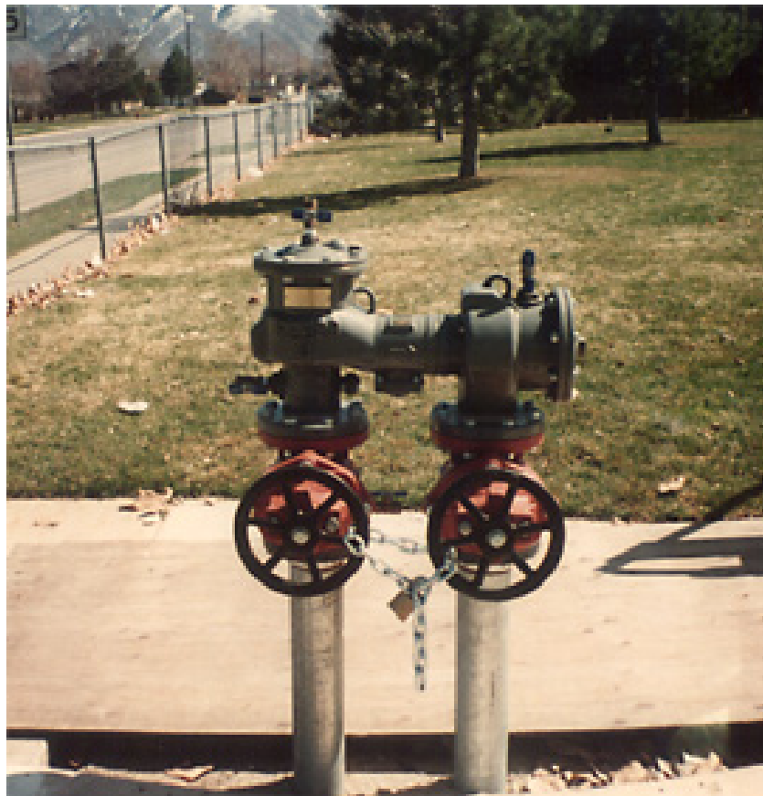
Double Check Backflow Assembly (Notice chain)
