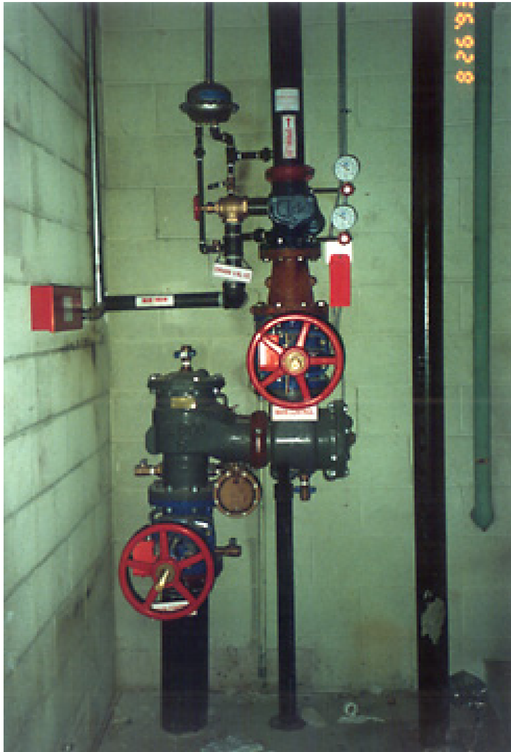
Reduced Pressure Backflow Assembly
