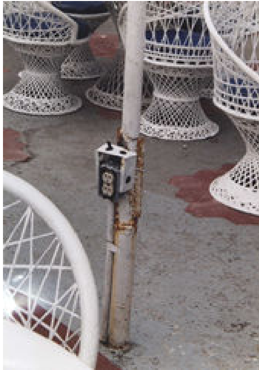
Dangerous Electrical Outlet
