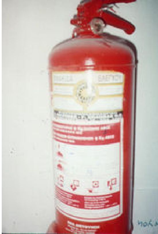
Fire Extinguisher without a discharge hose
