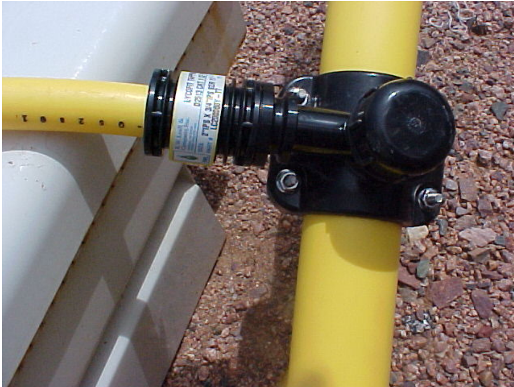
2 x \frac{3}{4} inch mechanical service tap
