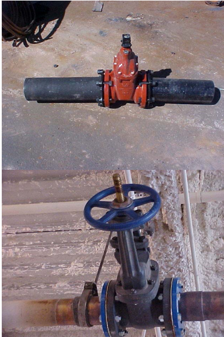
Two different styles of Gate Valves.
