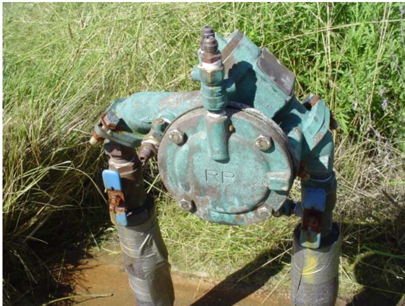
Various Reduced Pressure Principle Backflow Assemblies.
