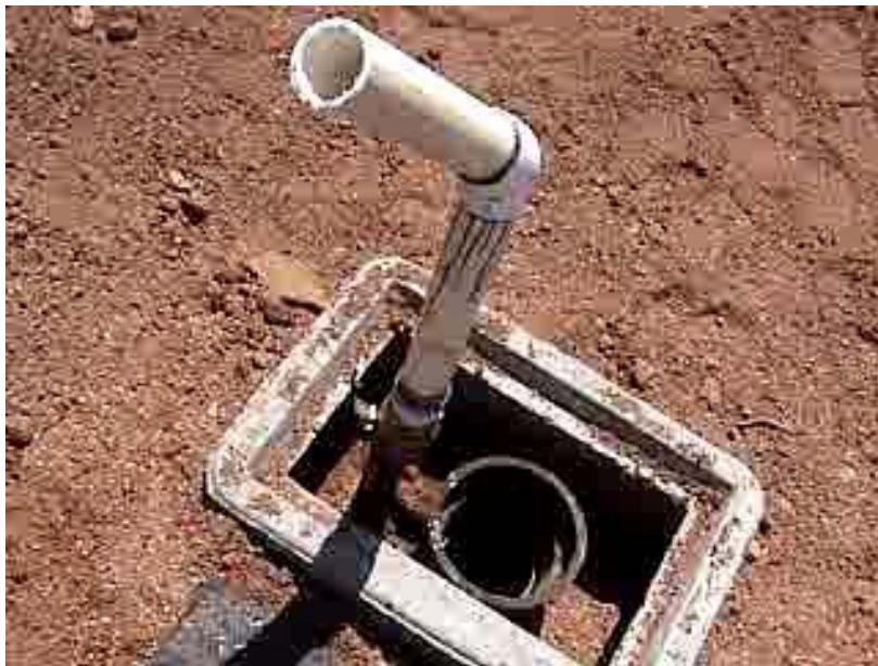
A temporary blow-off at a dead-end line.
