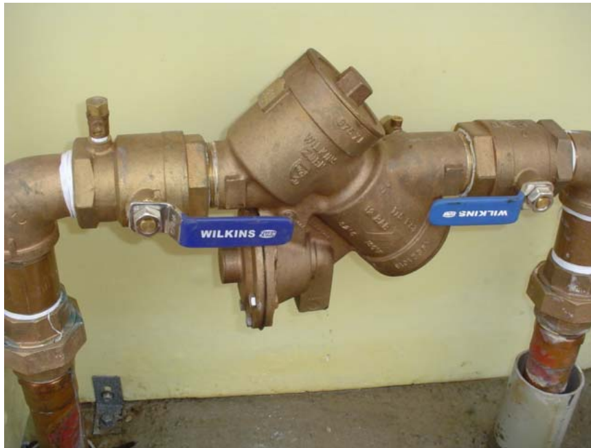
Various Reduced Pressure Principle Backflow Assemblies.
