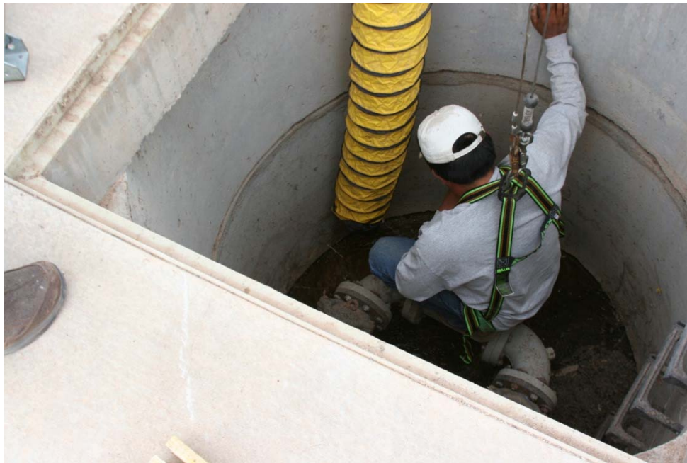
Entering a confined space with proper ventilation.
