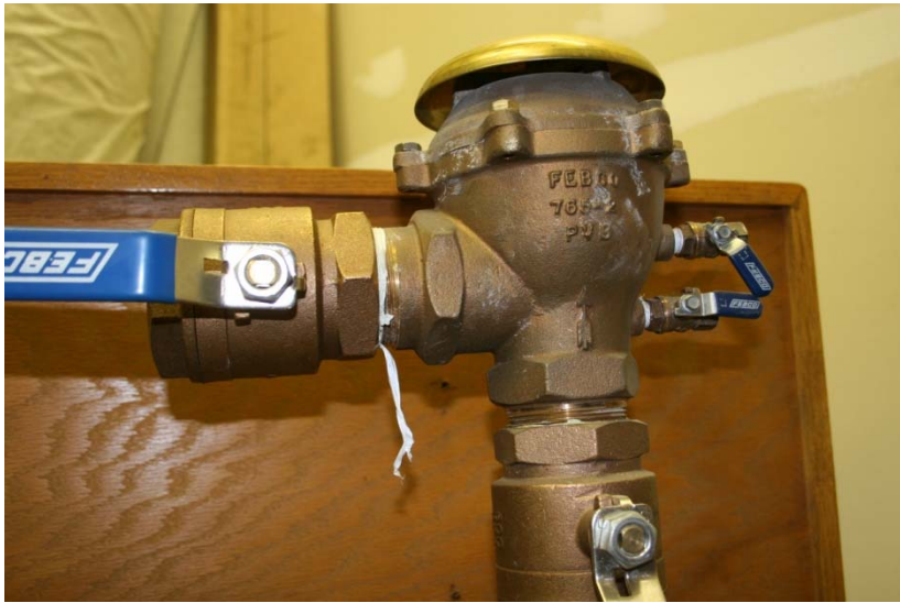
PRESSSURE VACUUM BREAKER ASSEMBLY
