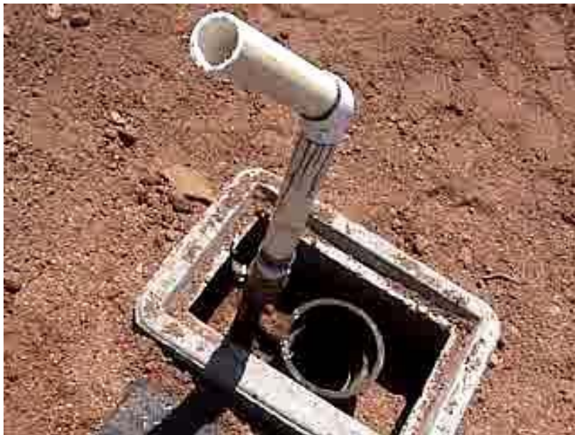
A temporary blow-off at a dead-end line.
