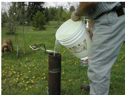
Pouring a Calcium Hypochlorite solution down a well to disinfect the well.
