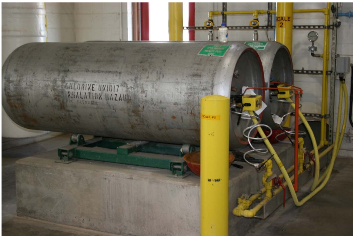
1 ton Chlorine containers. Automatic Shutoff device connected to the liquid side only. The top valve is used for the gas. Remember that containers lay on their sides and cylinders stand upright.
