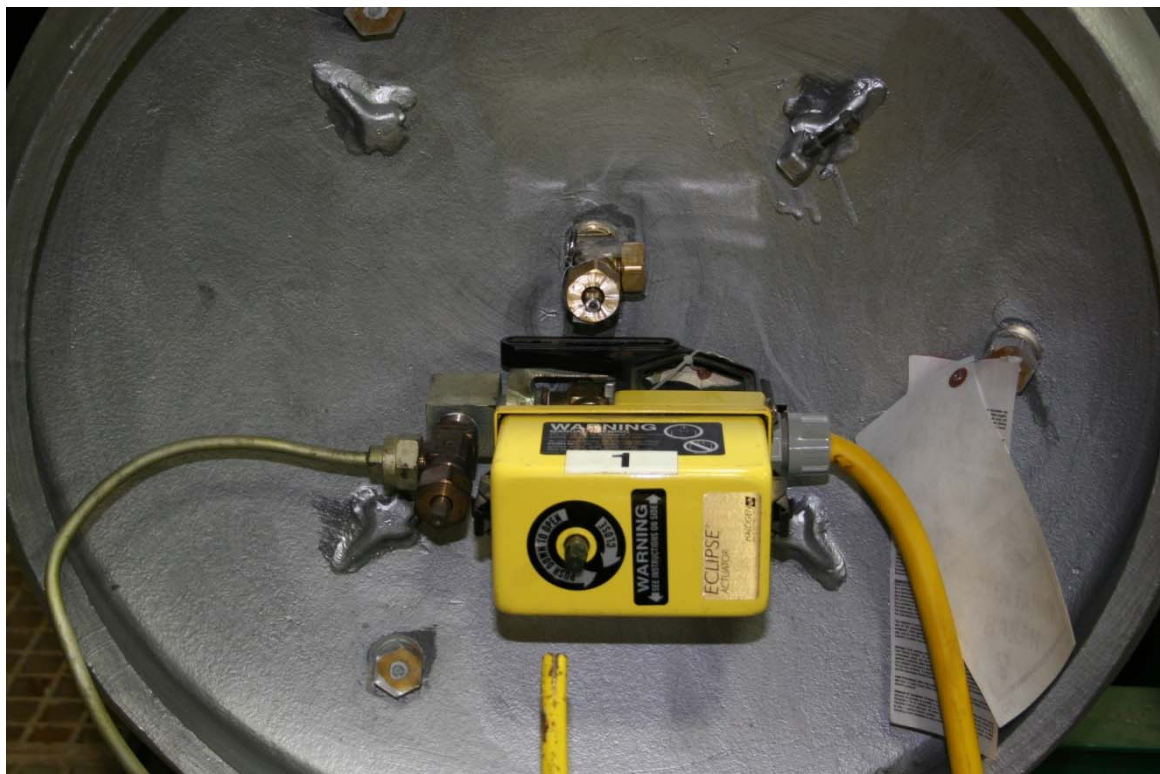
1 ton Chlorine containers. Automatic Shutoff device connected to the liquid side only. The top valve is used for the gas. Remember that containers lay on their sides and cylinders stand upright.
