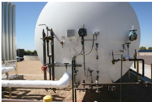
Oxygen tank is necessary to generate O_3
