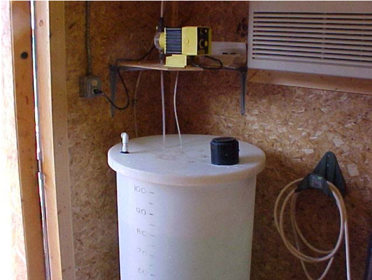
Small Chlorine solution tank.
