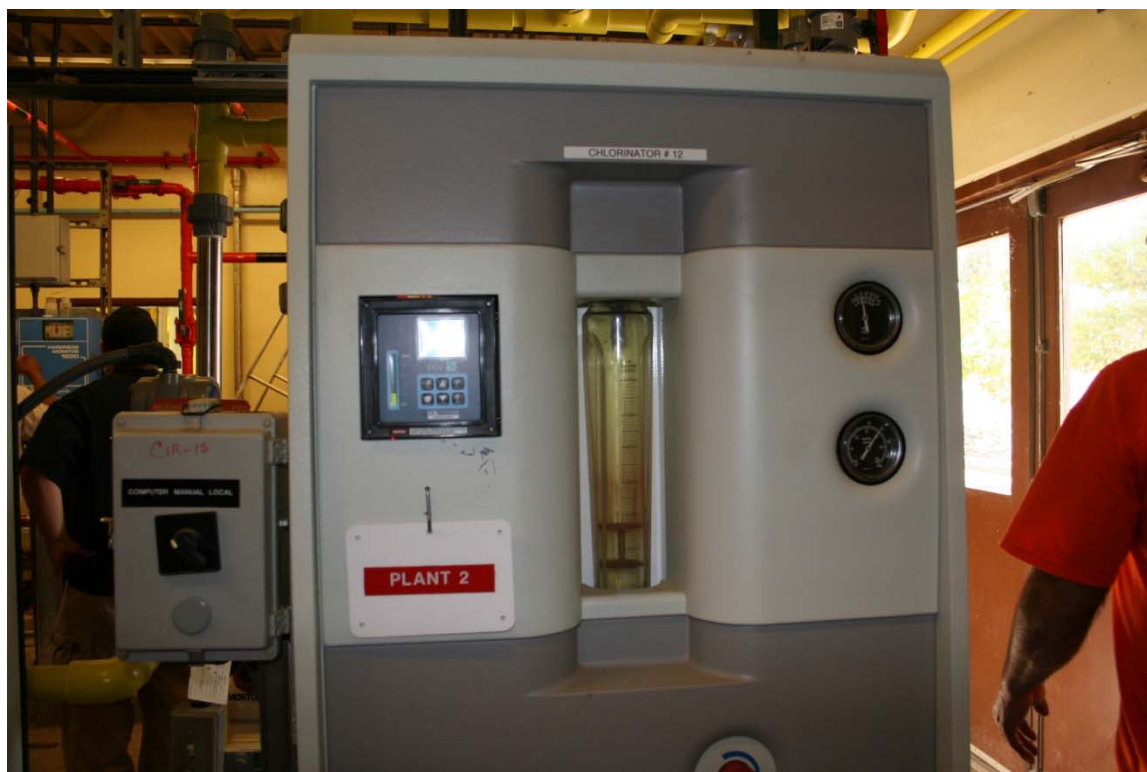
Chlorine gas rotometer
