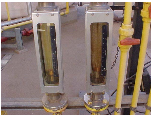
Chlorine measurement devices or Rotometers.
