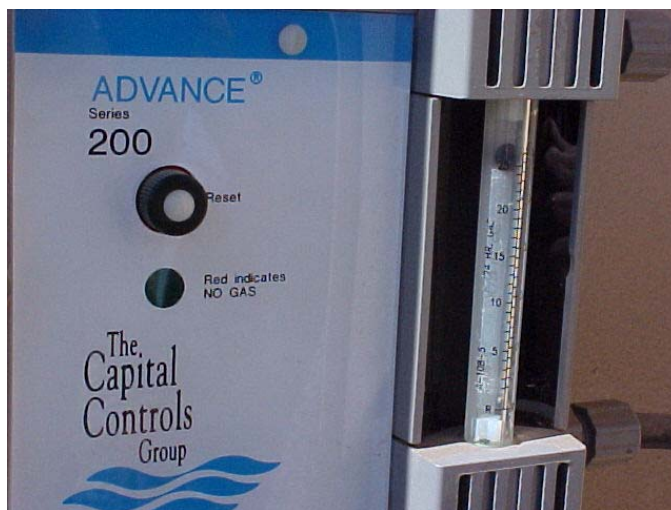
Chlorine measurement devices or Rotometers.
