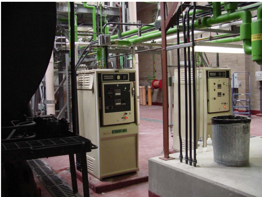
Chlorine evaporators next to a rail tank chlorine cylinder. Bottom photograph, SCBA should always be stored on the outside of the chlorine storage room.
