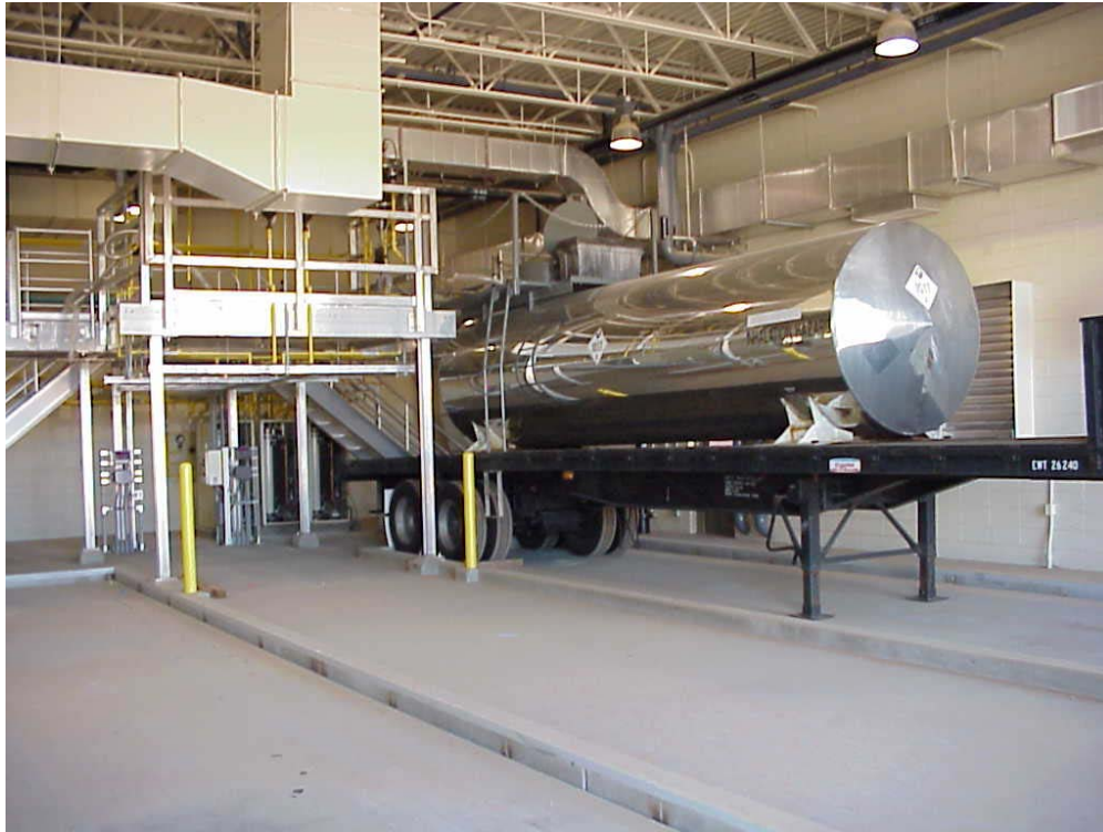
Example of a Chlorine Storage Room.
