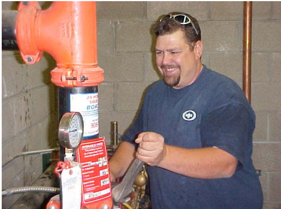
Top, a highly trained General Backflow Assembly Tester is working on a fireline assembly. Bottom, a double check backflow preventer with OS& Y valves.
