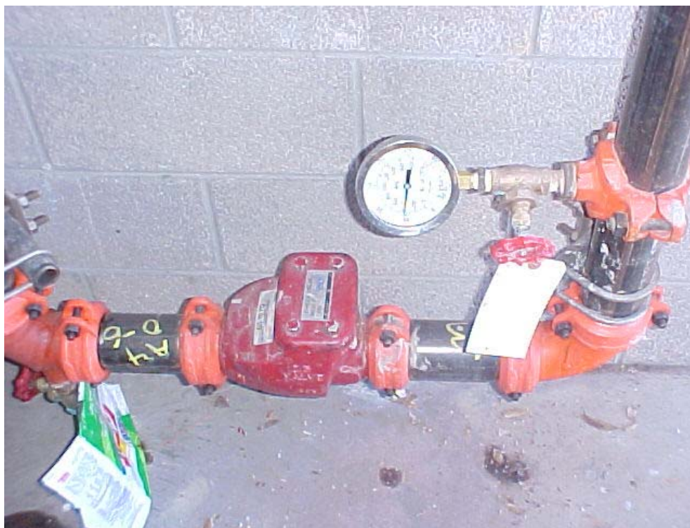
RPDA, Two Reduced Pressure Principle Backflow Assemblies together on a Fireline. Ames SS Assembly. Below an Antifreeze Loop with check valve on a Fireline. Notice the OS&Y Valves (Outside Screw and Yoke).
