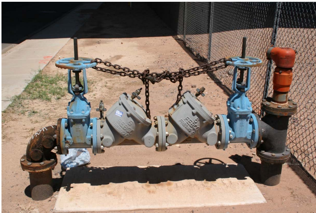
Top, a highly trained General Backflow Assembly Tester is working on a fireline assembly. Bottom, a double check backflow preventer with OS& Y valves.
