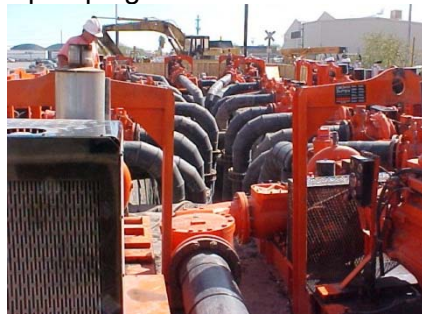
Pumps at a temporary sewer manhole by-pass.
