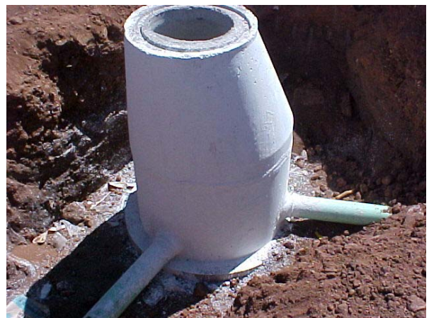
Newly finished Manhole and Laterals.
