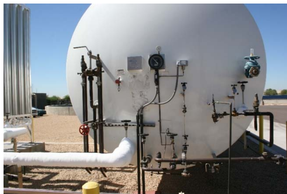
Oxygen tank is necessary to generate O_3
