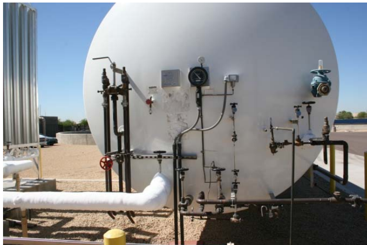
Oxygen tank is necessary to generate O_3
