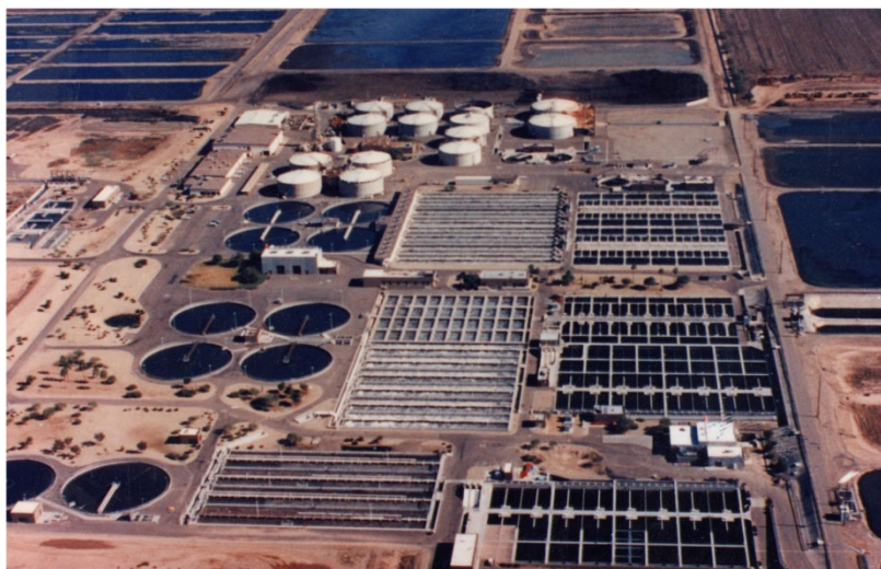
Modern wastewater treatment plant.
