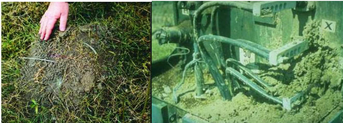
Fire ant mound; right side is Fire ant damage to an electrical transformer.
