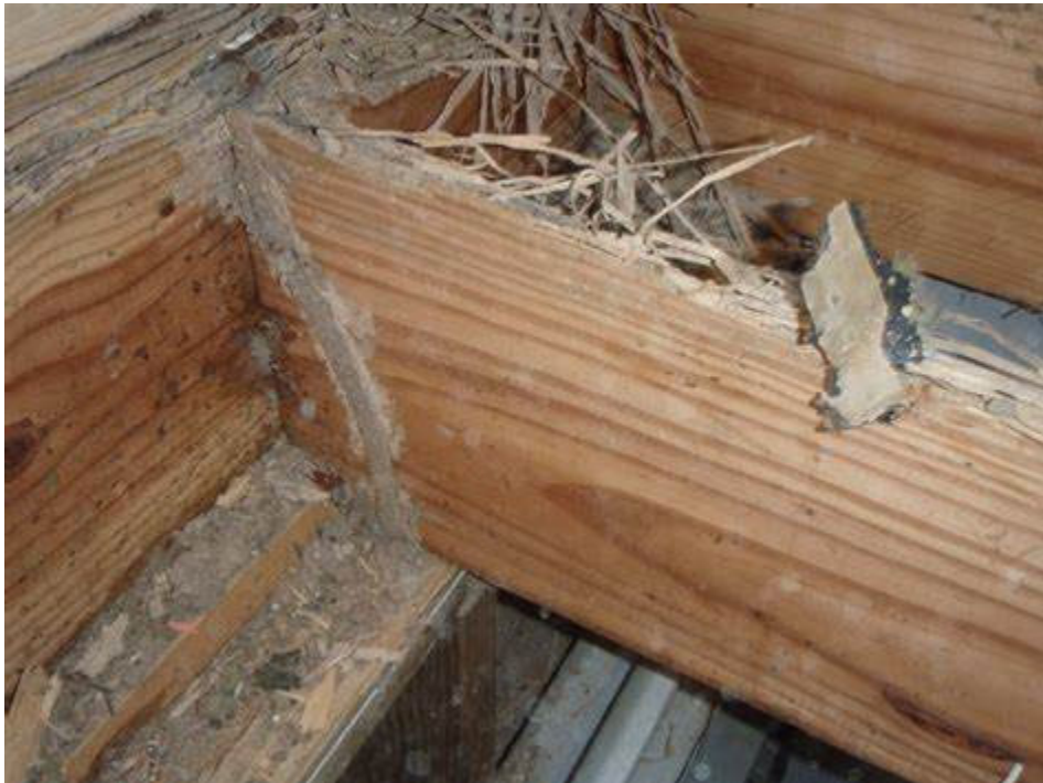
FORMOSOAN MUD TUB AND DAMAGE EXAMPLE
