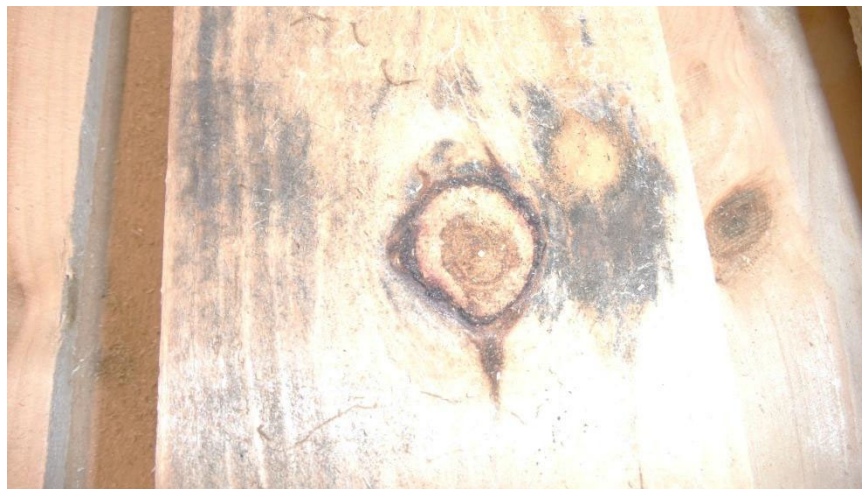
WOOD MOLD ON PROCESSED LUMBER MOLDS AND STAINS COME IN MANY DIFFERENT COLORS THIS ONE ABOVE IS WHITE
