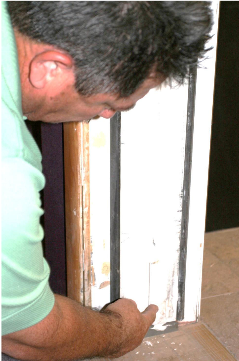
Probing interior trim wood reveals termite damage.
