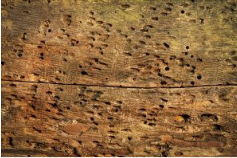
POWERPOST BEETLE DAMAGE
