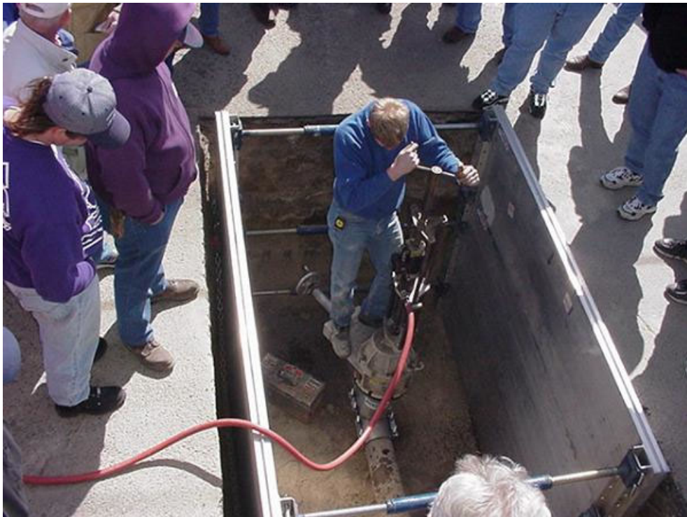
Hydro Stop valve insertion machine
