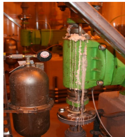
These photographs show an Alum leak. When exposed to air, this chemical becomes crystallized.
