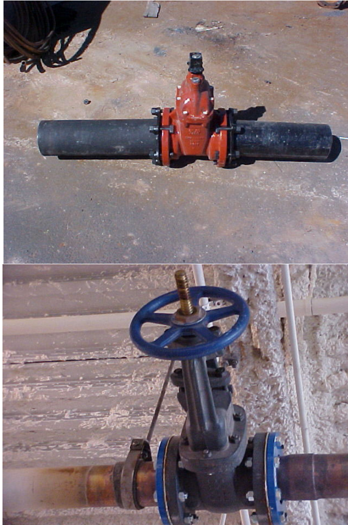
Different types of Gate Valves. (Linear)
