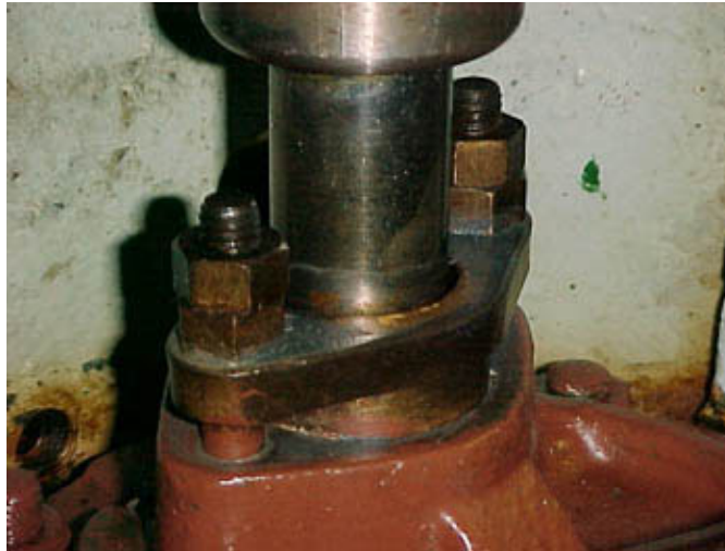
PUMP PACKING BOX WITH ADJUSTMENT LOCK NUTS
