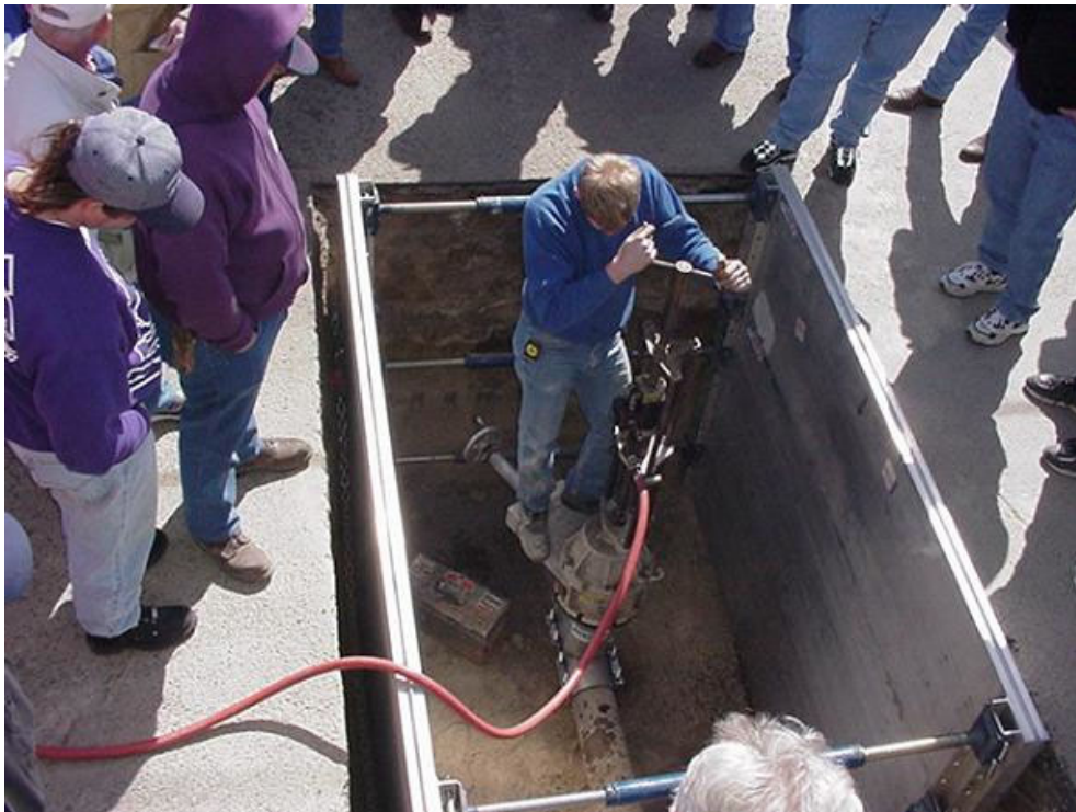
Hydro Stop valve insertion machine
