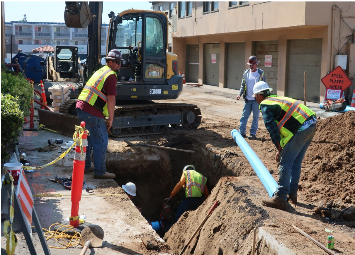
Replacing a section of plastic water main
