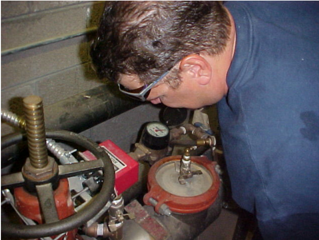
A Certified Backflow Tester (Jerry Durbin) examining a Double Check Detector check fire line assembly.
