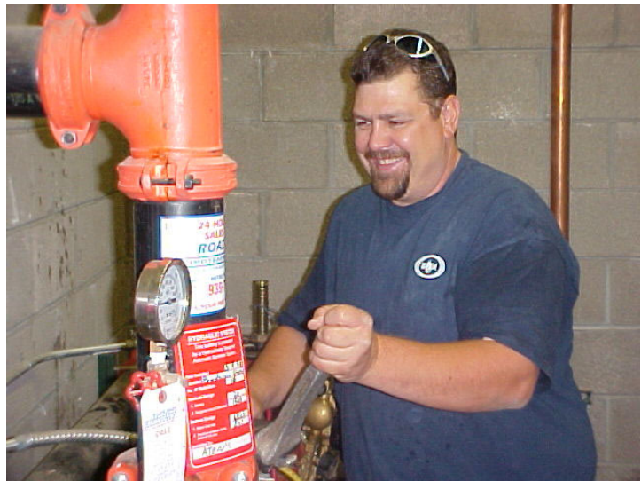
A Certified Backflow Tester (Jerry Durbin) examining a Double Check Detector check fire line assembly.
