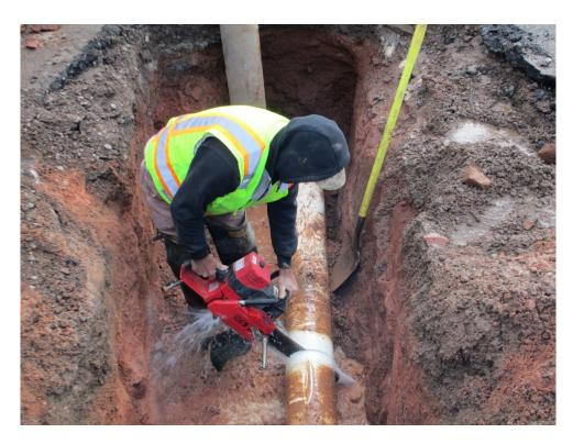
Any work with a chainsaw or powersaw should include proper safety equipment including proper eye protection, face shield, and hearing protection. The blue pipe is an eight-inch plastic C900 and will be utilized for the repair.
