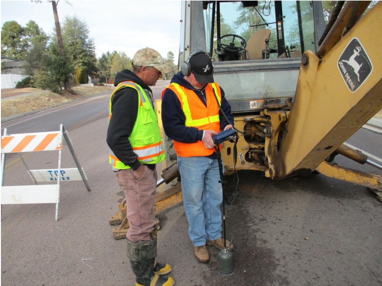
In this photograph, we see two men checking the results of a hydrophone. In areas of thick blacktop, it is difficult to locate small service leaks and slow water main breaks. A hydrophone is a microphone designed to be used underwater for recording or listening to underwater sound. Most hydrophones are based on a piezoelectric transducer that generates electricity when subjected to a pressure change.
