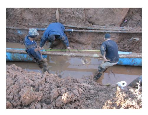
Ensure policies and procedures will be followed when excavating across foreign utilities and other underground structures. Ensure that the competent person *is available* while any trenching/excavation work is being performed. Ensure that benching, sloping, and shoring practices are followed when necessary. Ensure proper protection and support of existing utilities and structures.
