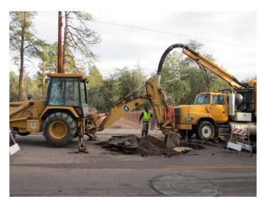
In this case, a sewer vactor was utilized to expedite removal of water and spoil. Utilizing a vactor is a great tool, but is dangerous. It is easy to lose tools and injure personnel if the vactor is not properly managed. The vactor is powerful enough to lift large stones and even a 200-pound man.
