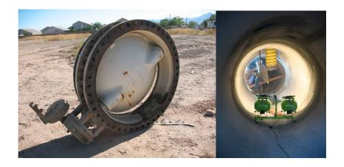
A broken 54-inch Butterfly and a worker inside the water main preparing the interior surface. Notice, this is a Permit Required Confined Space. Hot work permit is also required. Side note, there is a plastic version of the 54 and 60-inch butterfly valve.
