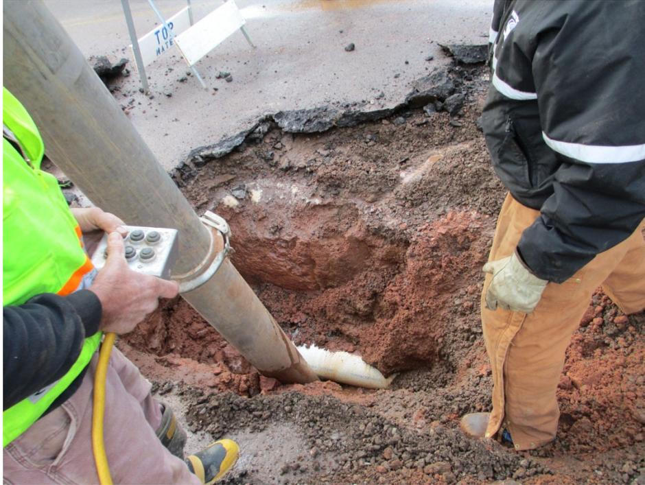
In this photograph, a plastic water main is discovered; there is a red wire under the main for bluestaking purposes. The hair-line crack is about a foot long, so it will be necessary to cut out about 4 feet to make sure the water main will not leak in the future.
