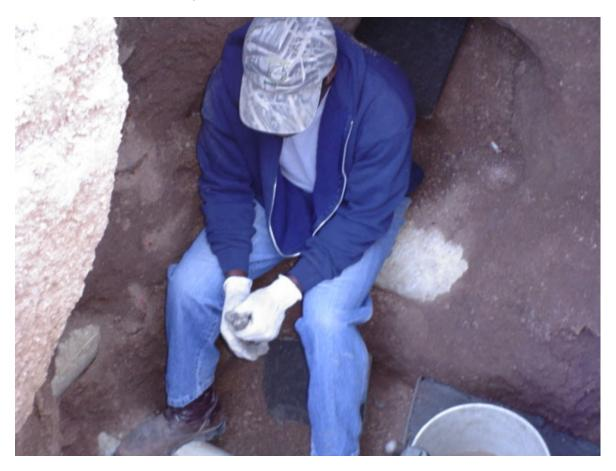
This poor soul is probably going to be a short timer here on earth. He is sitting on the sewer main in a bell shaped hole under a steel plate which cars are driving over. No protection at all. There was a ladder in the trench but was about 50 feet away.
