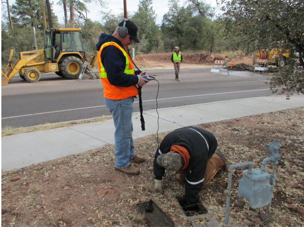
These men are listening to a stop to find a difficult leak. Some hydrophones magnify the sound and others use a meter to locate the leak. Many old-timers use a short piece of copper tubing and have good results.
