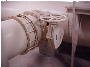
Thermal insulation of the valve body is recommended for operating temperatures above 392°F (200°C). The valve should be installed in the closed position to ensure that the laminated seal in the disc is not damaged during installation.
