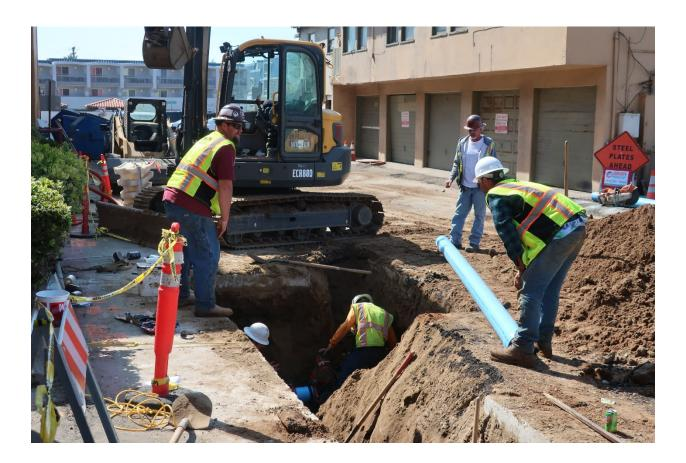
The distribution system must protect water quality between the source and the customer's tap. Proper construction/repair is important in maintaining system integrity. Care must be taken that no foreign material is introduced into the system during repair or pipe laying operations.
