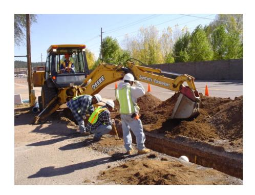
Two unsafe excavation examples: Top, notice the man in a 6-foot-deep trench with no ladder or shoring, and the placement of spoil. Bottom photograph, utilities are marked after the excavation has begun, no hard hats, no ladders, no protective system, incorrect spoil placement.
