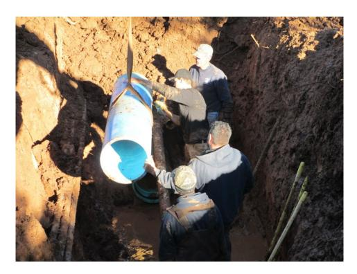
Wear appropriate personal protective equipment (PPE) as required for the task being performed and as required per OSHA regulations. Ensure a spotter is used if there are overhead power lines, underground utilities or tight working conditions in the work area. Verify the competent person is on site and that records are kept of all work and safety procedures.
