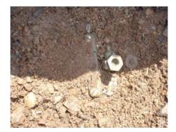
Another buried RP assembly deep inside a vault, all we can see is a test cock. All RPs need to be installed 12 inched above the ground. This device was buried in ground and not tested for over 25 years. Owners are required to test their devices once a year at a minimum.
