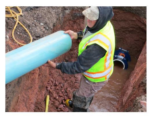
You will notice the blue Hymax coupling is being utilized instead of a clamp or flex coupling. This coupling is easy to use and has only two bolts and a special two-part gasket for odd size pipe.
