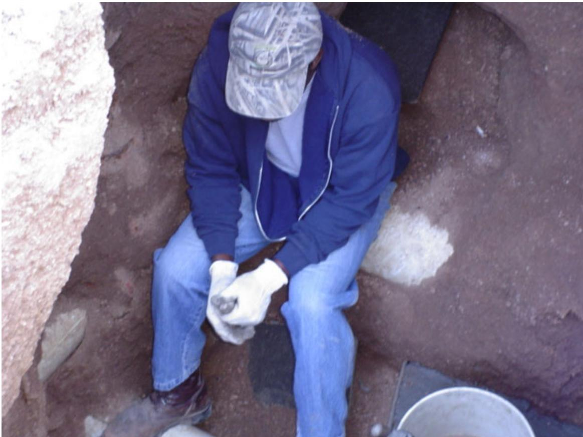
This poor soul is probably going to be a short timer here on earth. He is sitting on the sewer main in a bell shaped hole under a steel plate which cars are driving over. No protection at all. There was a ladder in the trench but was about 50 feet away.
