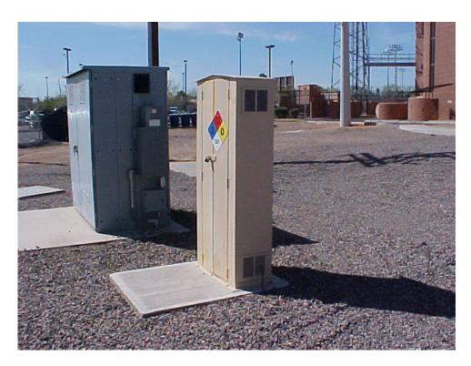
Small chlorine storage shed in the foreground; notice the vents at the bottom and top. The bottom vent will allow the gas to ventilate because  $Cl_2$  gas is heavier than air.
