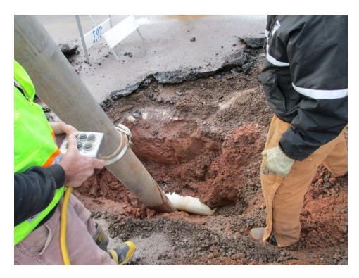
In this photograph, a plastic water main is discovered; there is a red wire under the main for bluestaking purposes. The hair-line crack is about a foot long, so it will be necessary to cut out about 4 feet to make sure the water main will not leak in the future.
