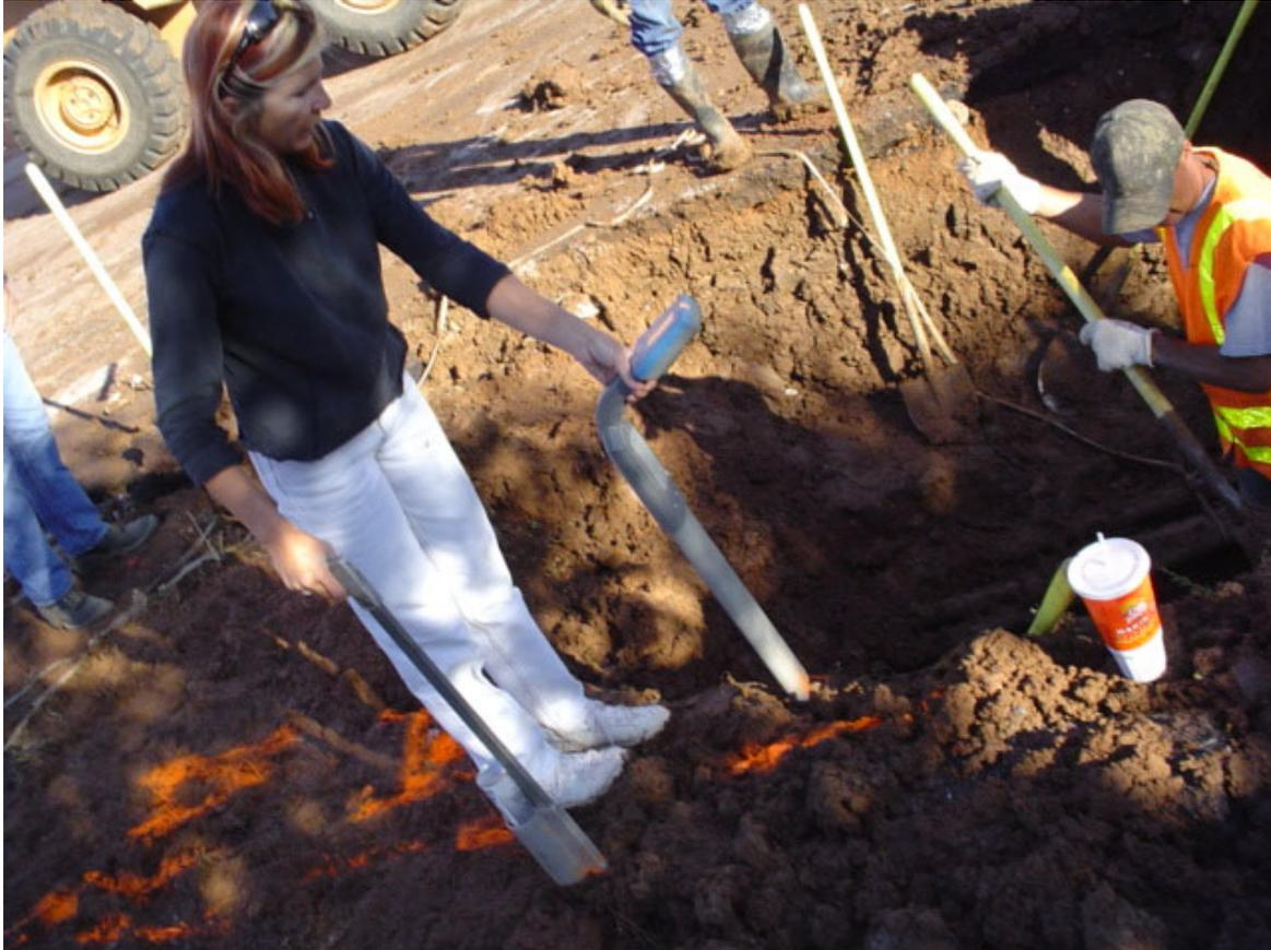
Always wait for the buried utilities to be marked before excavation begins. Unbelievably, this service repair crew dug 9 feet deep before the Locator showed up and marked fiber optics in the same trench. Notice that the employees do not have hard hats, ladders, or any protective systems. Several major OSHA violations.
