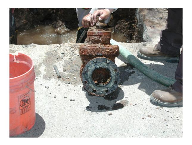
Here is a 4-inch broken gate valve with serious tuberculation. The valve is broken in the closed position. The rust particles are sharp and can easily cut the water service worker.
