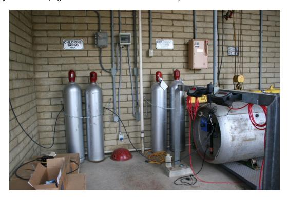
In the photo, we have a 1-ton chlorine gas container and 150-pound Cl<sub>2</sub> gas cylinders. The 1- ton is on a scale. Cylinders stand up-right and containers on their sides.
