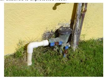
This PVB is not 12 inches above the ground nor the highest downstream outlet.
