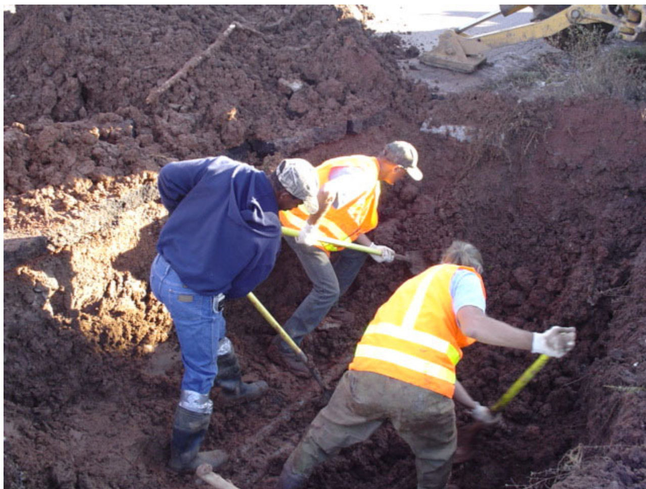
A water distribution crew repairing a hidden leak.
