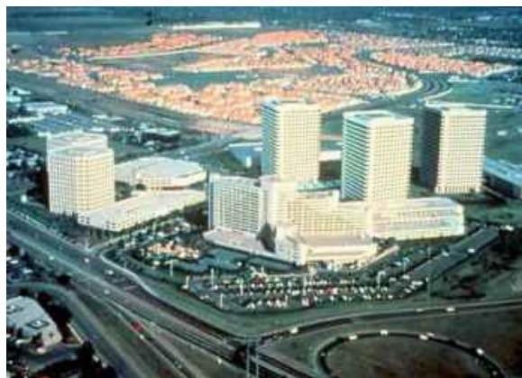
The Irvine Ranch Water District provides recycled water for toilet flushing in high rise buildings in Irvine, California. For buildings over seven stories, the additional cost of providing a dual system added only 9% to the cost of plumbing.
