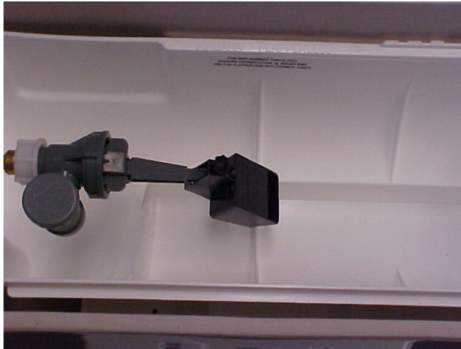
Inside the tank of the Flapperless Low-Use Toilet made by Niagara.
